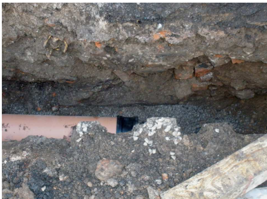
Plate 4: Fragmentary remains of a brick wall exposed in the excavated service trench
