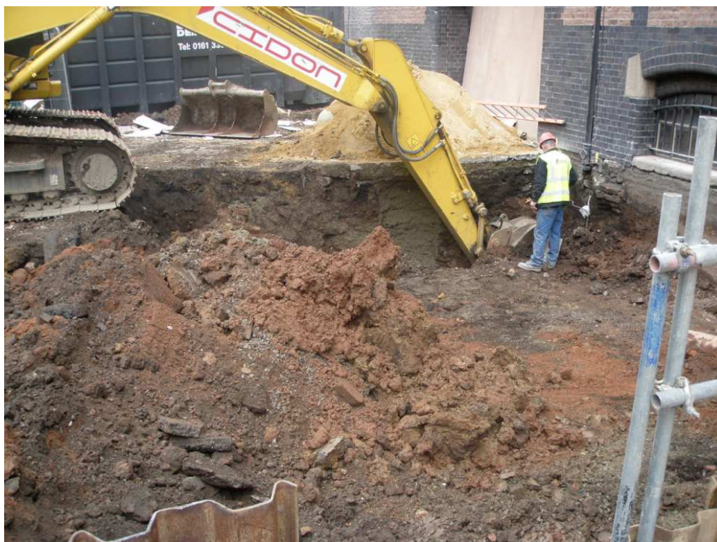
Plate 6: Excavating the western lift shaft
