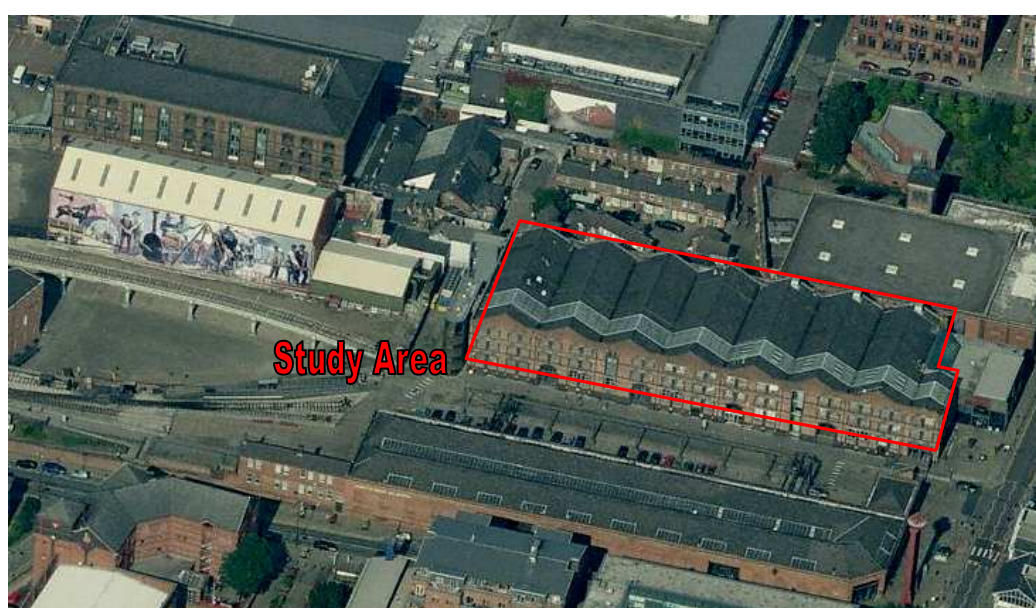
Plate 1: Aerial view of Lower Byrom Street Warehouse
