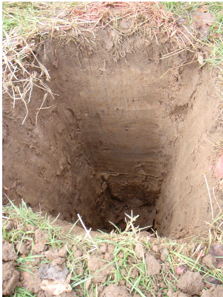
Plate 2: Inspection pit for BH8
