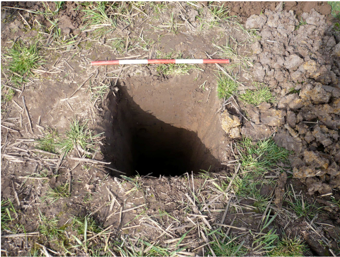
Plate 1: Inspection pit for BH4
