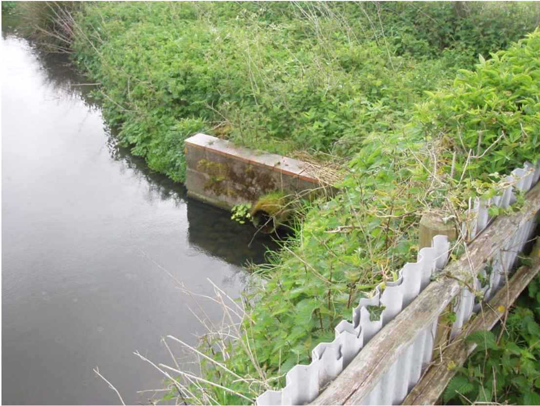
Plate 3: Site 11 , drainage pipe discharging into pond
