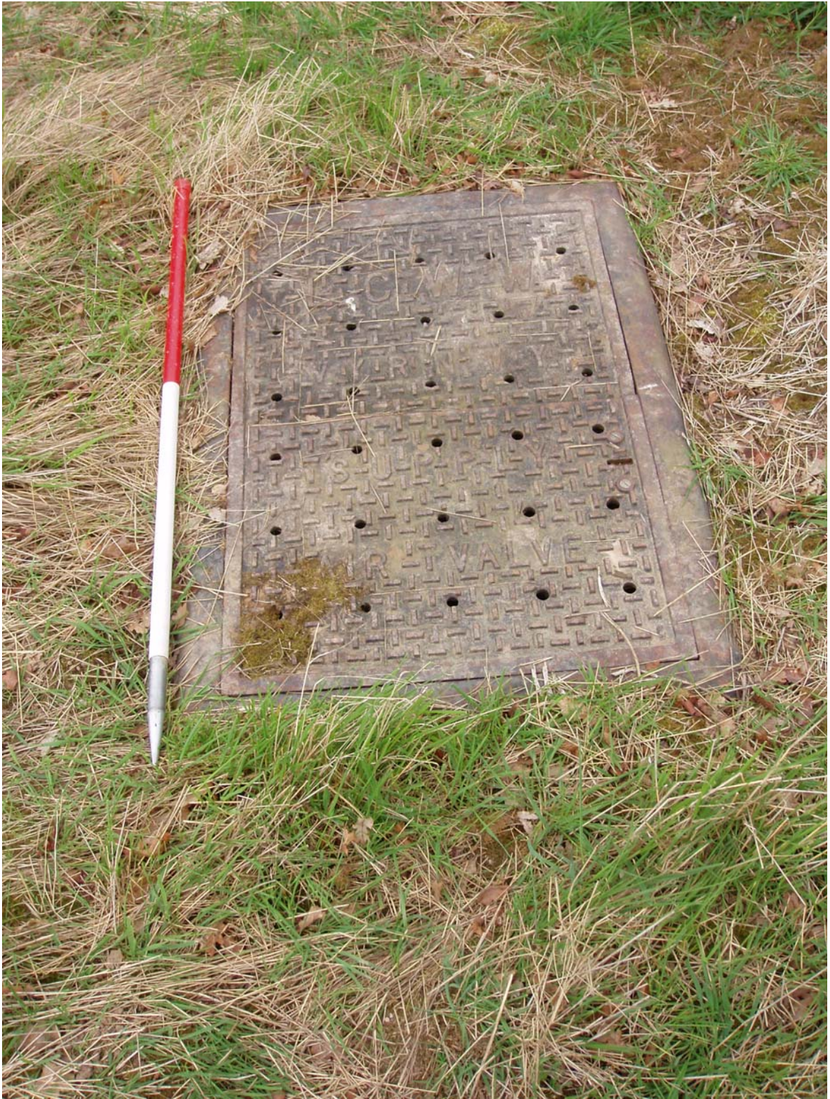
Plate 5: Site 13 , metal inspection cover marked L.C.W.W. and Vyrnwy, of the same style as those at sites 14 and 15 .
