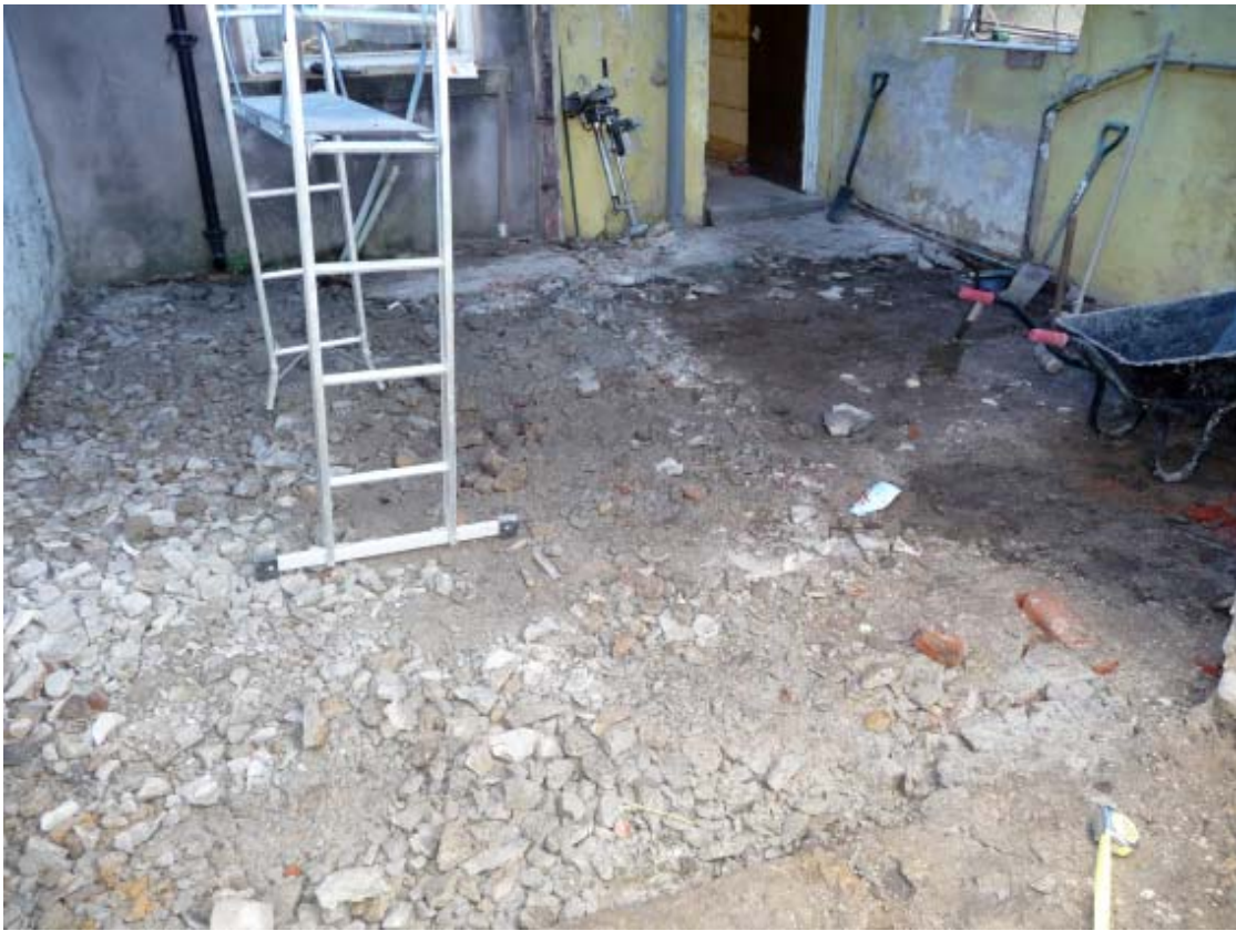
Plate 1: Area of excavation, prior to work
