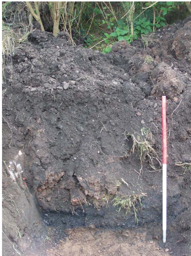
Plate 4: Section through the Carlisle to Silloth railway embankment (Site 15)
