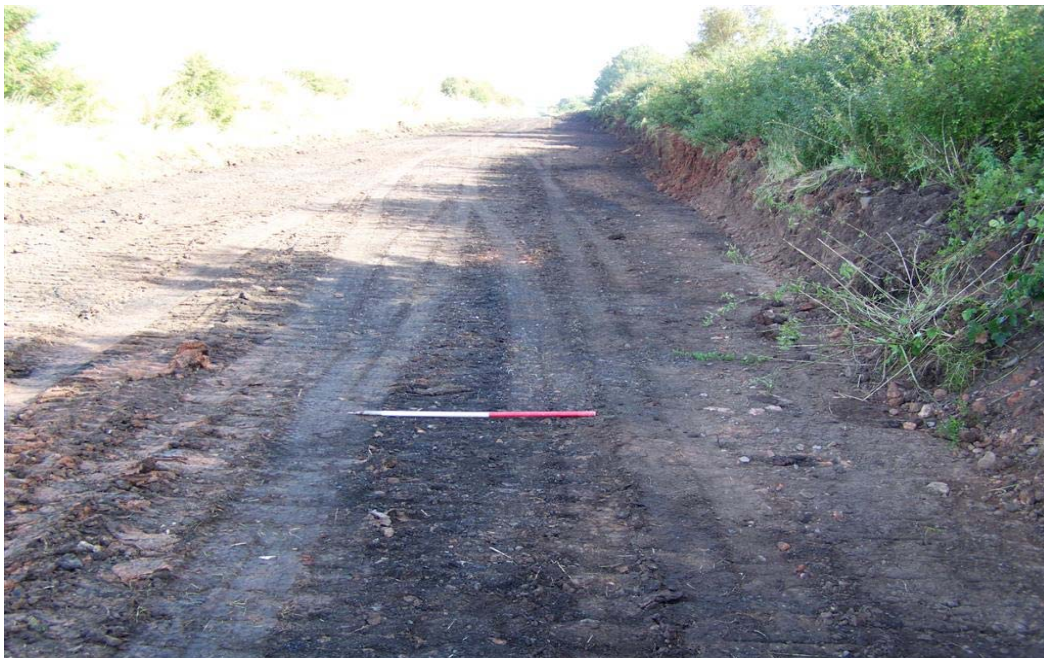
Plate 2: Stripped easement in Field 2
