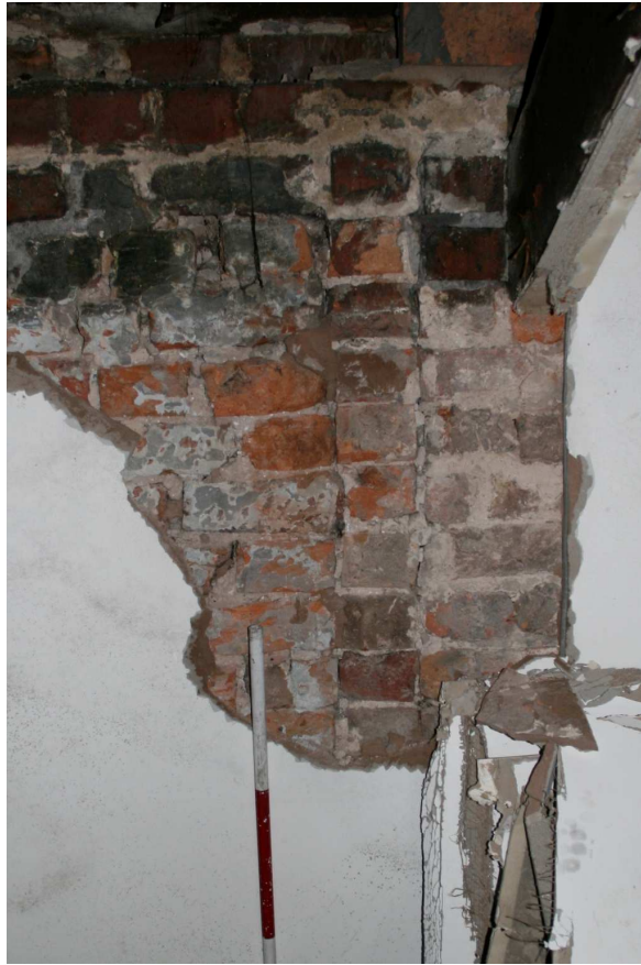
Plate 7: Scar of original single-skin dividing wall between 89 and 91 Great Ancoats Street, exposed on the second floor
