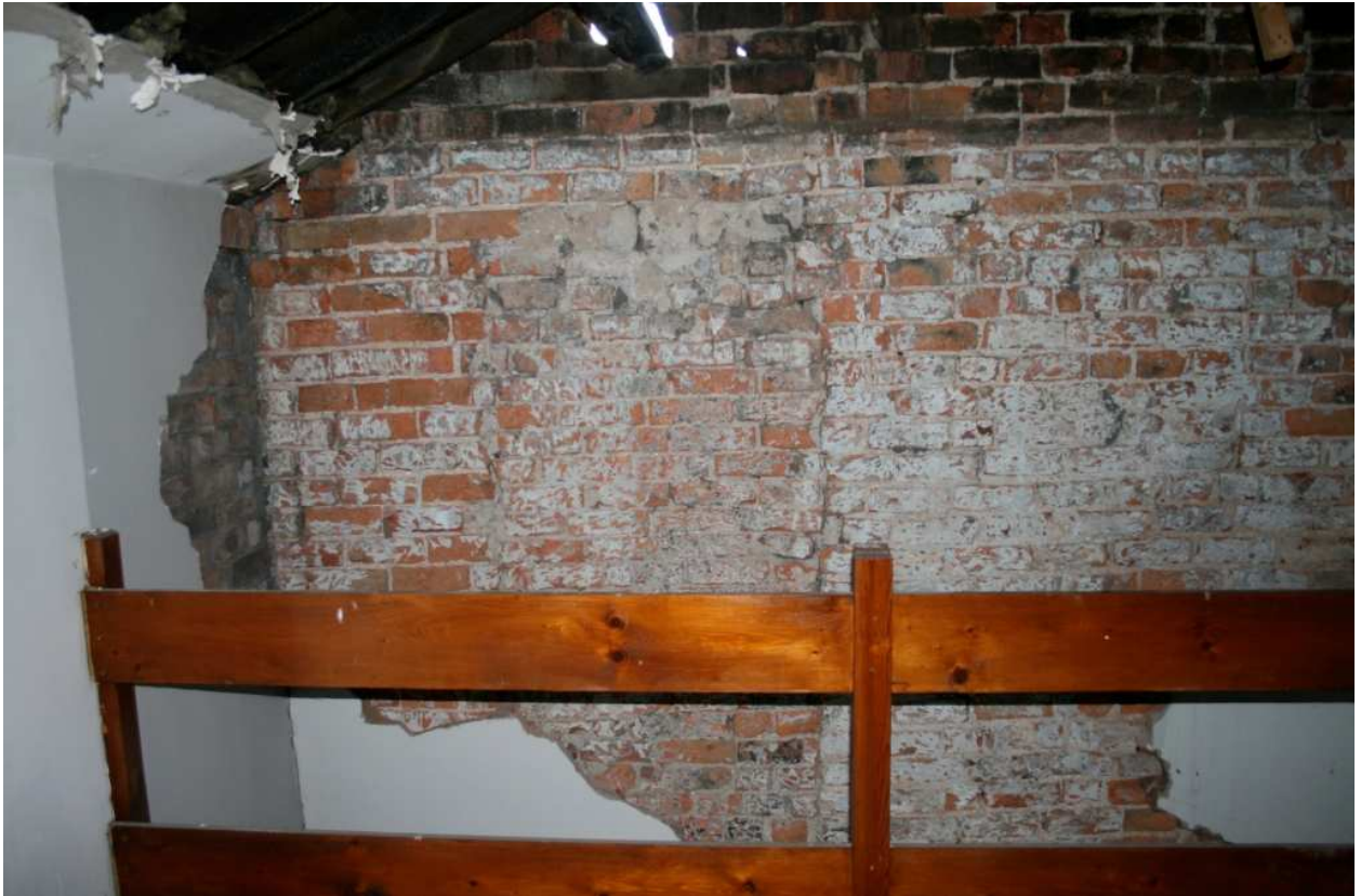
Plate 9: Blocked doorway on the second floor of 89 Great Ancoats Street
