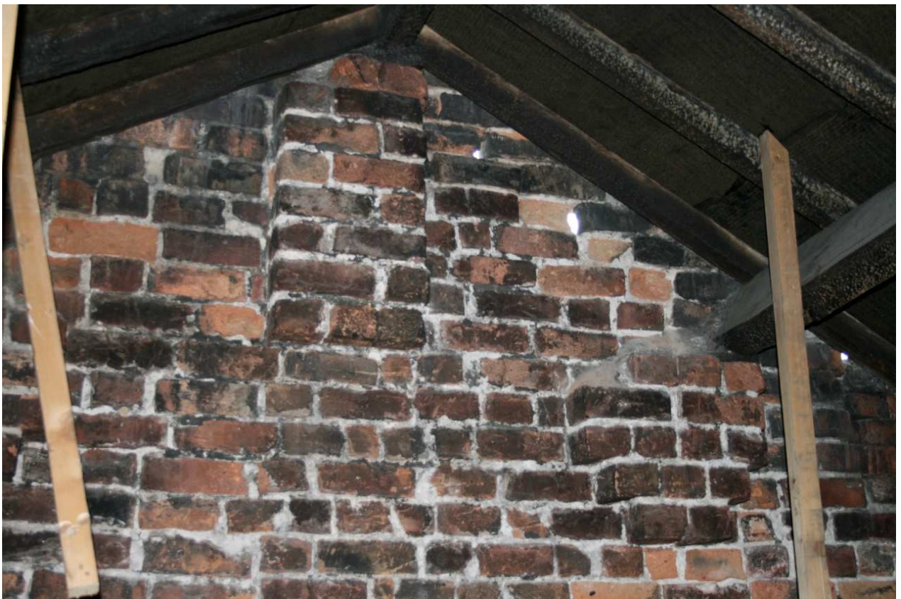
Plate 10: Tiered brick corbels on the second floor of 89 Great Ancoats Street
