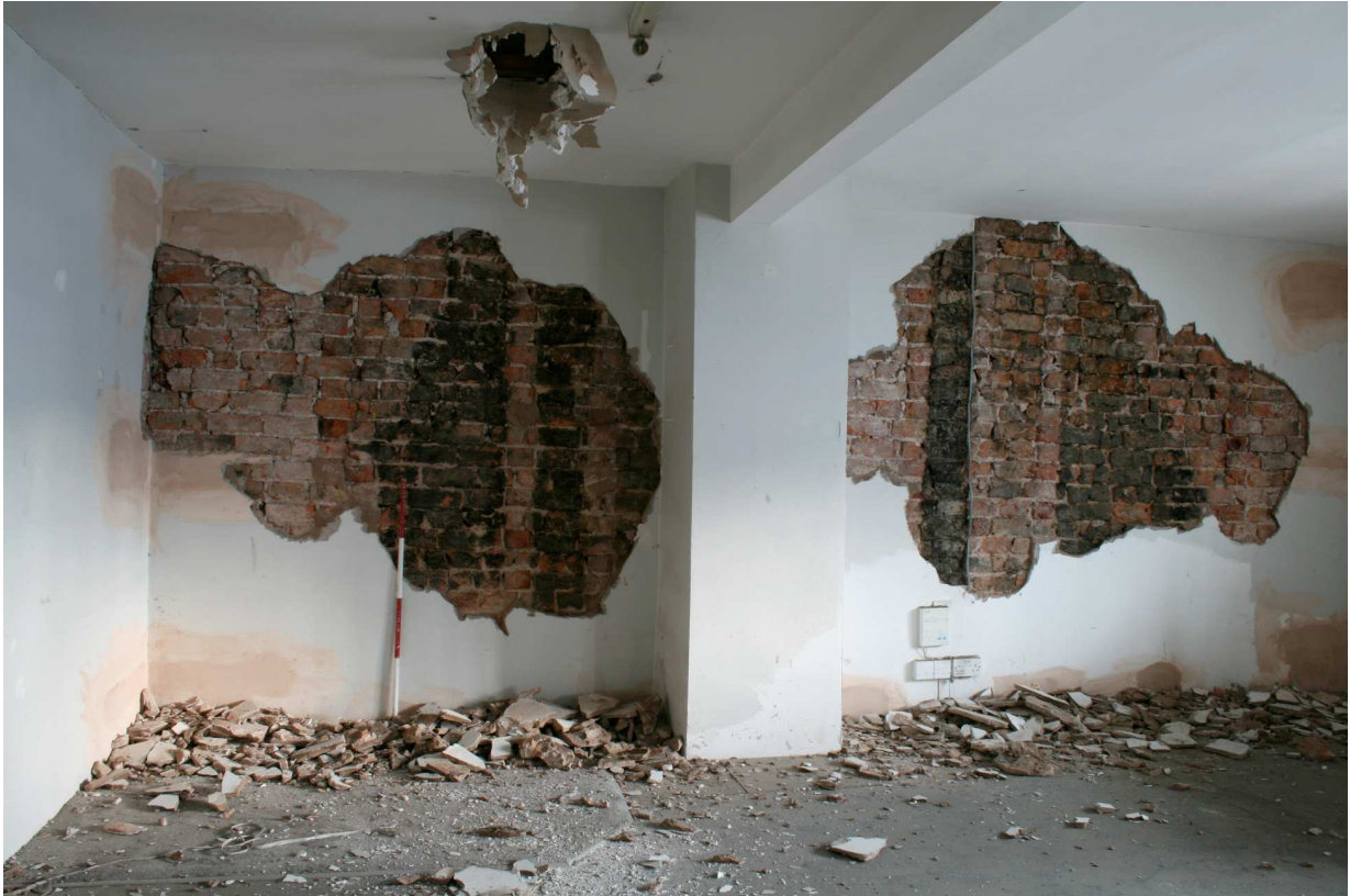
Plate 5: Scars of two fireplaces surviving on the south-east elevation of the first floor of 91 Great Ancoats Street
