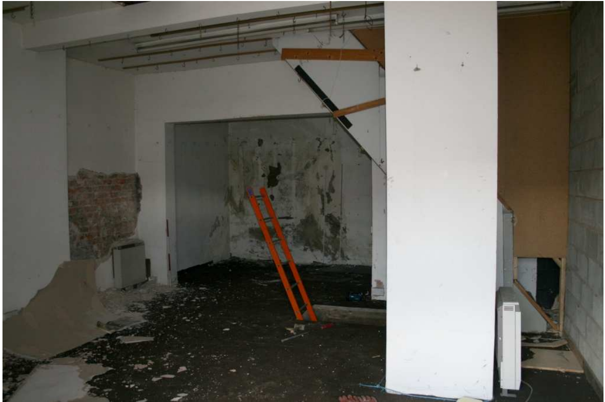
Plate 3: Ground floor, 89 Great Ancoats Street
