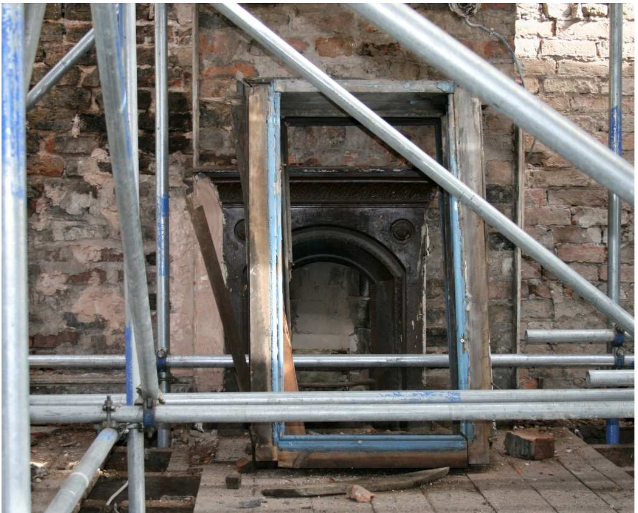
Plate 12: In-situ fireplace on the first floor of 87 Great Ancoats Street
