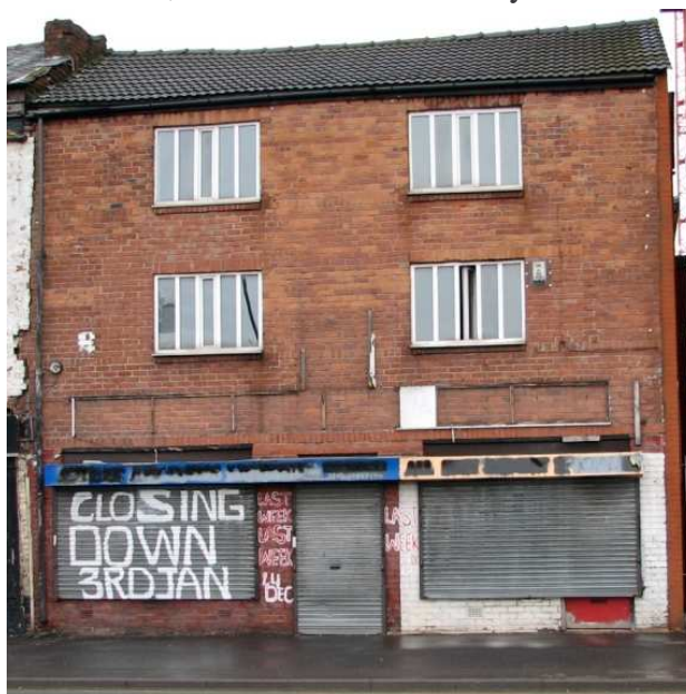
The front elevation of 89-91 Great Ancoats Street
