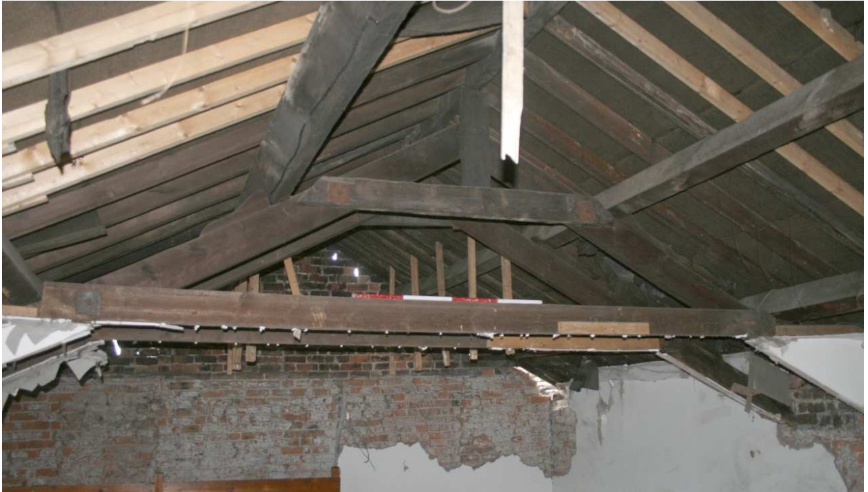
Plate 11: Truss detail with decorative cleats, 89 Great Ancoats Street
