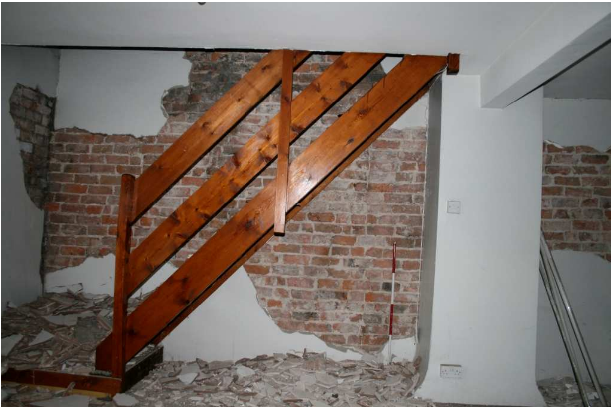
Plate 6: Butt joint behind the modern stairs on the first floor of 89 Great Ancoats Street
