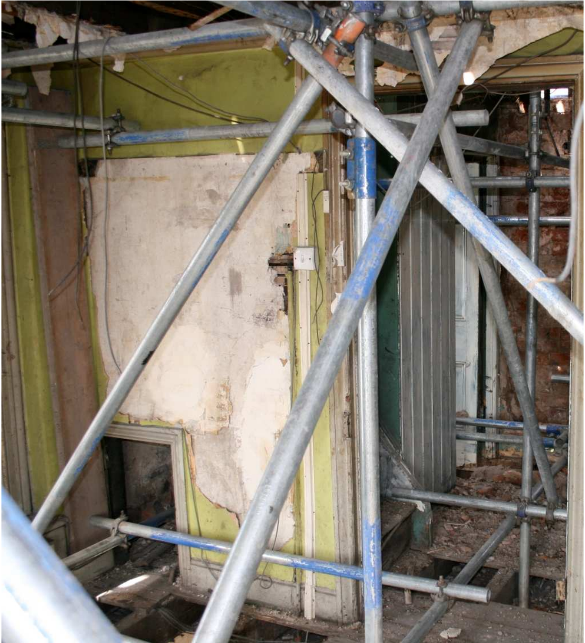
Plate 13: In-situ stair ladder on the first floor of 87 Great Ancoats Street
