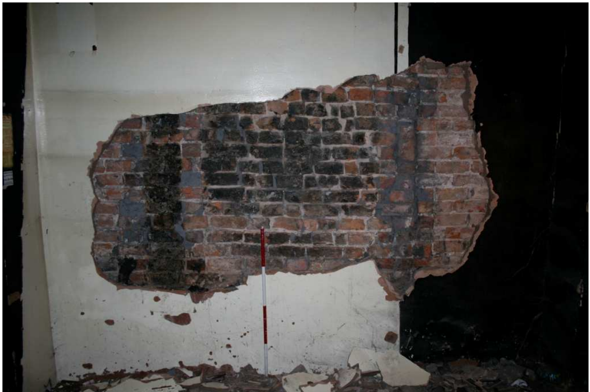
Plate 4: Fireplace scar on the south-eastern wall of the ground floor of 91 Great Ancoats Street
