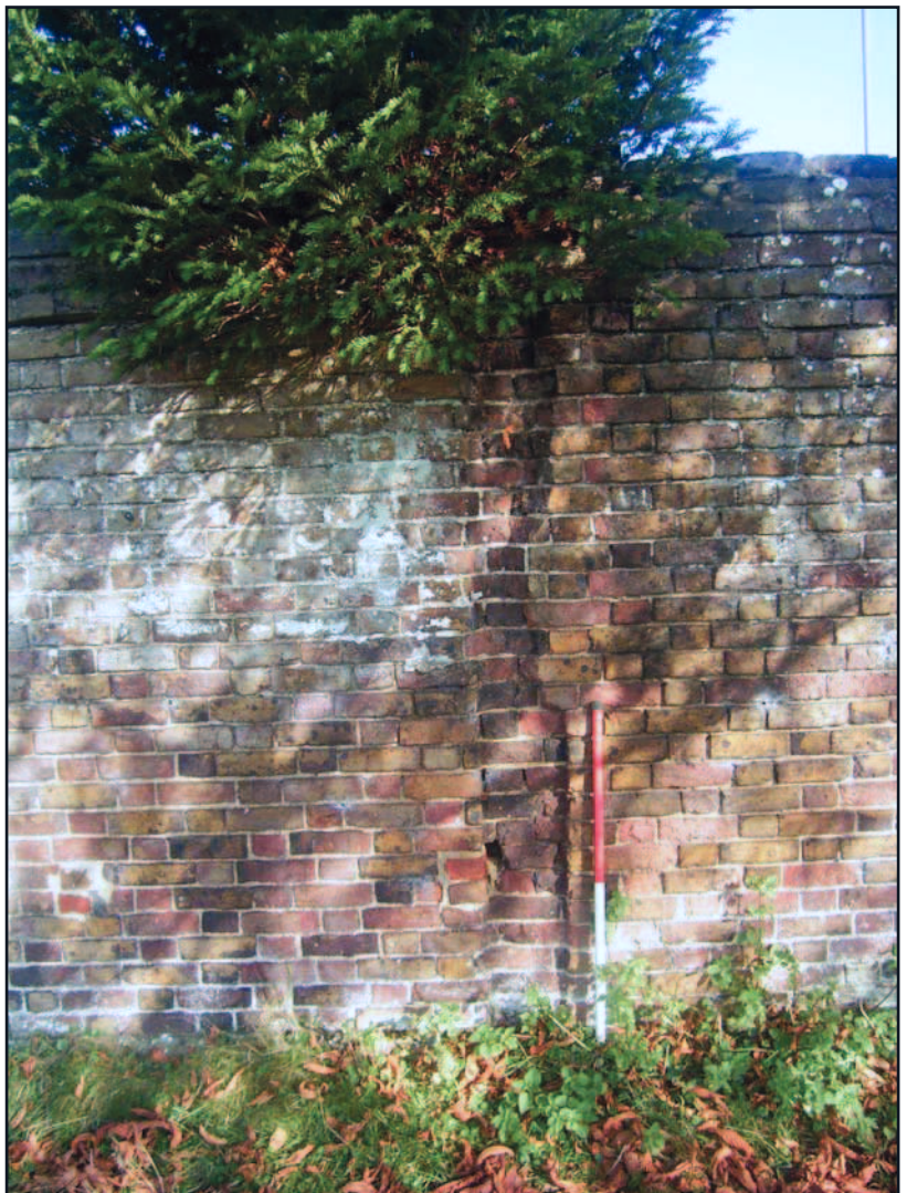
Plate 6 : Scar from later inserted wall (south face)
