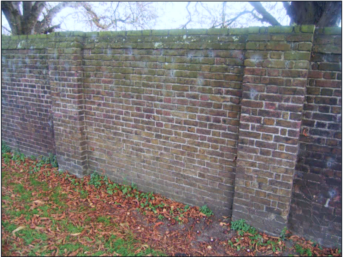
Plate 7 : Buttresses on the north face
