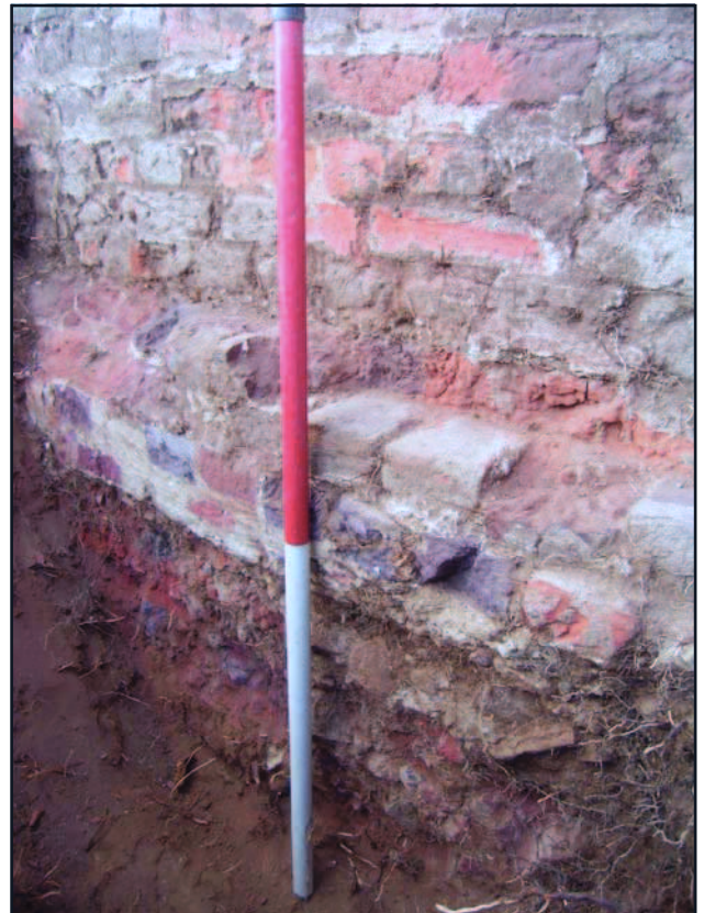
Plate 9 : Foundations in Trench 2
