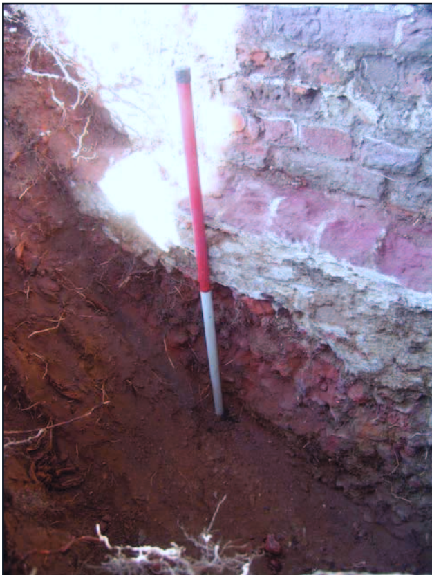
Plate 8 : Foundations in Trench 1
