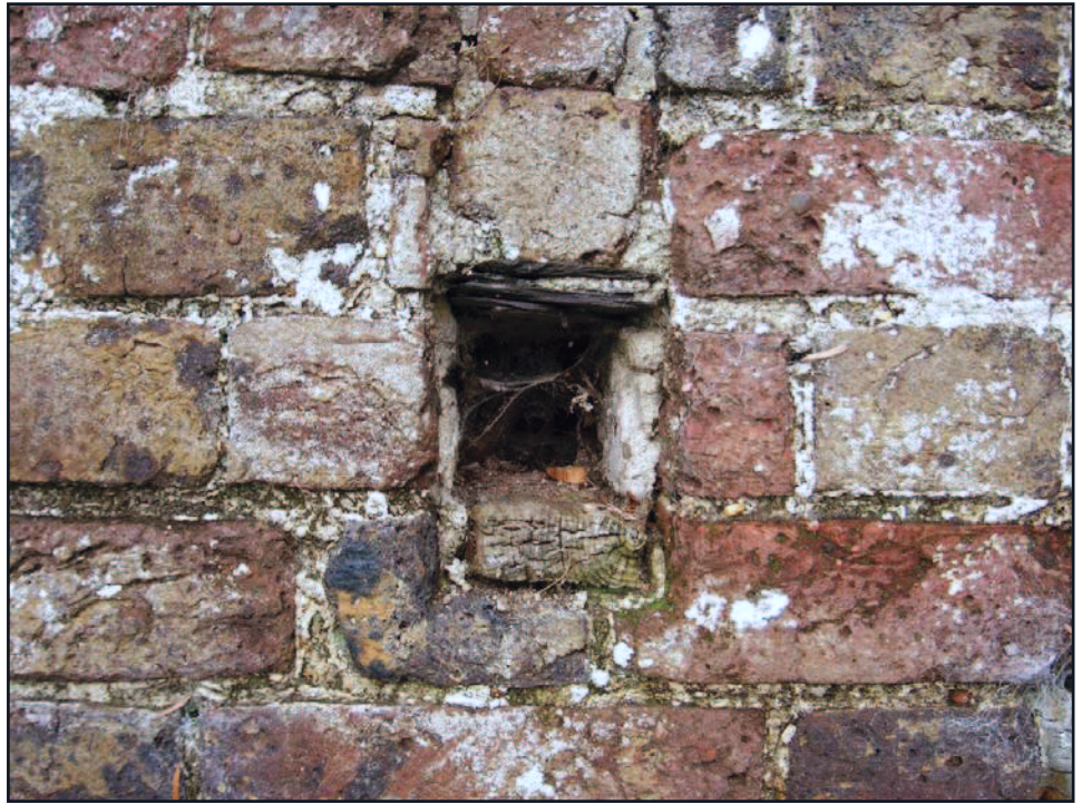
Plate 5 : Later inserted hole (south face).
