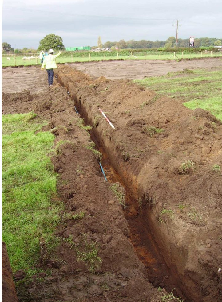
Plate 3: View along service trench, looking north-west
