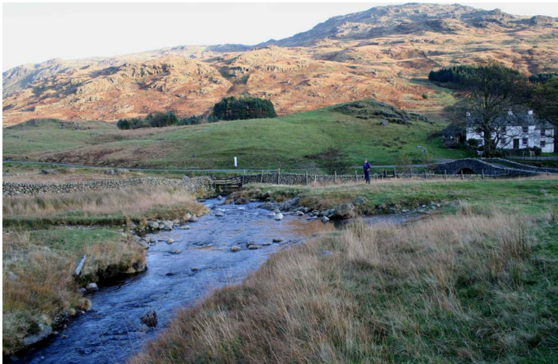
Plate 2: Three successive routes; the modern ford in the foreground, the low agger mound bridging point in the centre, and Cockley Beck bridge, carrying the modern road, in the background (photo position 40)
