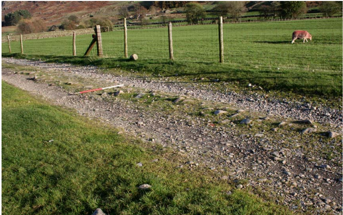
Plate 24: Section of road in moderate repair, with cobbles standing proud in the centre of the track (photo position 20)
