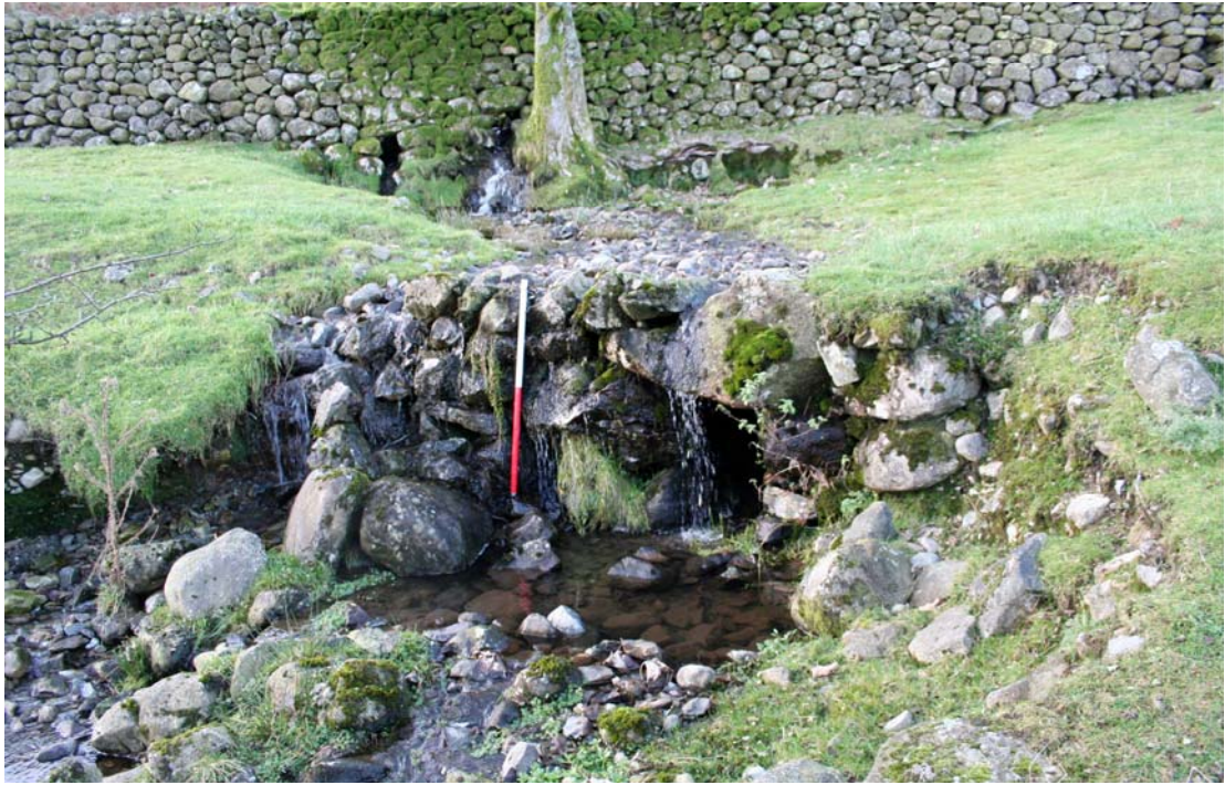
Plate 37: The substantial ford retaining wall at Roundley Beck (photo position 33a)
