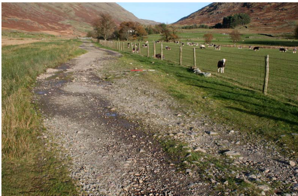
Plate 22: A wide view showing the gradual shifting of the line of the modern track and the exposed cobbles in the centre of the picture (photo position 18)
