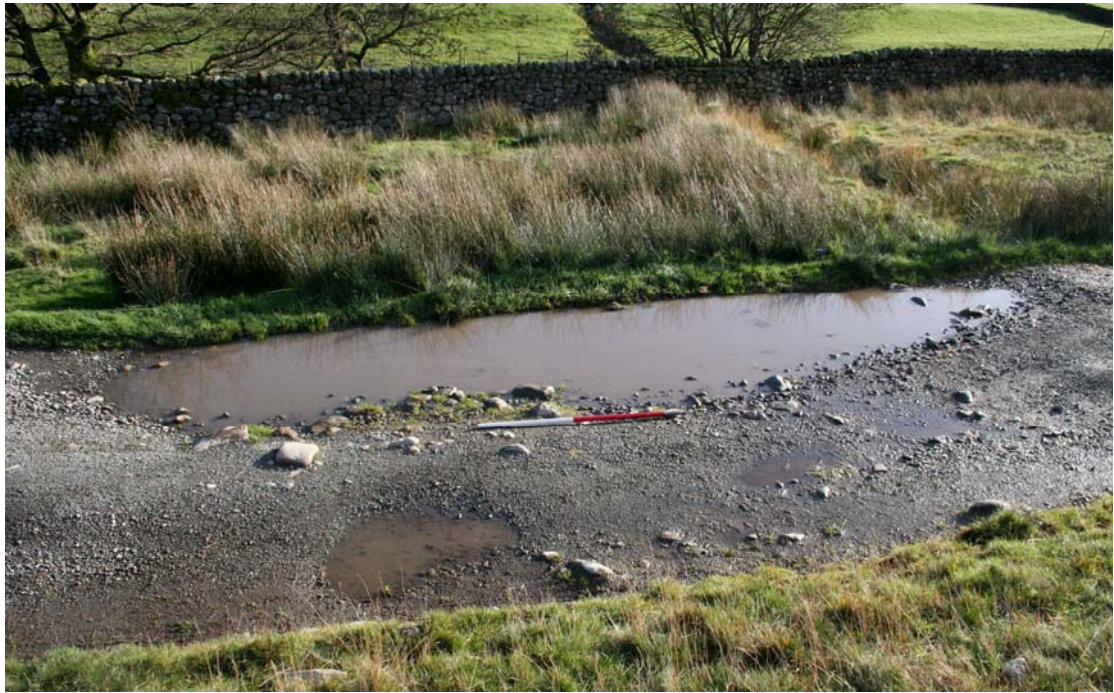
Plate 9: Area of large erosion scar (photo position 5)
