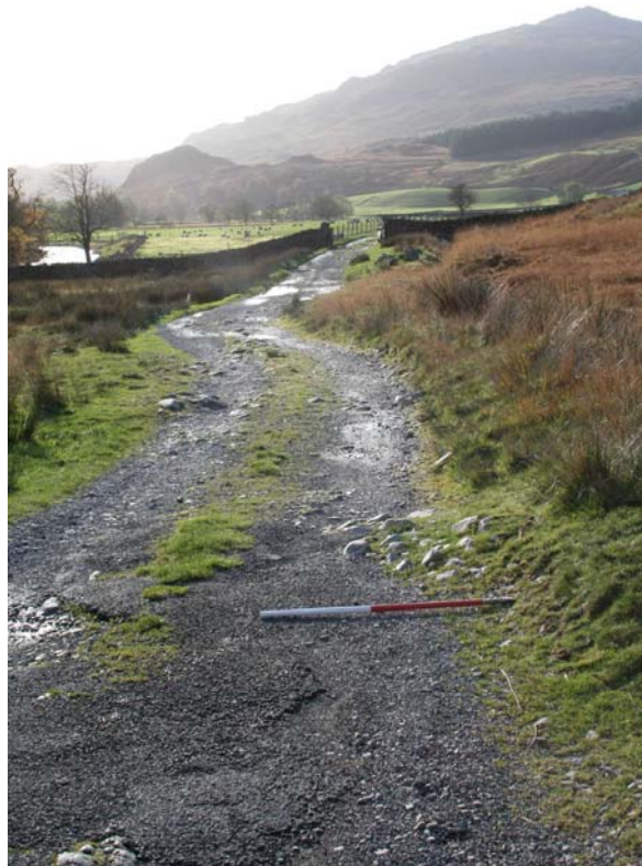
Plate 5: view of road surface looking south-west (photo position 1)
