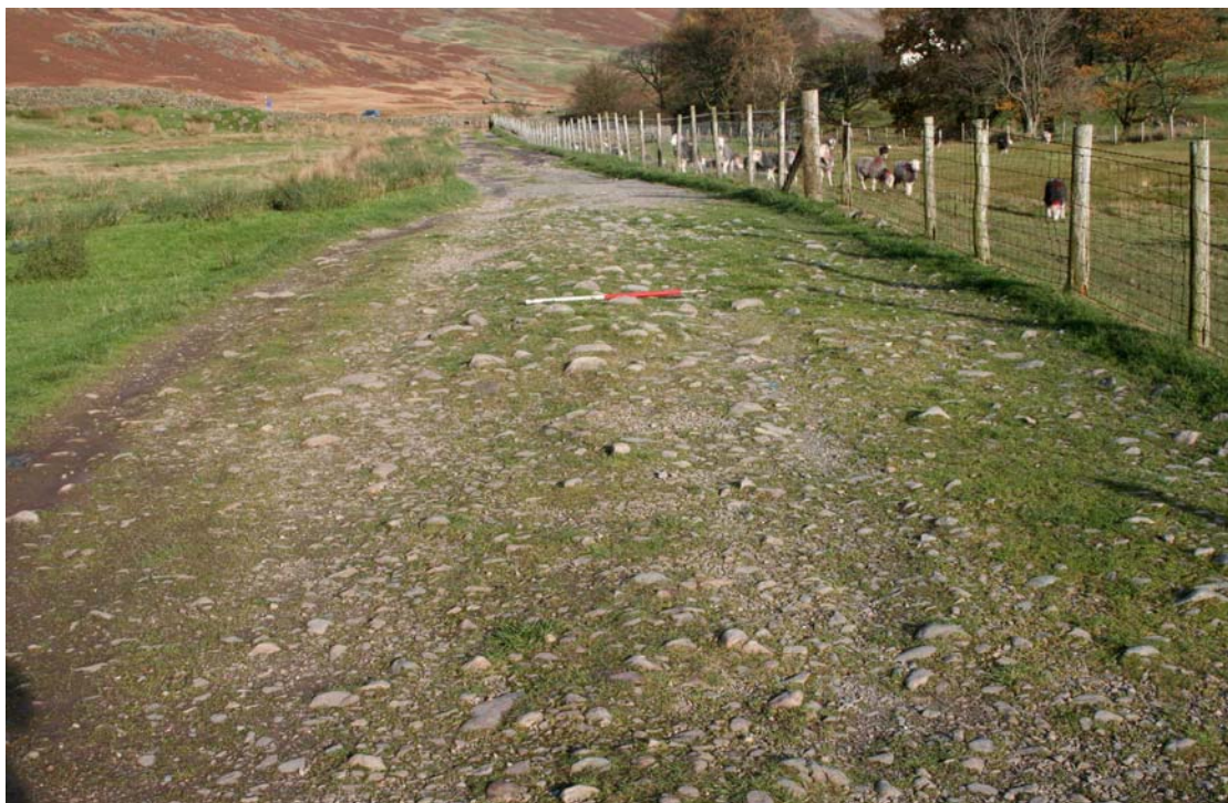
Plate 20: A broad area of erosion revealing an extensive cobbled patch (photo position 16)
