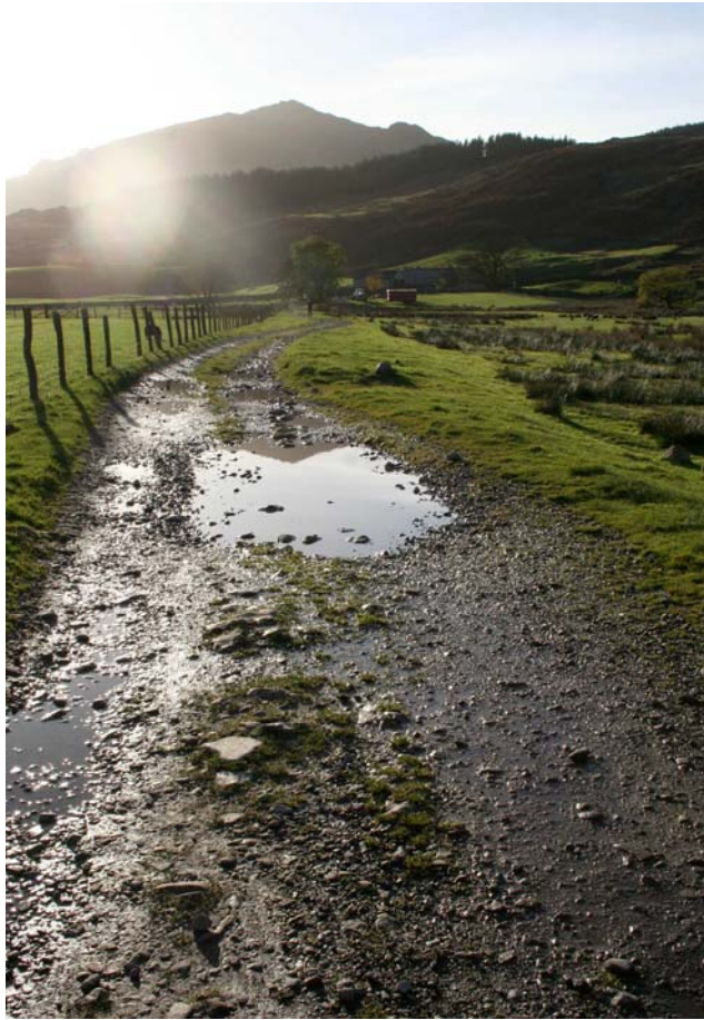
Plate 25: A view along the track (looking south-west), showing areas of erosion and surface cobbles at photo position 21
