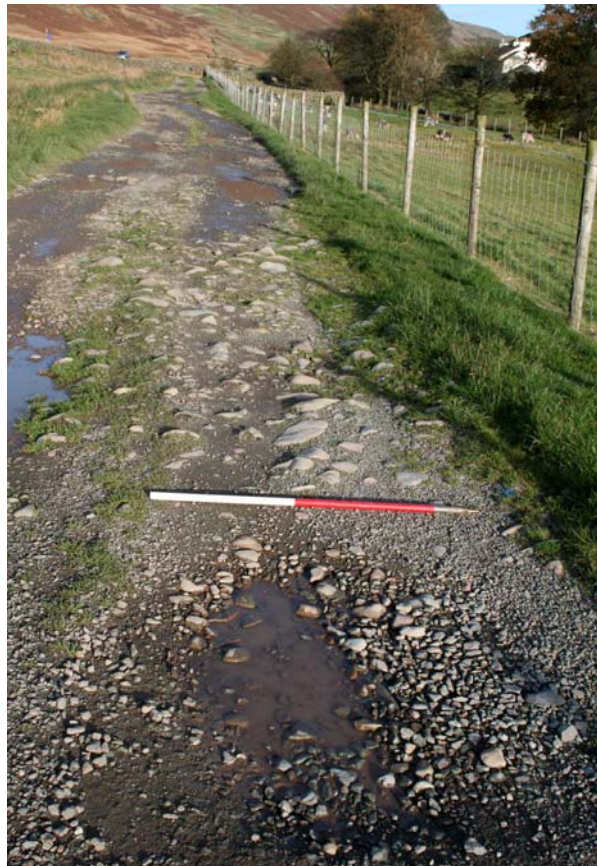
Plate 18: Cobbles exposed by vehicle wear with an absence of similar material, due to further erosion, in the pothole in the foreground (photo position 14)
