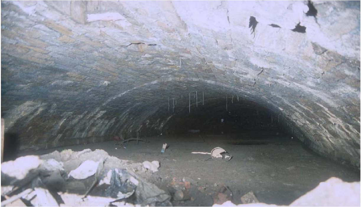
Plate 15: Internal detail of northern head-race tunnel, Trench 5
