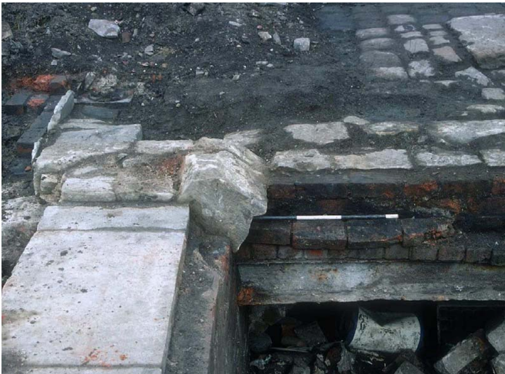
Plate 14: Dressed sandstone springer for head-race tunnel arch
