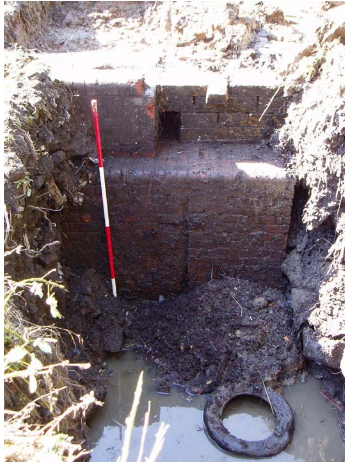
Plate 3: Brick stopping of southern head-race tunnel
