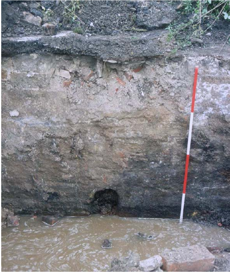
Plate 13: Floor-level aperture, north elevation, Trench 5
