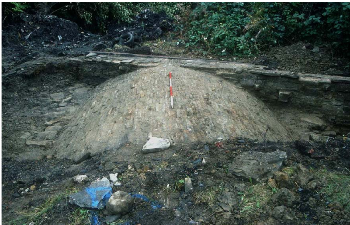
Plate 4: Crown of southern head-race tunnel
