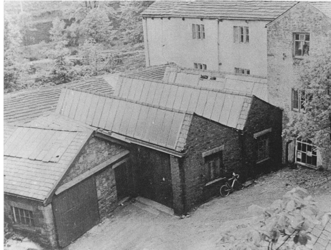
Plate 2: The boiler house (on the left) prior to demolition
