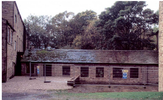
Plate 3: Looking west across site of boiler house
