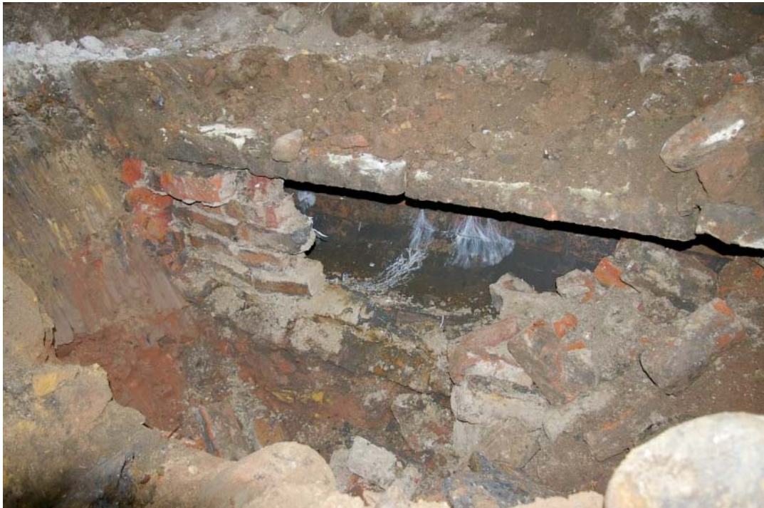
Plate 8: View of Trench 3A showing the culvert located in the sondage at the south end of the trench, looking south-east
