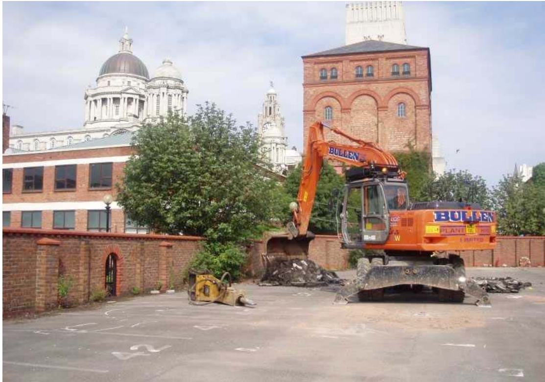
Plate 13: General working view of Trench 4, looking north
