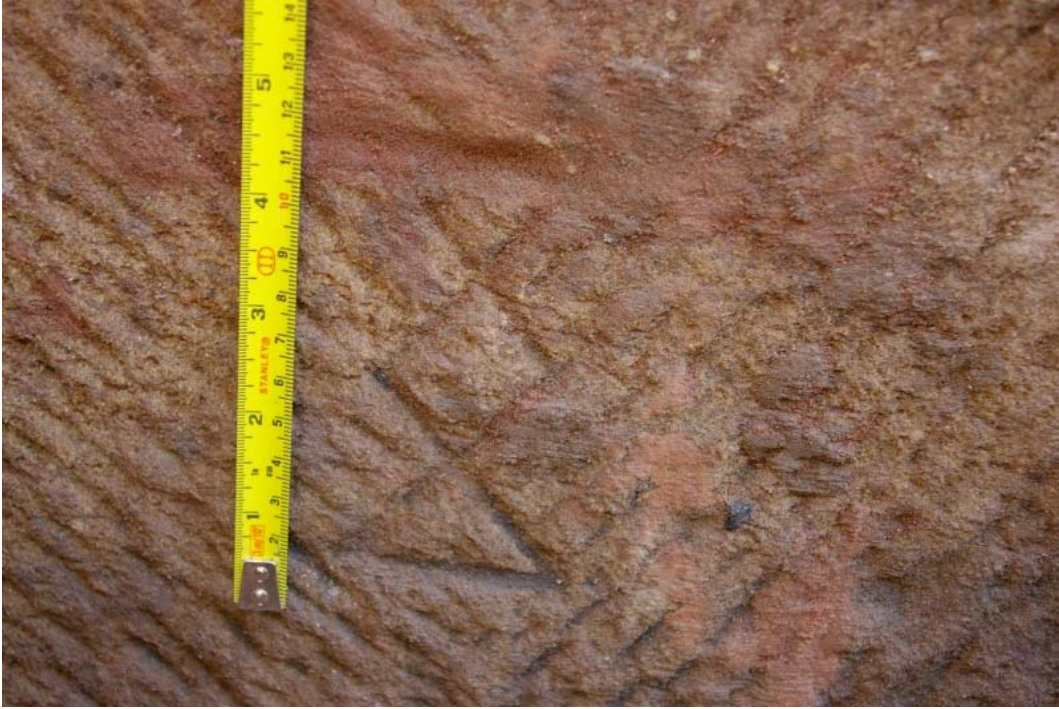
Plate 5: View of Trench 1 showing a close up of a mason's mark on the western face of Manchester Dock wall, 3109 , looking east
