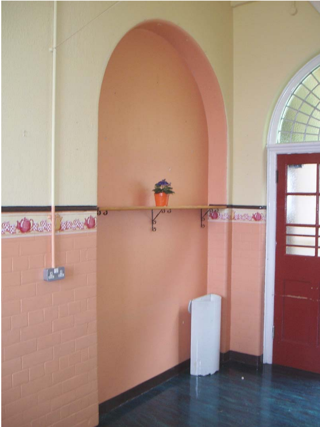
Plate 15: The blocked doorway in room F7
