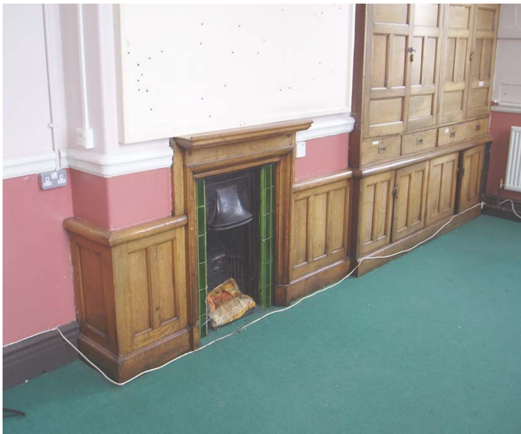
Plate 17: The fireplace in room G2
