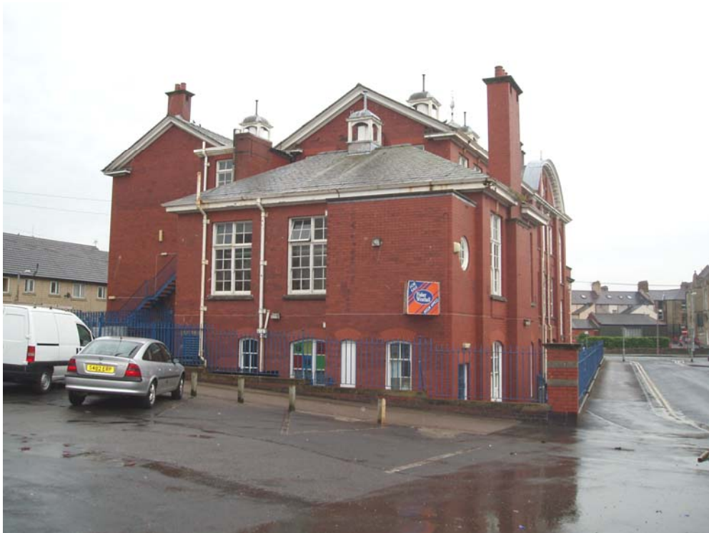
Plate 4: South-facing view of the north elevation
