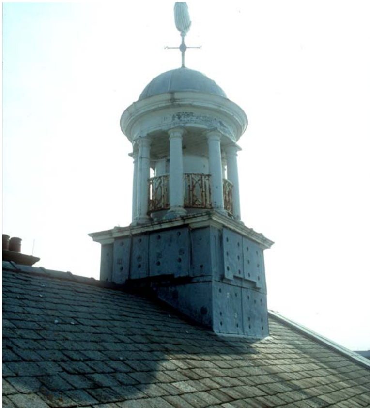
Plate 5: The cupola on the roof of the front façade
