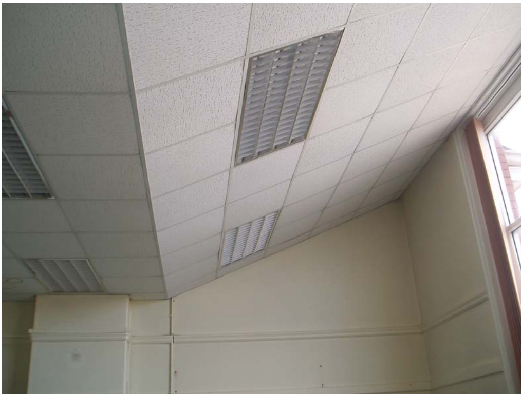
Plate 9: The modern suspended ceiling as seen in rooms F8 and F12 on the first floor
