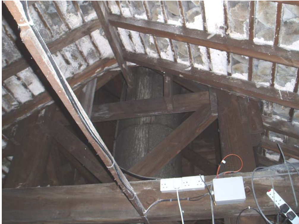
Plate 6: The central ventilation shaft of the cupola, within the roof space of the second floor
