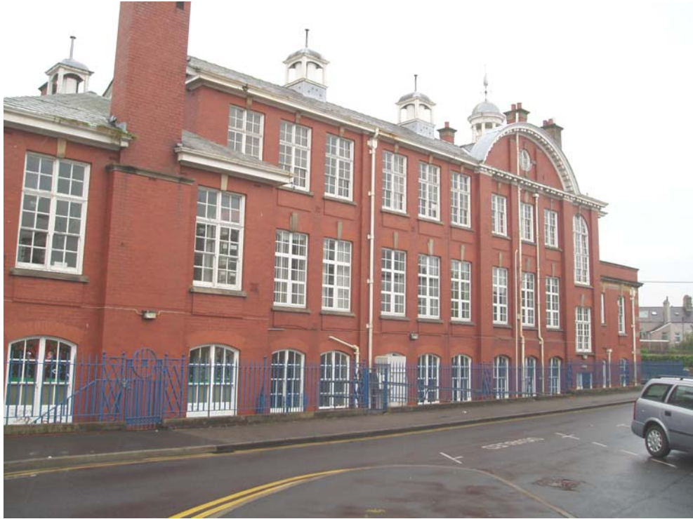
Plate 2: South-east-facing view of the west elevation
