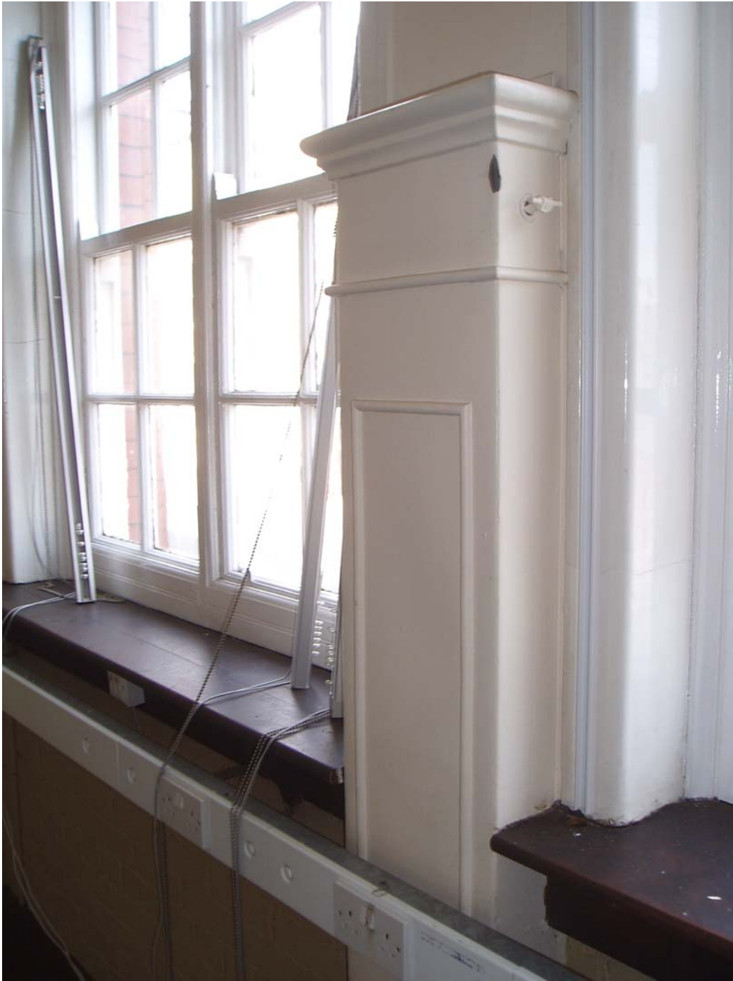
Plate 12: Detail of the fresh air inlets leading to the ventilation system in the roof
