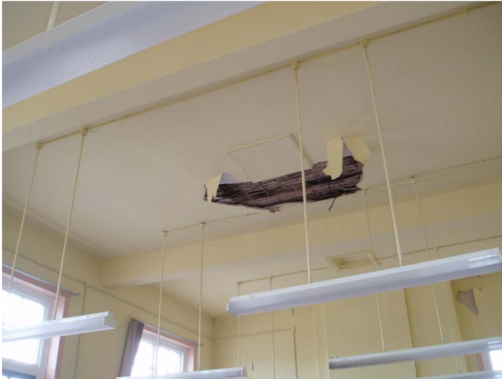
Plate 8: The lath and plaster ceiling in room F1 on the first floor
