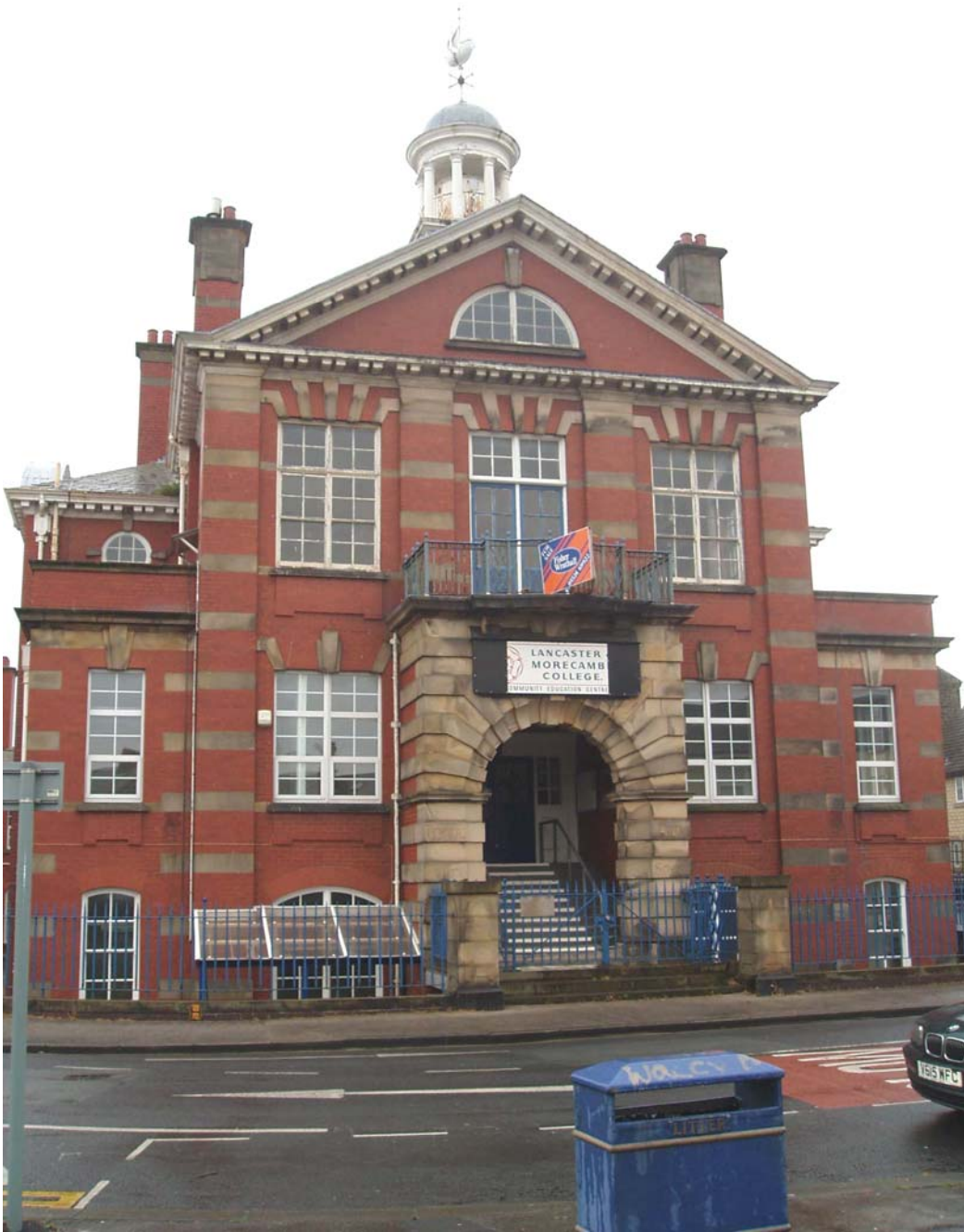
Plate 1: North-facing-view of the front (south) elevation of the Community Education Centre
