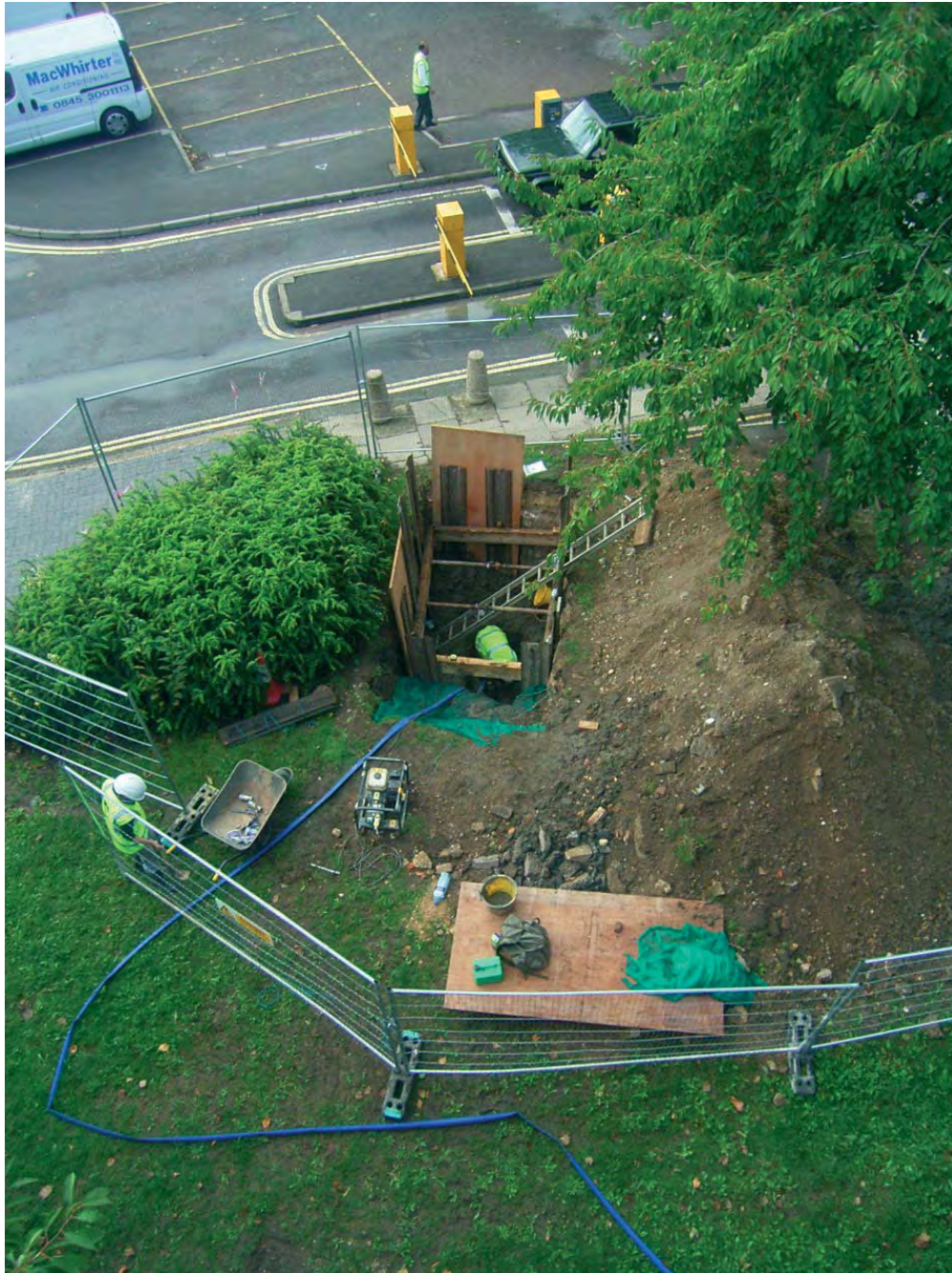
Plate 6: Trench 11 under excavation (looking South)
