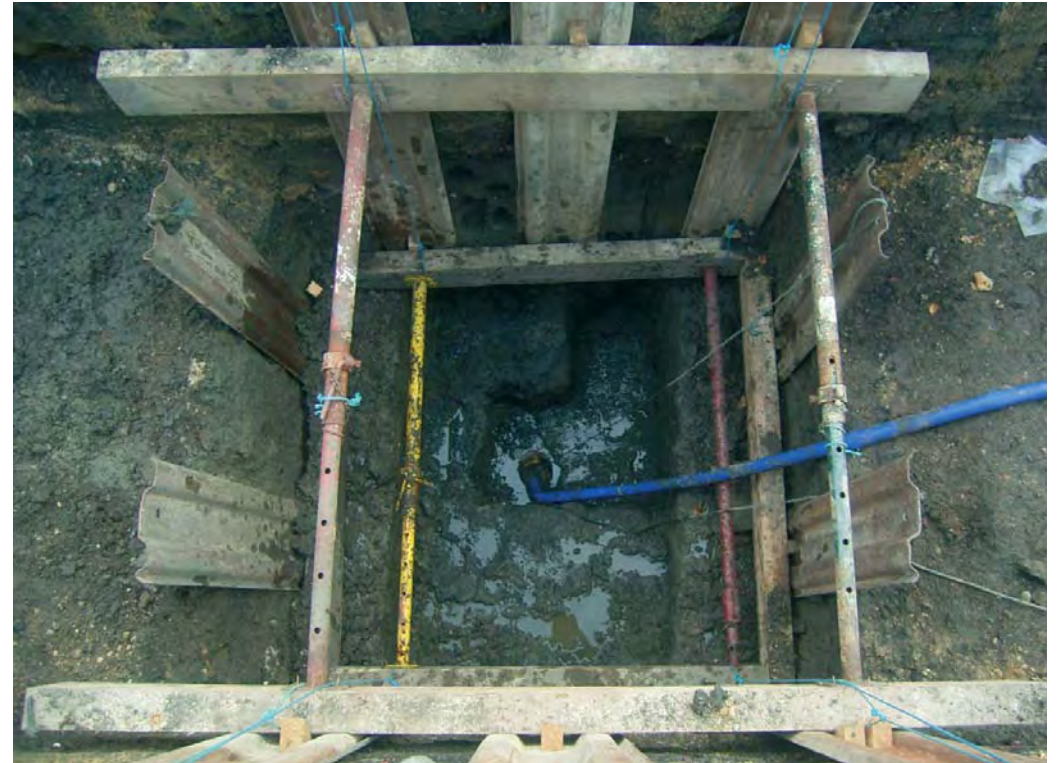
Plate 7: Open Pole Shoring, Trench 6
