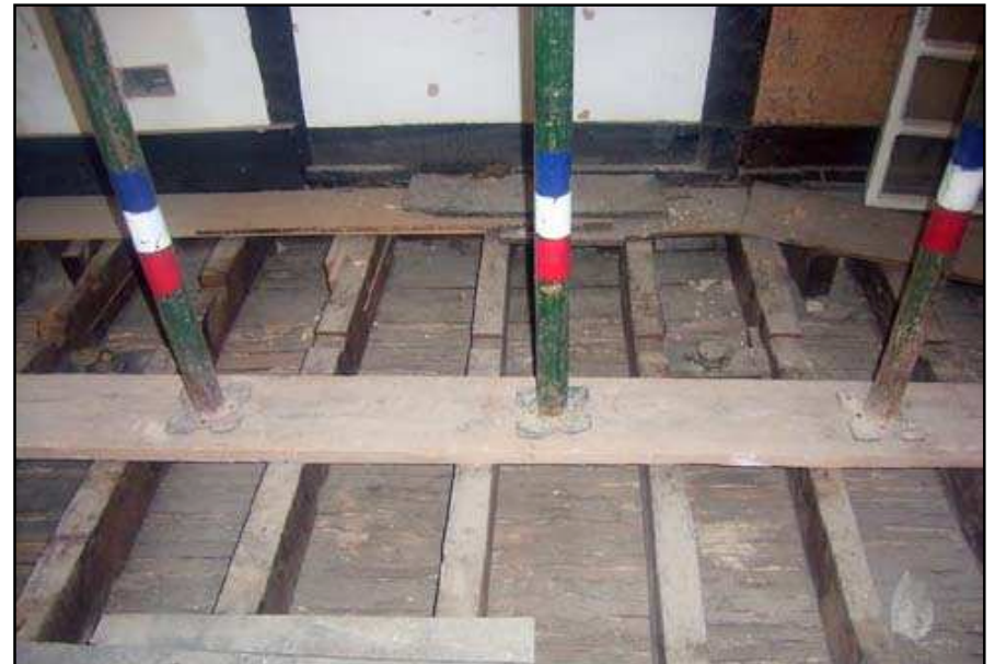
Plate 16: Floor joists in west room, first floor, No. 7 Brewer Street
