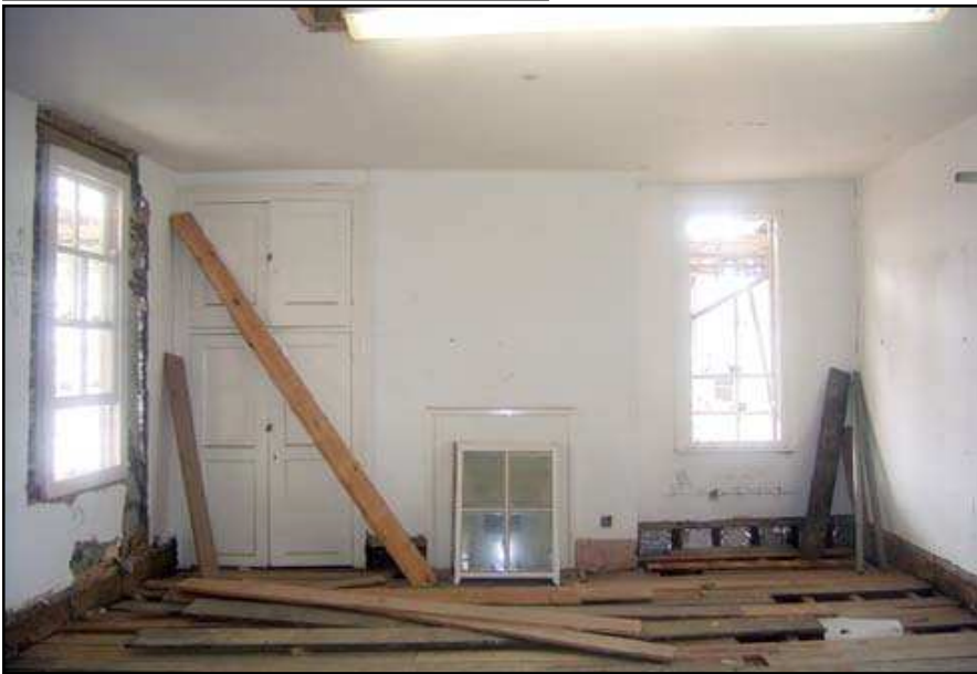
Plate 47: Second floor room of 8B, facing south, No. 8 Brewer Street
