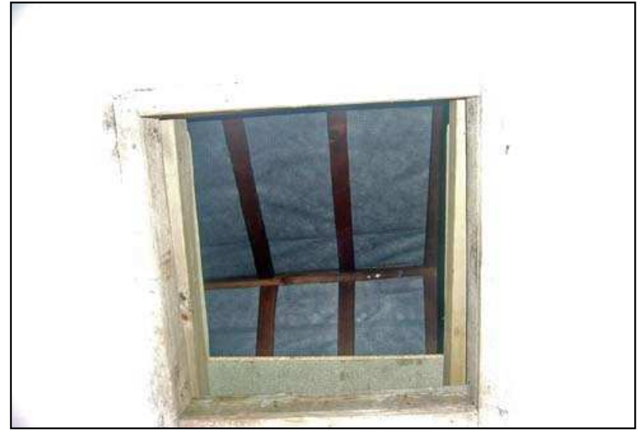
Plate 48: Roof structure of 8B, seen through hatch in ceiling of second floor.
