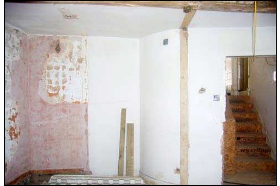
Plate 38: First floor room of 8A, facing south, No. 8 Brewer Street
