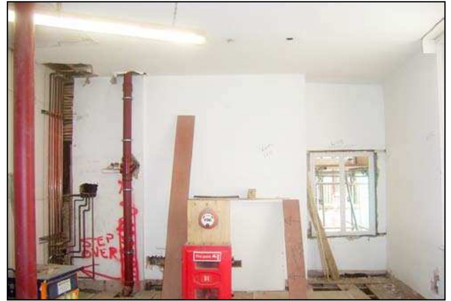
Plate 40: First floor room of 8C, facing south, No. 8 Brewer Street
