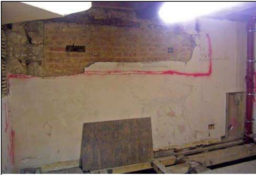
Plate 35: Red brick blocking in west wall of ground floor of 8A, No. 8 Brewer Street
