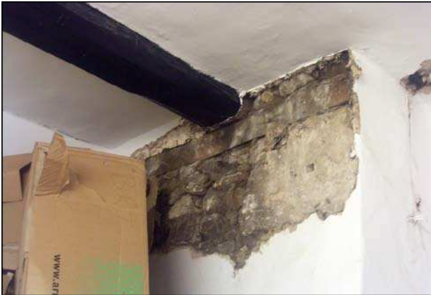
Plate 11: Exposed west chimney stack in ground floor of No. 7 Brewer Street
