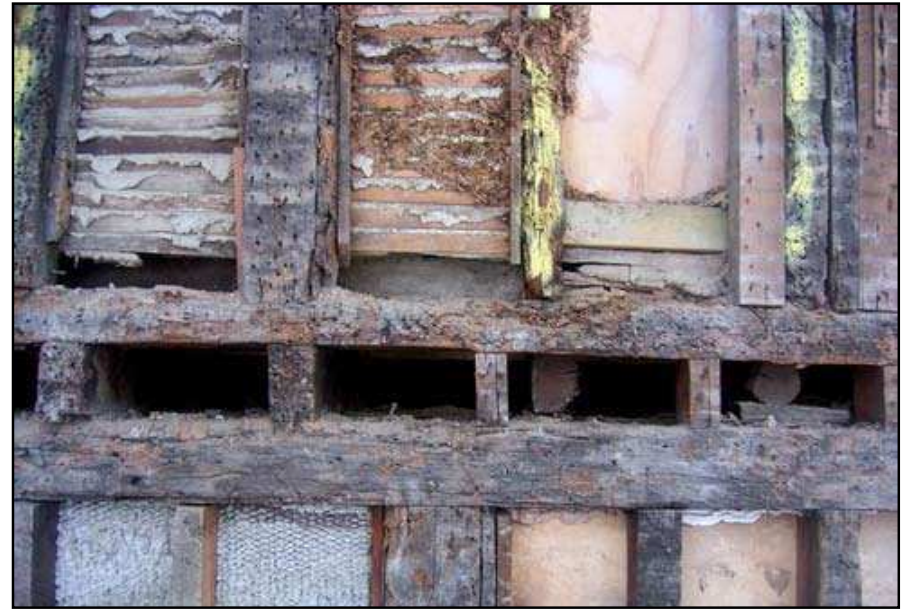
Plate 8: Wall and sill plates of north elevation showing floor joists in between
