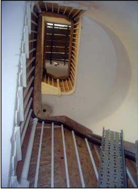
Plate 37: Stairway of 8B, No. 8 Brewer Street
