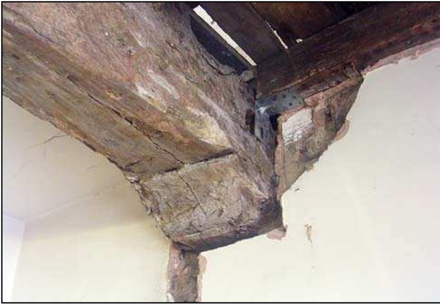
Plate 39: Chamfered truss in first floor room of 8A, No. 8 Brewer Street
