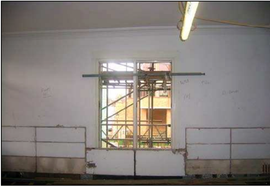
Plate 43: Second floor room of 8B, facing west, No. 8 Brewer Street
