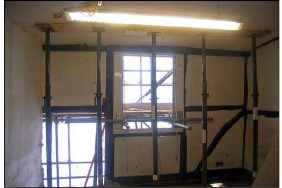
Plate 14: North wall of north room, first floor, No. 7 Brewer Street
