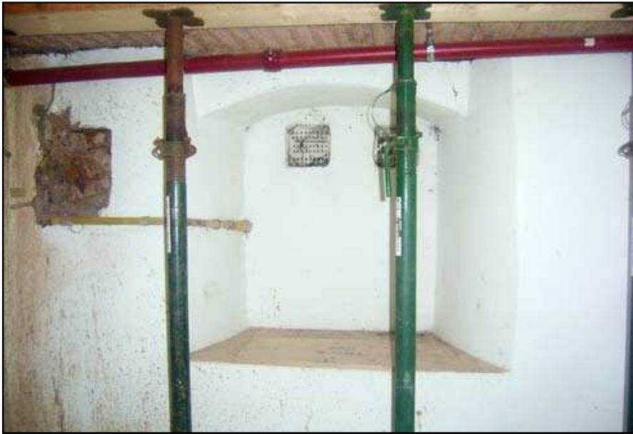
Plate 9: Alcove in north wall of cellar, No. 7 Brewer Street
