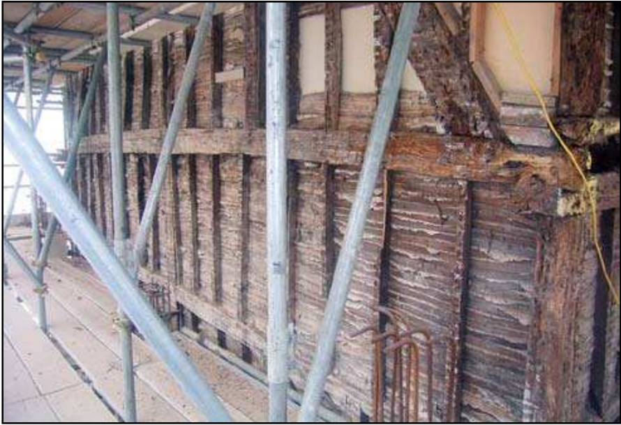
Plate 5: Timber framing on east elevation of No. 7 Brewer Street
