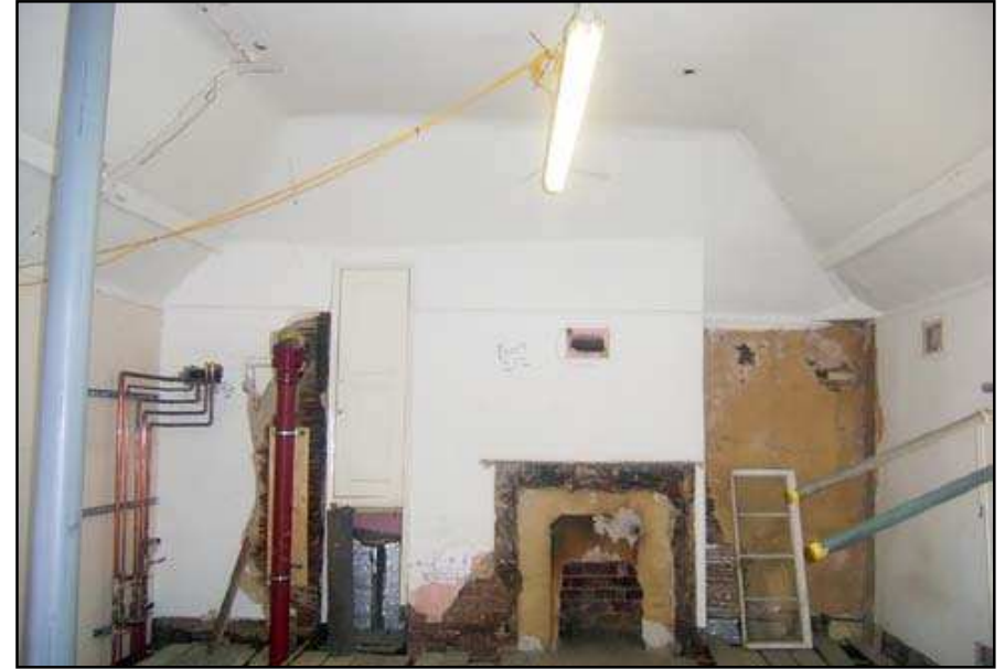
Plate 46: Second floor room of 8C, facing south, No. 8 Brewer Street
