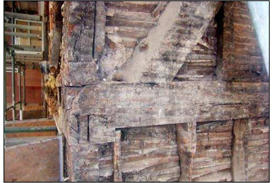
Plate 6: Pegged tenon and mortice joint, east elevation of No. 7 Brewer Street
