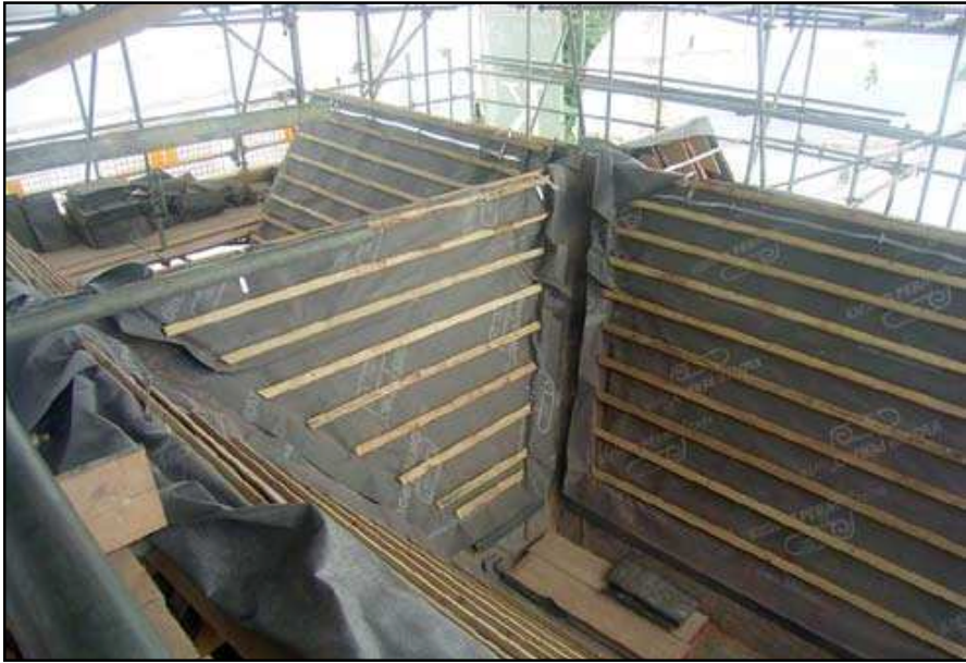
Plate 27: Roof structure of No. 7 Brewer Street, facing north east
