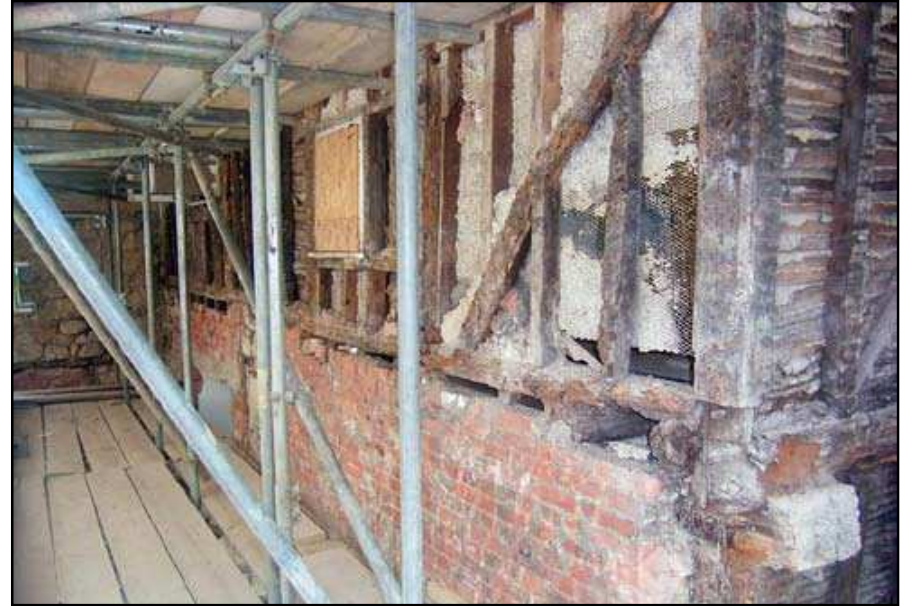
Plate 2: Later red brick wall on Ground Floor of No. 7 Brewer Street
