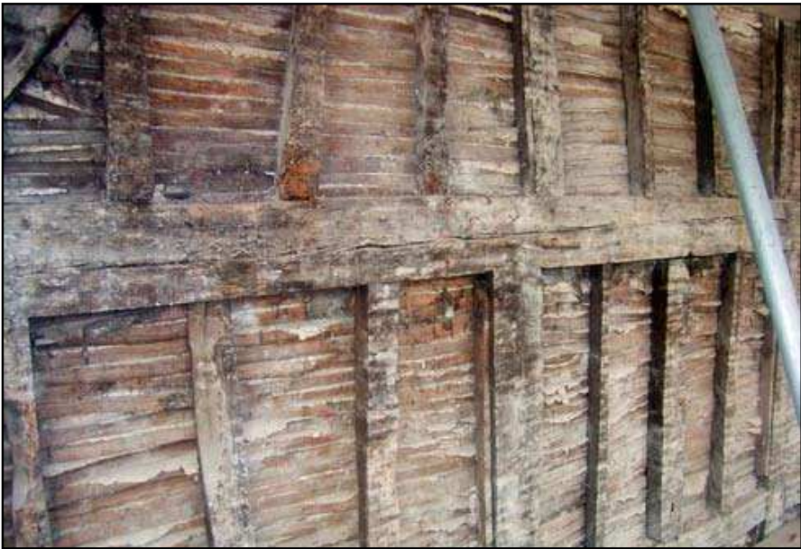
Plate 3: Timber framing on east elevation of No. 7 Brewer Street
