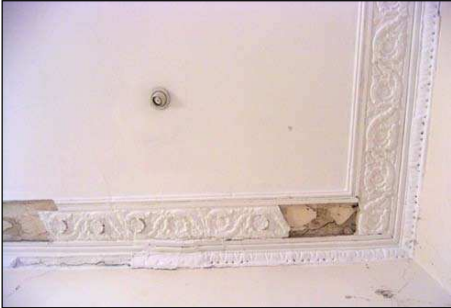
Plate 33: Cornice in ground floor of 8B, No. 8 Brewer Street
