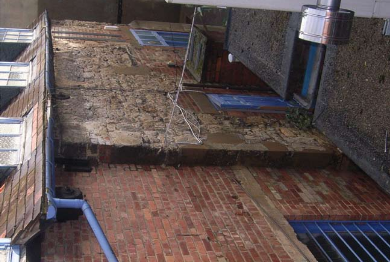
Plate 2: Stone section of south wall of 6 Brewer Street
