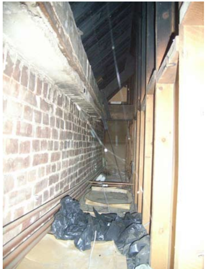
Plate 14: Charred roof boards in void on north side of 6 Brewer St.
