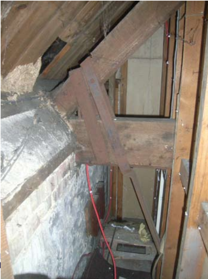
Plate 13: End of tie-beam in 6 Brewer St.
