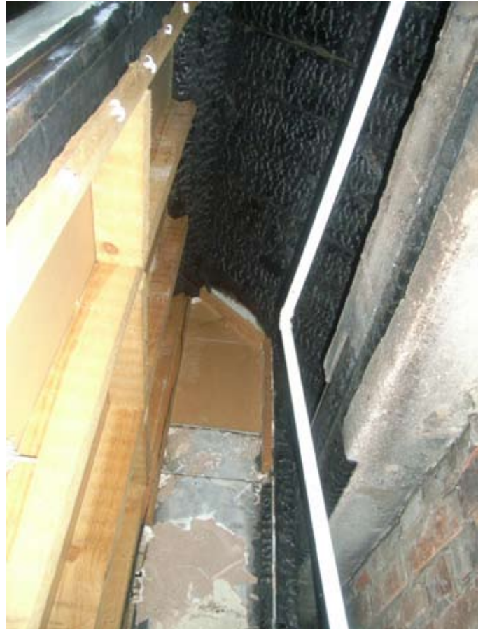
Plate 14: Charred roof boards in void on north side of 6 Brewer St.
