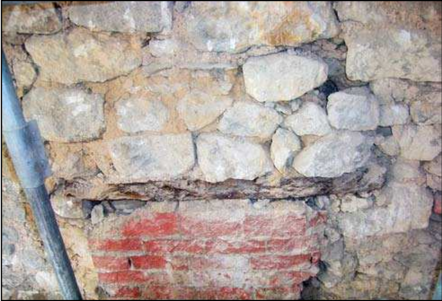
Plate 1: Primary limestone rubble coursing and later red brick patching on Ground Floor of No. 7 Brewer Street
