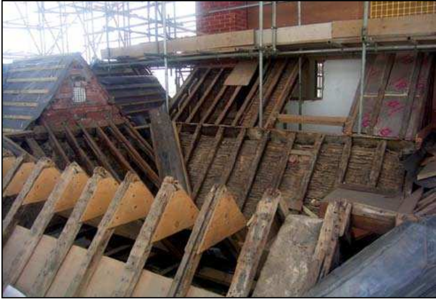
Plate 49: Roof structures of No. 7 (left), 8A (foreground) and 8B (background), facing south
