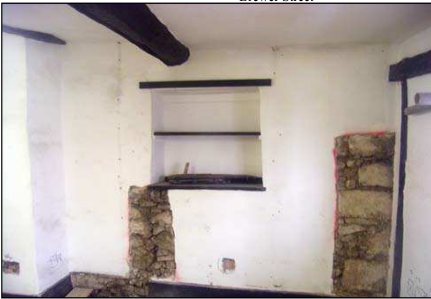
Plate 23: West party wall with alcove, second floor, No. 7 Brewer Street
