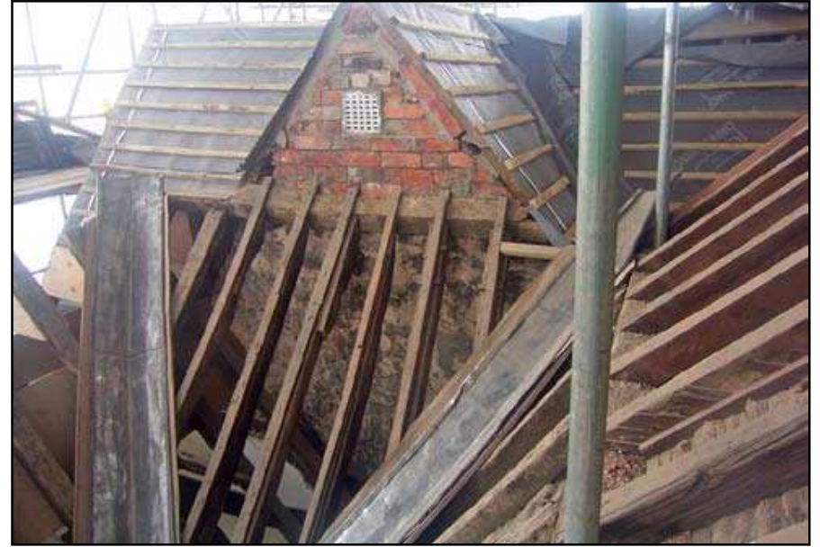
Plate 50: Roof structures of 8B (foreground) and No. 7 (background), facing east
