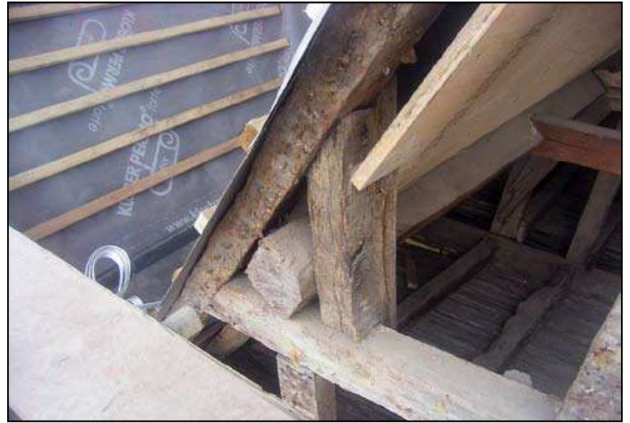
Plate 28: Structure of north dormer showing purlin, No. 7 Brewer Street
