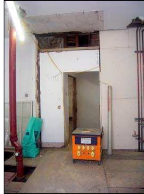
Plate 42: East doorway of first floor room of 8C, No. 8 Brewer Street
