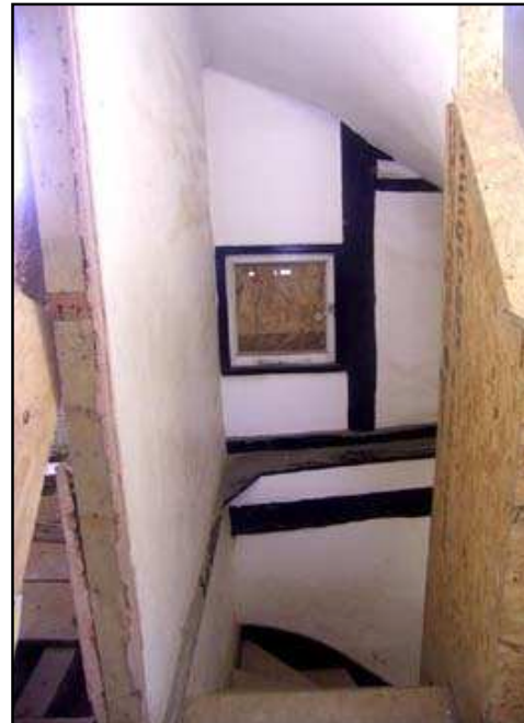
Plate 12: Stairway between ground and first floor, facing south, No. 7 Brewer Street
