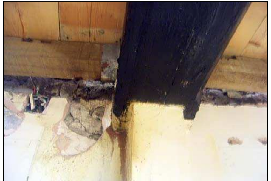
Plate 36: Chamfered truss in ground floor of 8A, No. 8 Brewer Street
