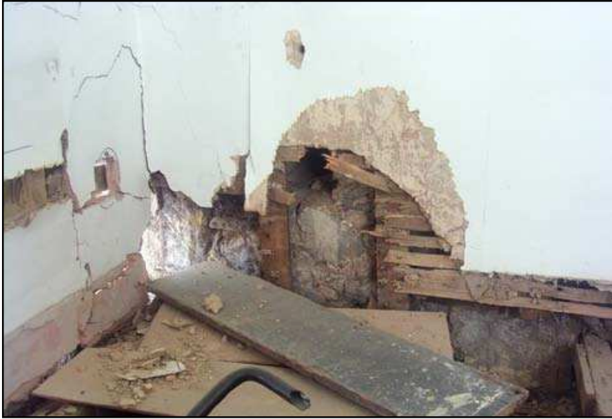
Plate 41: North east corner of first floor room of 8C, No. 8 Brewer Street
