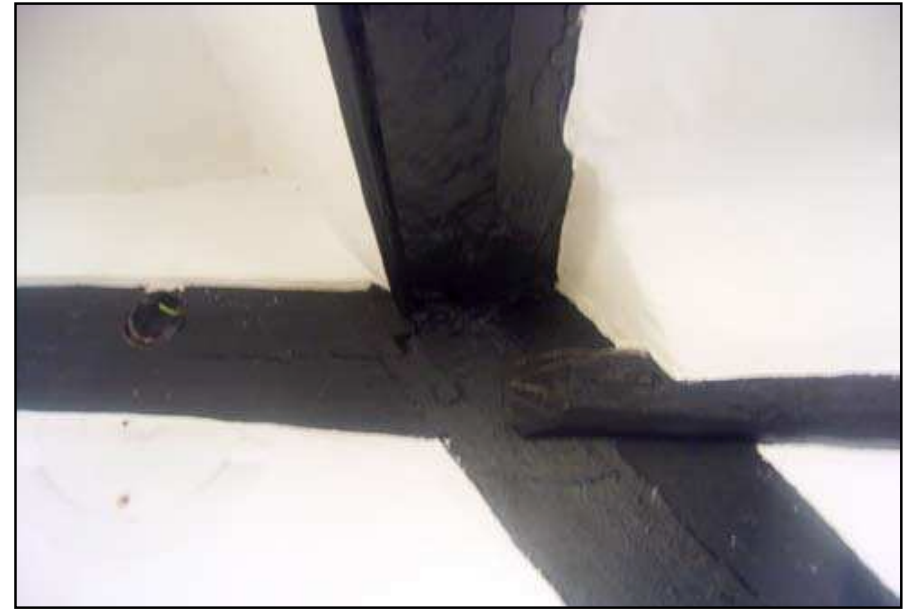
Plate 20: Butt purlin in roof, facing west, second floor, No. 7 Brewer Street
