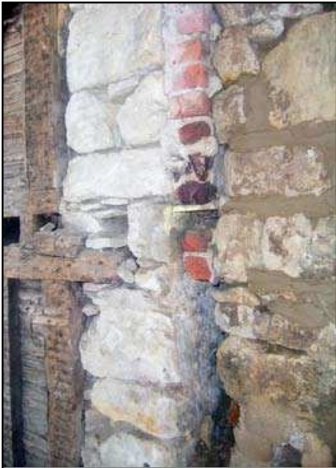
Plate 5: Timber framing on east elevation of No. 7 Brewer Street
