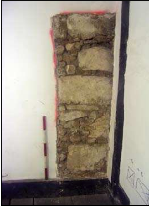
Plate 21: Exposed masonry in west party wall, second floor, No. 7 Brewer Street
