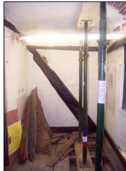
Plate 24: Principal rafter in east wall of south west room, second floor, No. 7 Brewer Street
