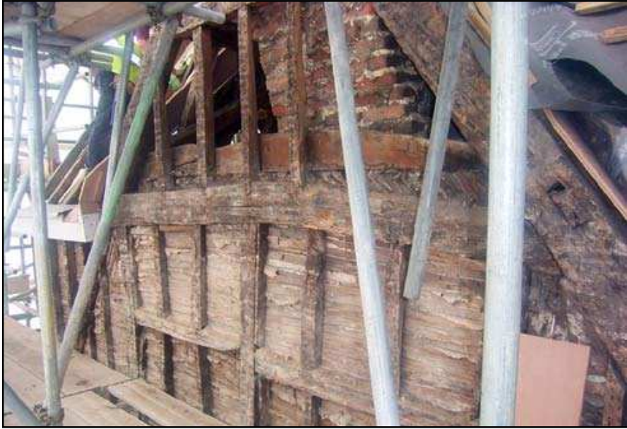
Plate 25: East gable of roof of No. 7 Brewer Street
