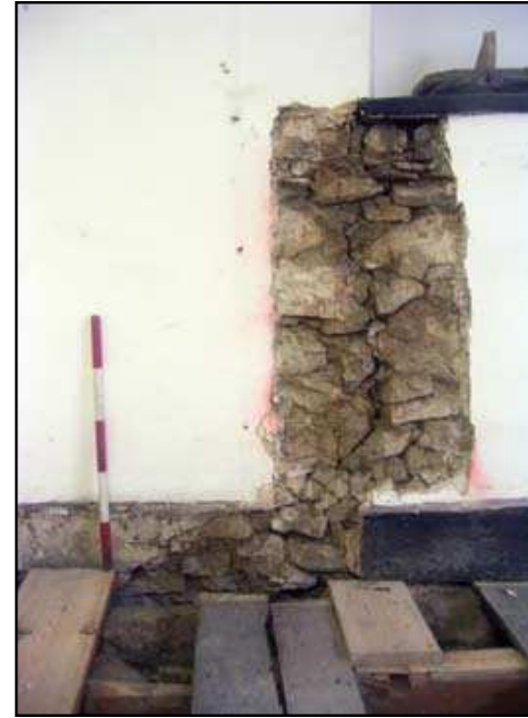
Plate 22: Exposed masonry in west party wall, second floor, No. 7 Brewer Street
