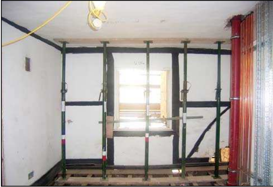
Plate 13: South wall of west room, first floor, No. 7 Brewer Street
