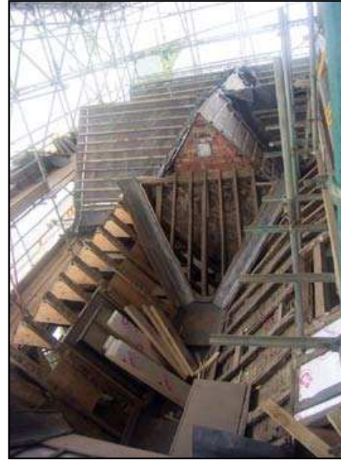
Plate 30: Roof structures of No. 7 and part of No. 8, facing east
