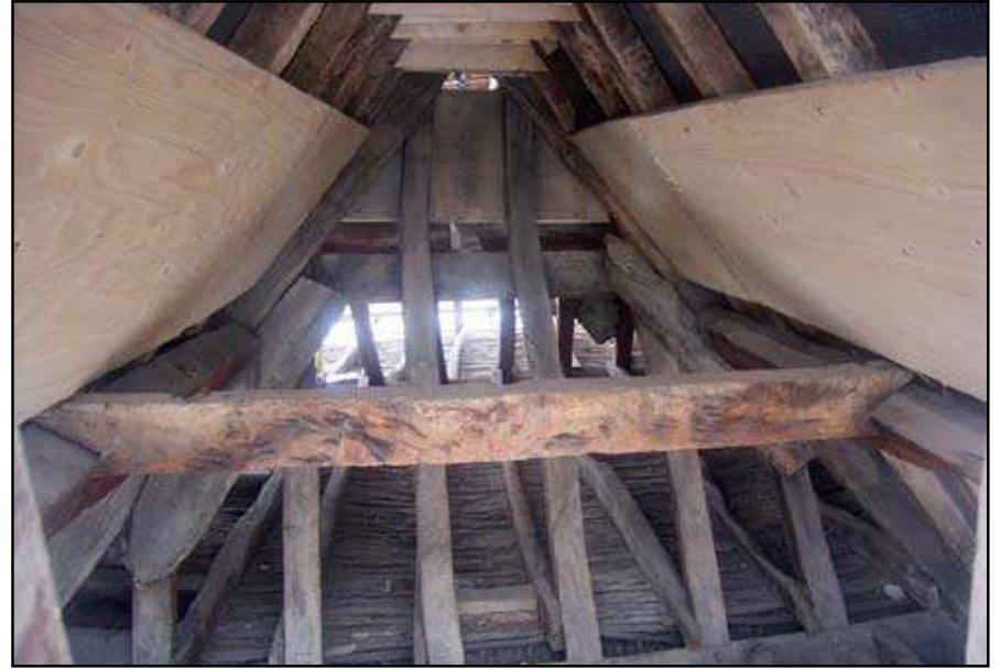
Plate 26: Interior of north dormer, No. 7 Brewer Street
