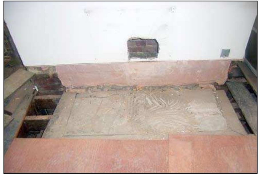
Plate 44: Hearth in first floor room of 8B, facing south, No. 8 Brewer Street
