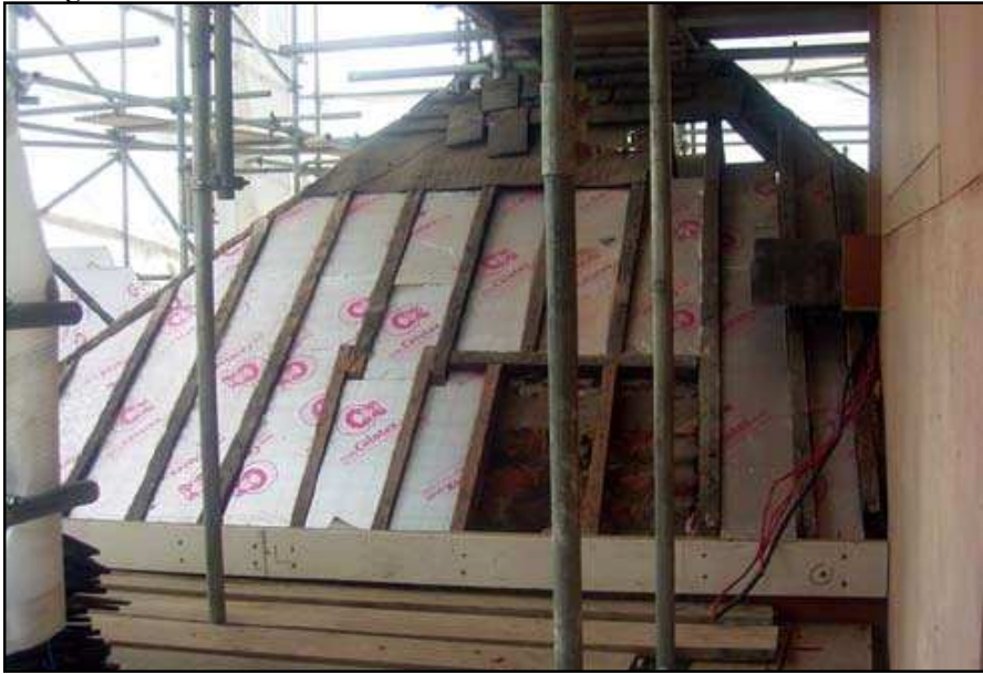
Plate 51: Roof structure of 8C, facing north
