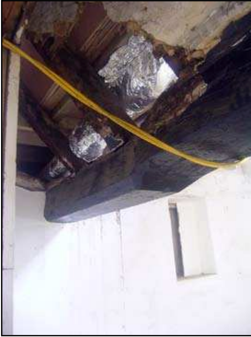
Plate 45: Chamfered ceiling beam in second floor room of 8A, facing west, No. 8 Brewer Street
