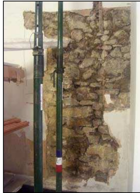
Plate 10: Exposed west stone party wall in ground floor of No. 7 Brewer Street
