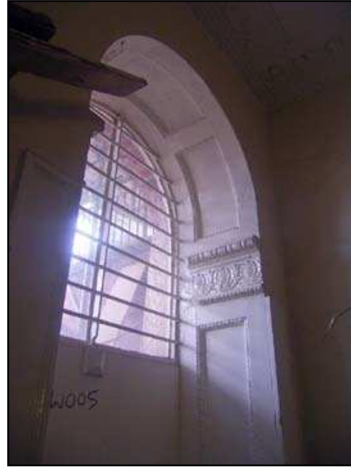
Plate 34: Window surround in ground floor of 8B, No. 8 Brewer Street
