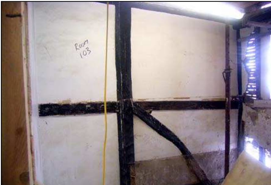
Plate 15: East wall of south room, first floor, No. 7 Brewer Street
