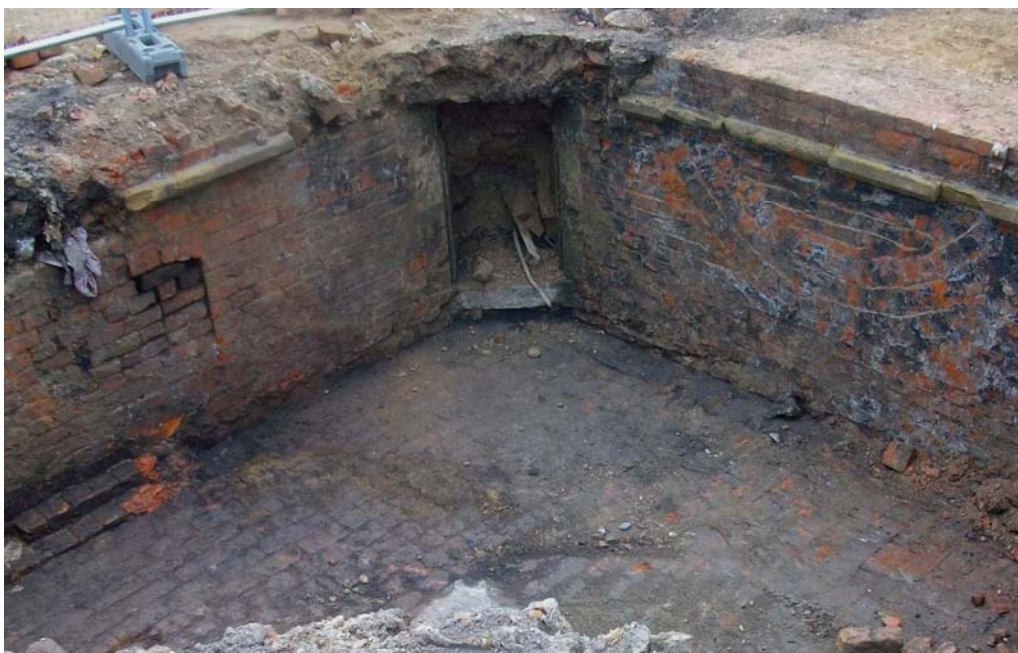
Plate 14: Doorway with stone embrasure at south-west corner of tower basement
