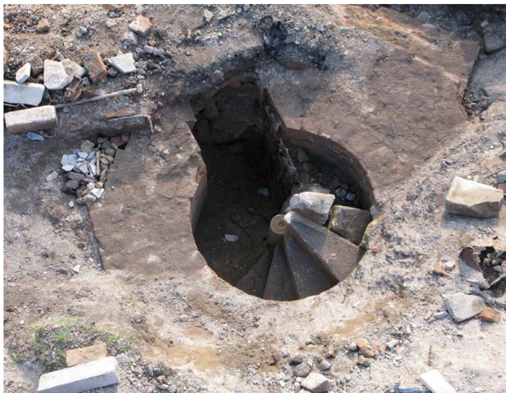
Plate 12: The excavated foundations for the north-east corner of the tower
