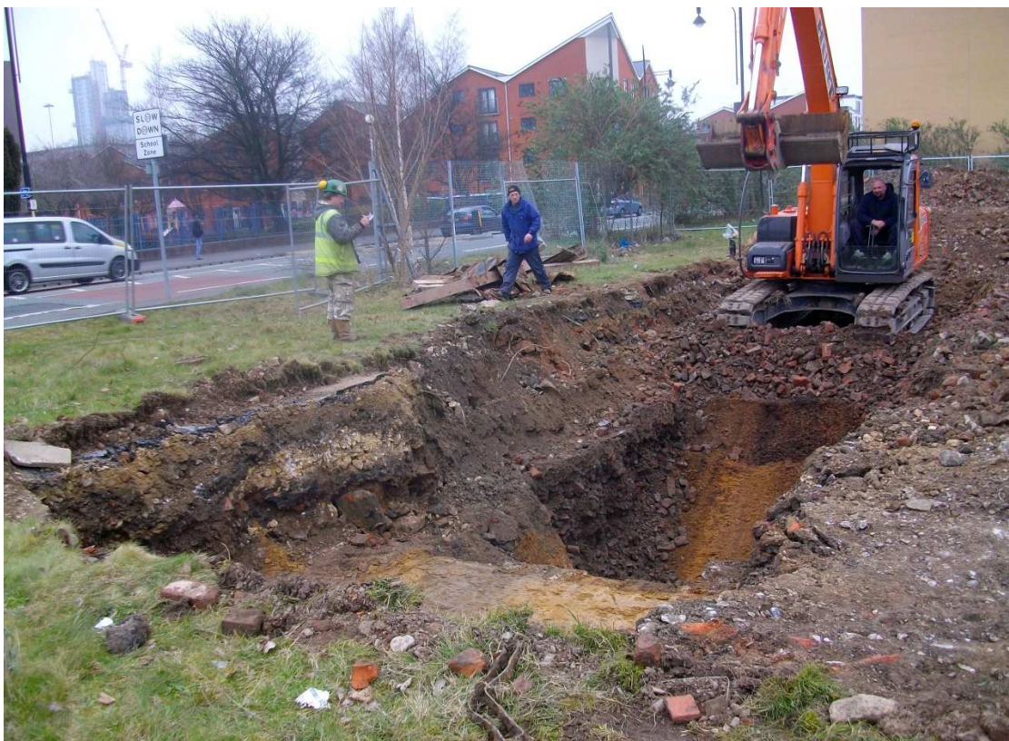
Plate 29: General view of the demolition rubble and natural deposits exposed in Trench 3
