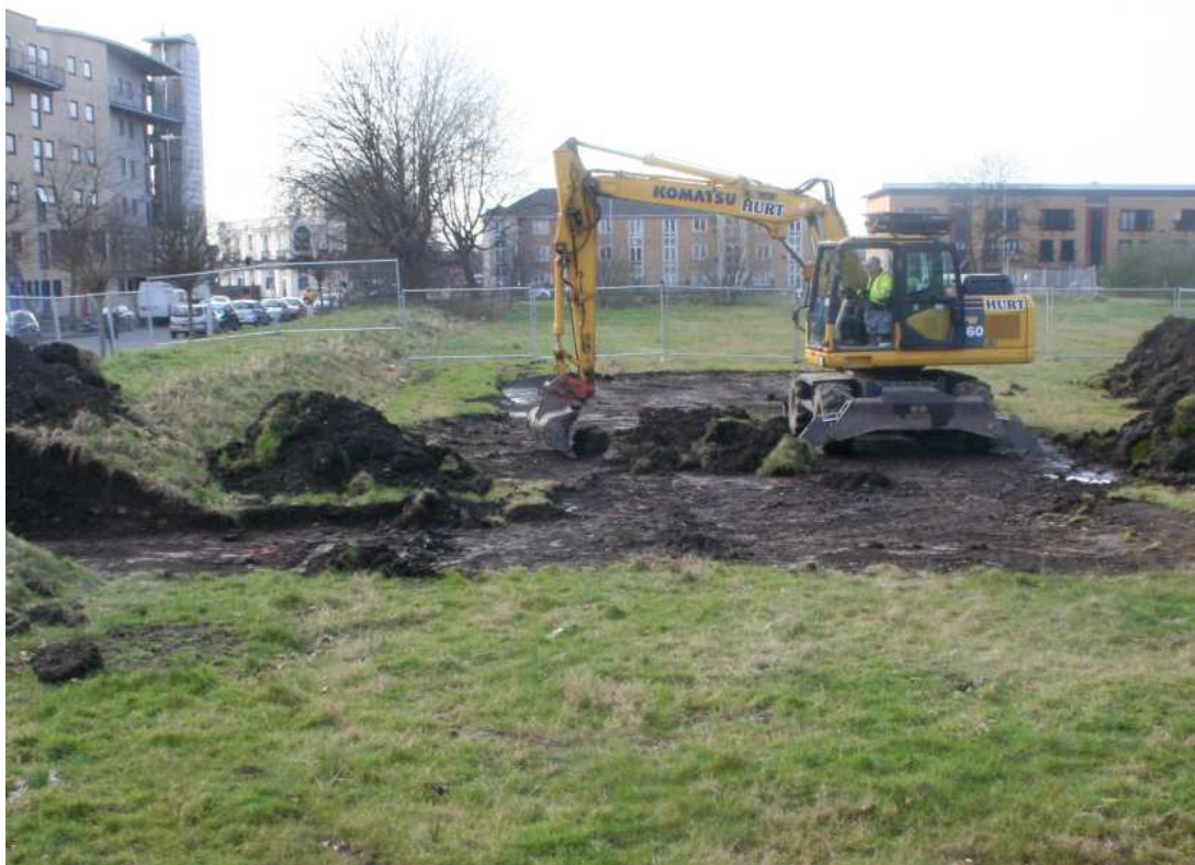
Plate 7: Mechanical stripping of Trench 1
