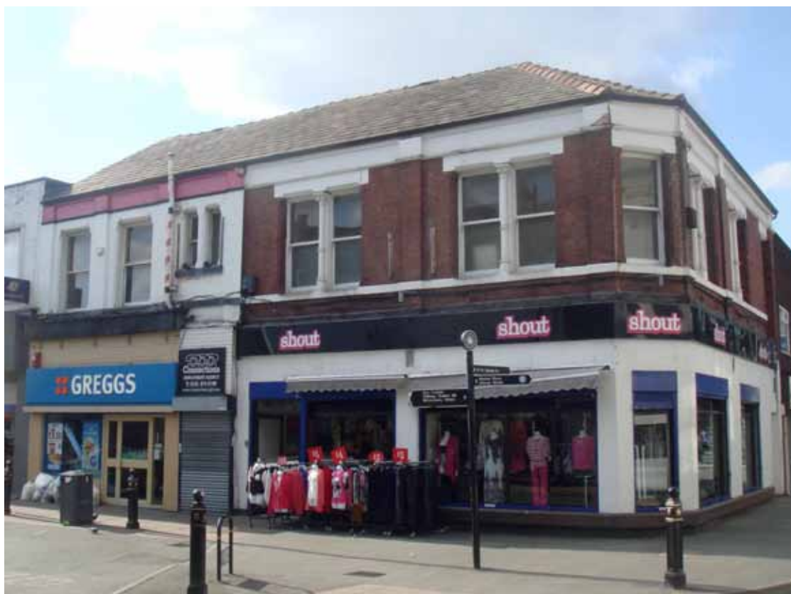
Plate 3: Nos 76-80 Prince's Street (Site 05)
