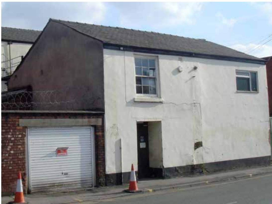
Plate 4: Building on Bridgefield Street to the rear of nos 38-40 Prince's Street (Site 10b)
