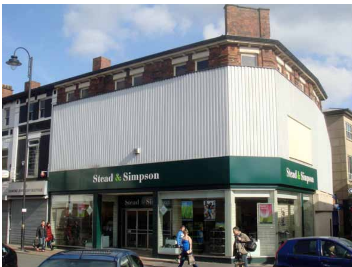
Plate 6: Nos 87-91 Prince's Street (Site 44)
