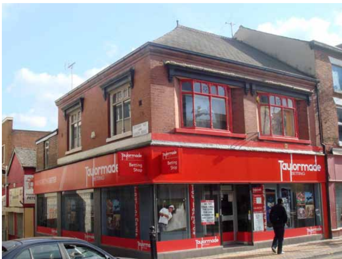
Plate 5: Nos 29-33 Prince's Street (Site 41)
