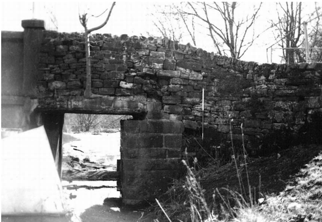
Plate 73: South-western wing wall (11) and sandstone abutment (12) (MF SB06_01)
