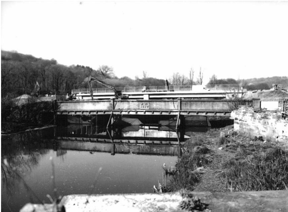
Plate 19: West-facing view across the river Calder showing the south-east-facing elevation of Sterne Bridge (MF SB04_12)
