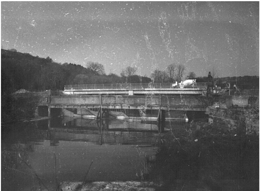
Plate 4: South-east-facing elevation of Sterne Bridge (MF SB01_03)
