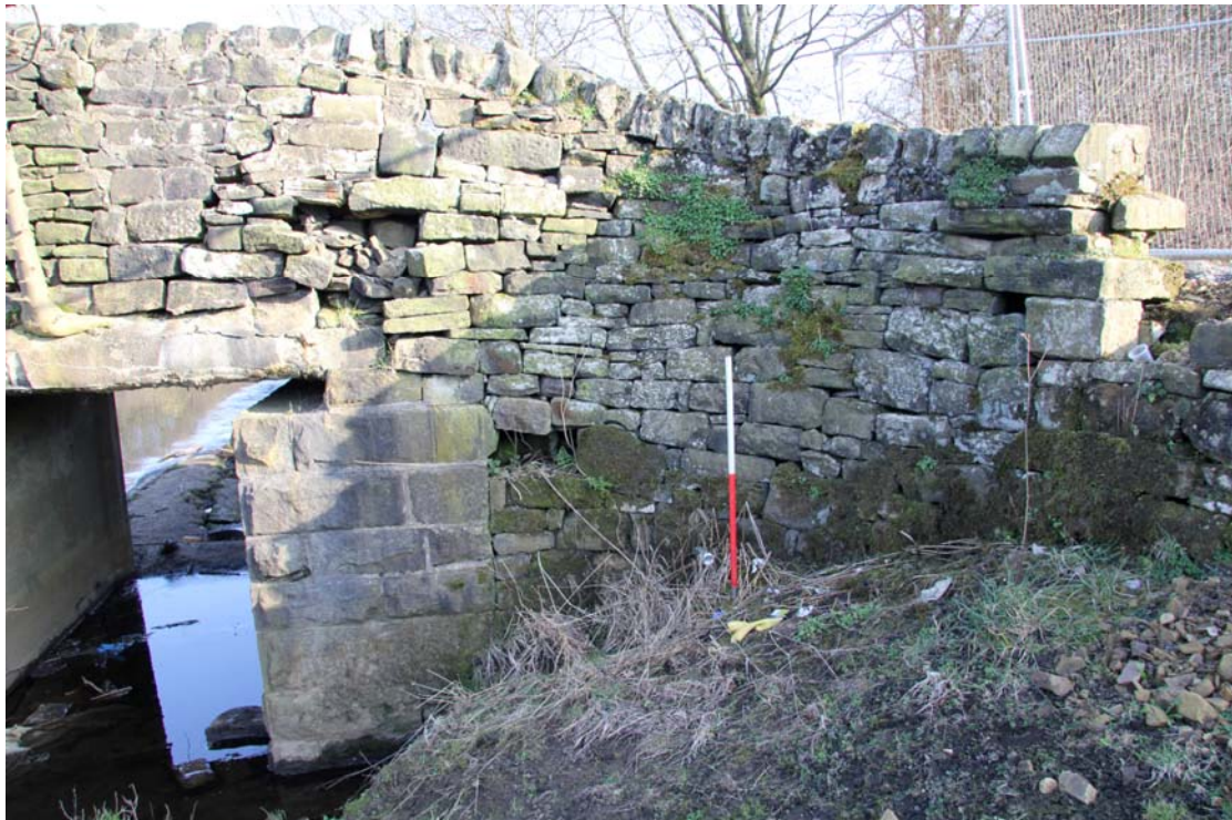
Plate 68: Interface between the south-east wing wall (11) and stone abutment (12) (IMG_2424)
