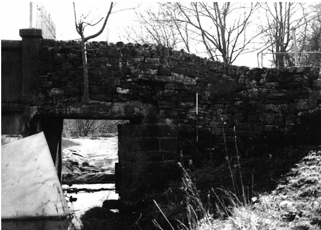
Plate 75: South-western wing wall (11) and sandstone abutment (12) (MF SB06_03)
