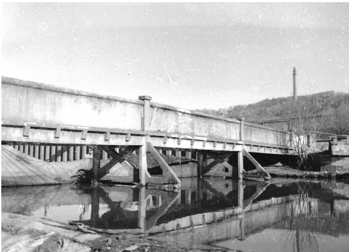
Plate 34: North-facing view showing south-east-facing bridge elevation, trestles (4a) and (4b), and cut-waters (5) and (5a) (MF SB03_05)
