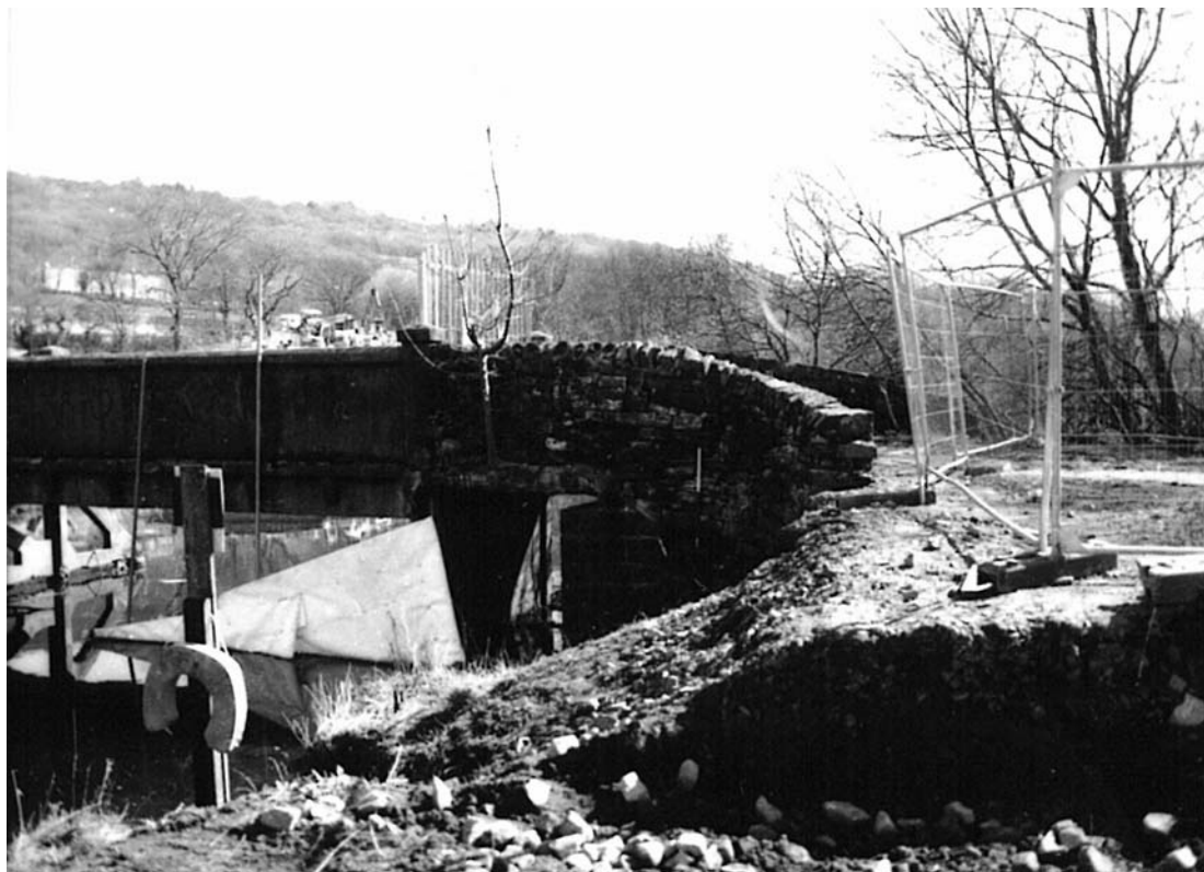
Plate 77: South-western wing wall (11) and sandstone abutment (12) (MF SB06_06)
