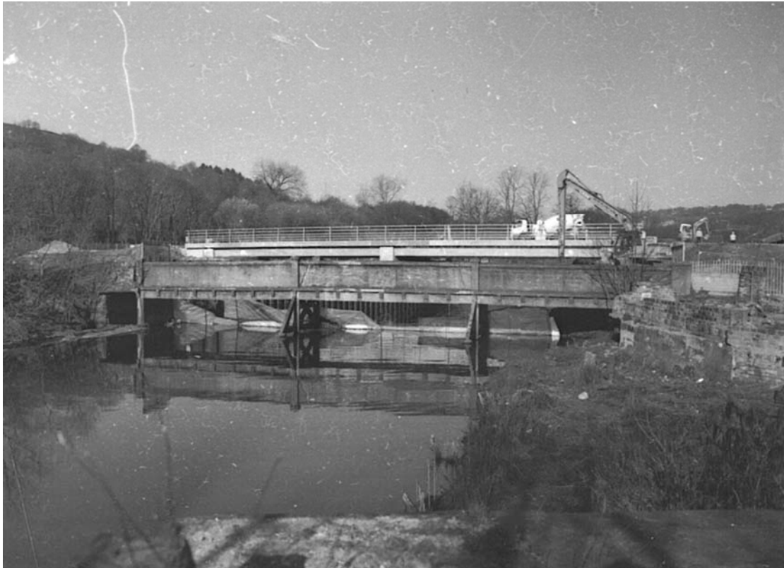
Plate 5: South-east-facing elevation of Sterne Bridge (MF SB01_04)
