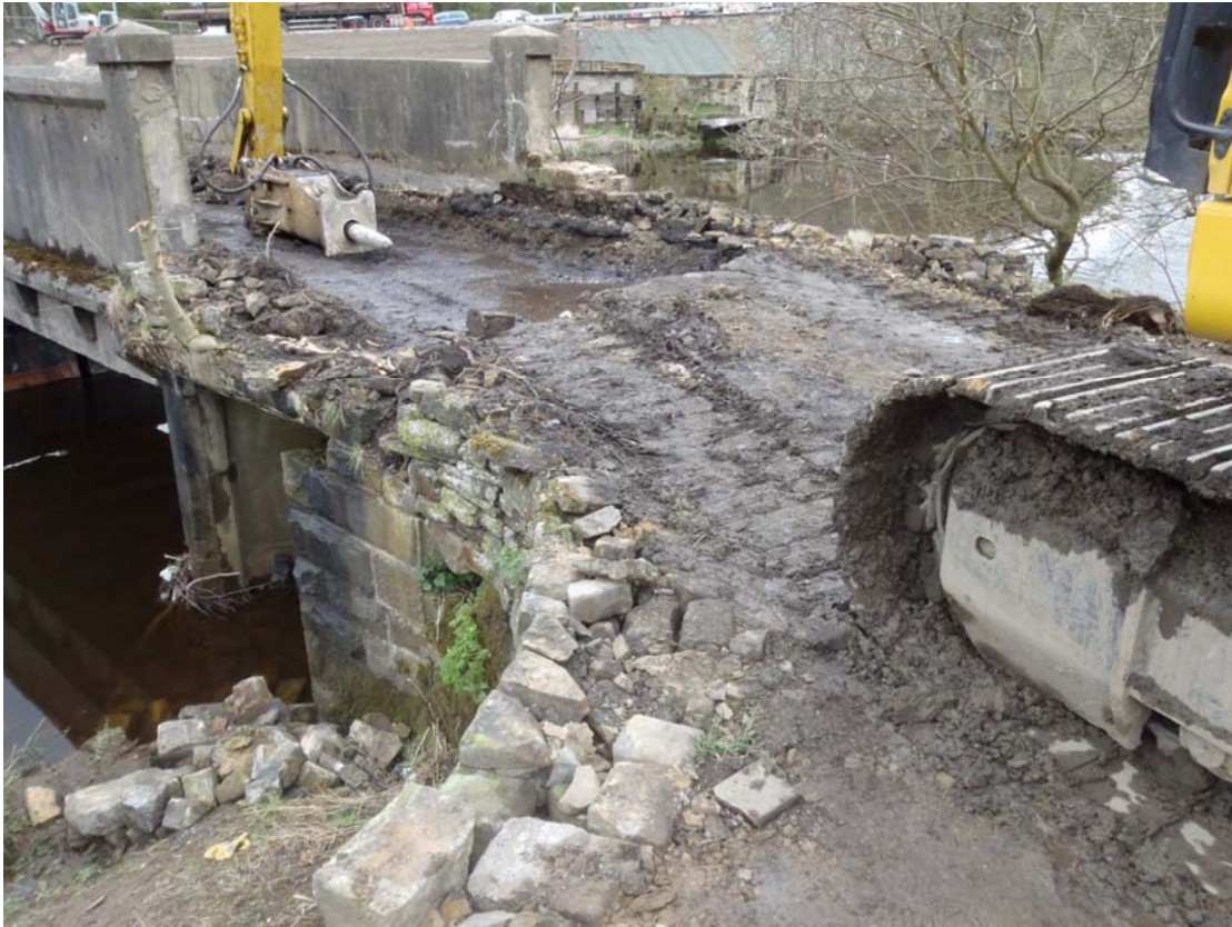
Plate 89: East-facing view across the demolished parapet and wing walls (11) (P3020745.JPG)
