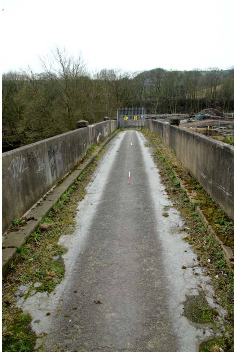
Plate 84: View across the bridge to the southern bank, showing the bridge deck (14) flanked by concrete parapet walls (10) (IMG_2361)
