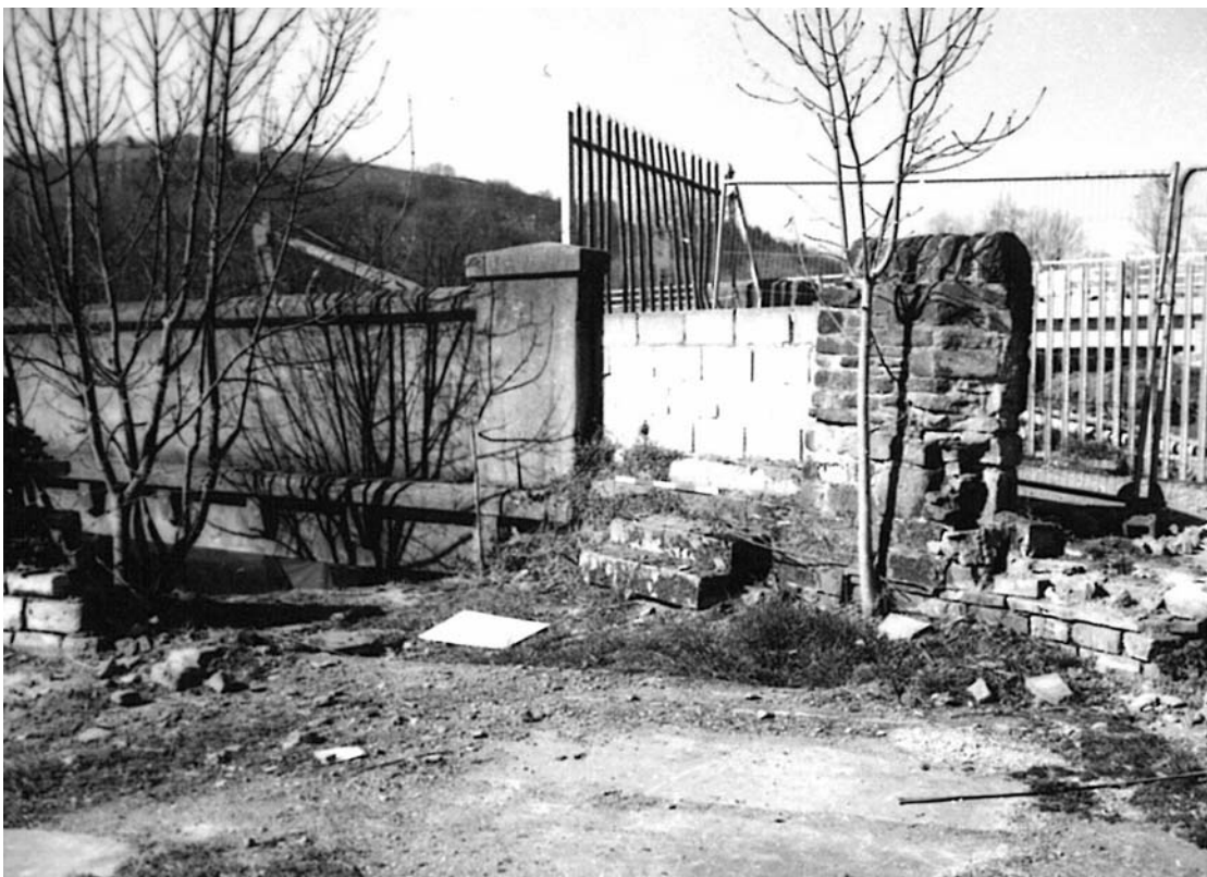
Plate 16: Stepped access (1) and vertical sandstone pillar (2) (MF SB05_01)
