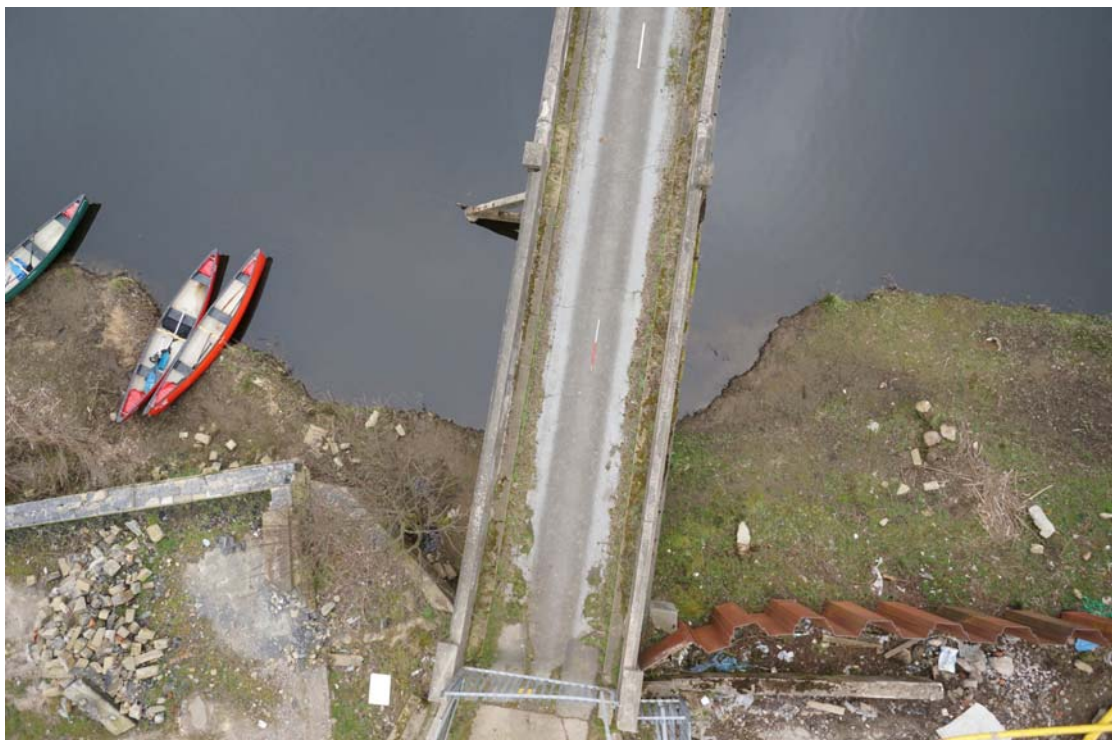
Plate 81: Aerial view showing bridge deck (14) flanked by parapet walls (10) (DSC00475)
