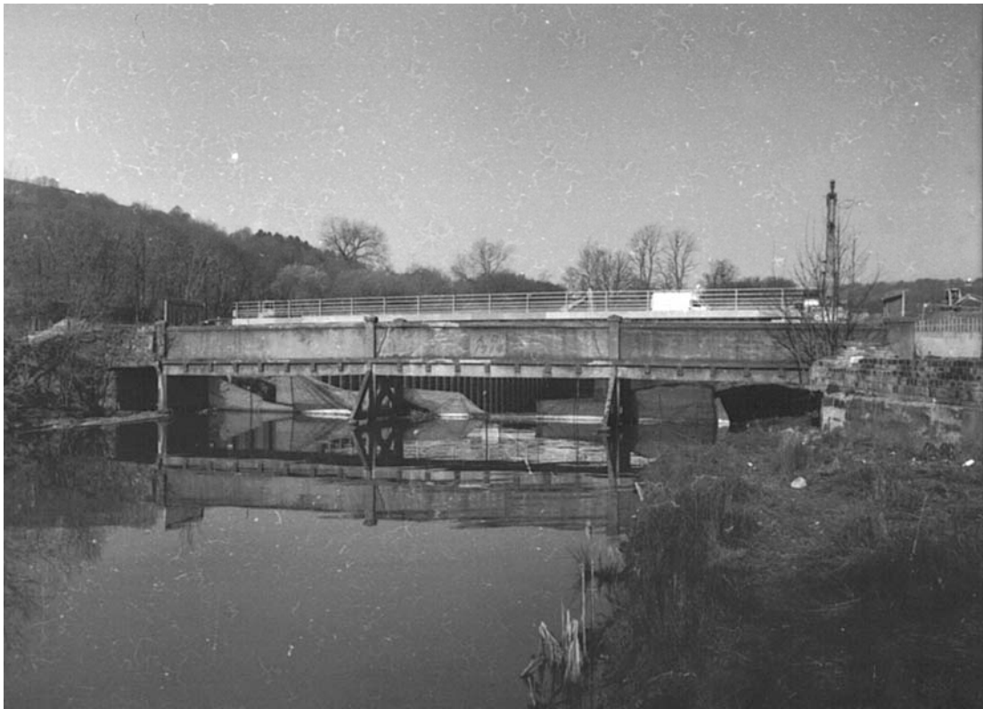
Plate 7: South-east-facing elevation of Sterne Bridge (MF SB01_07)
