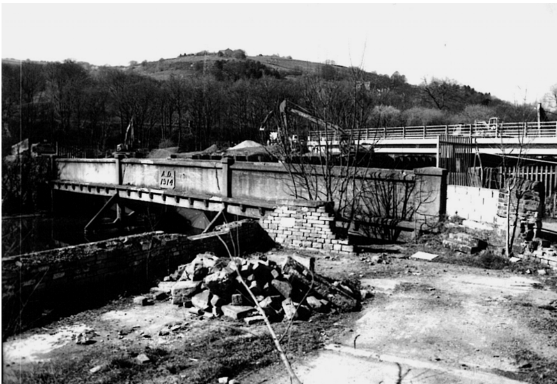
Plate 14: Stepped access (1) and vertical sandstone pillar (2) (MF SB04_09)
