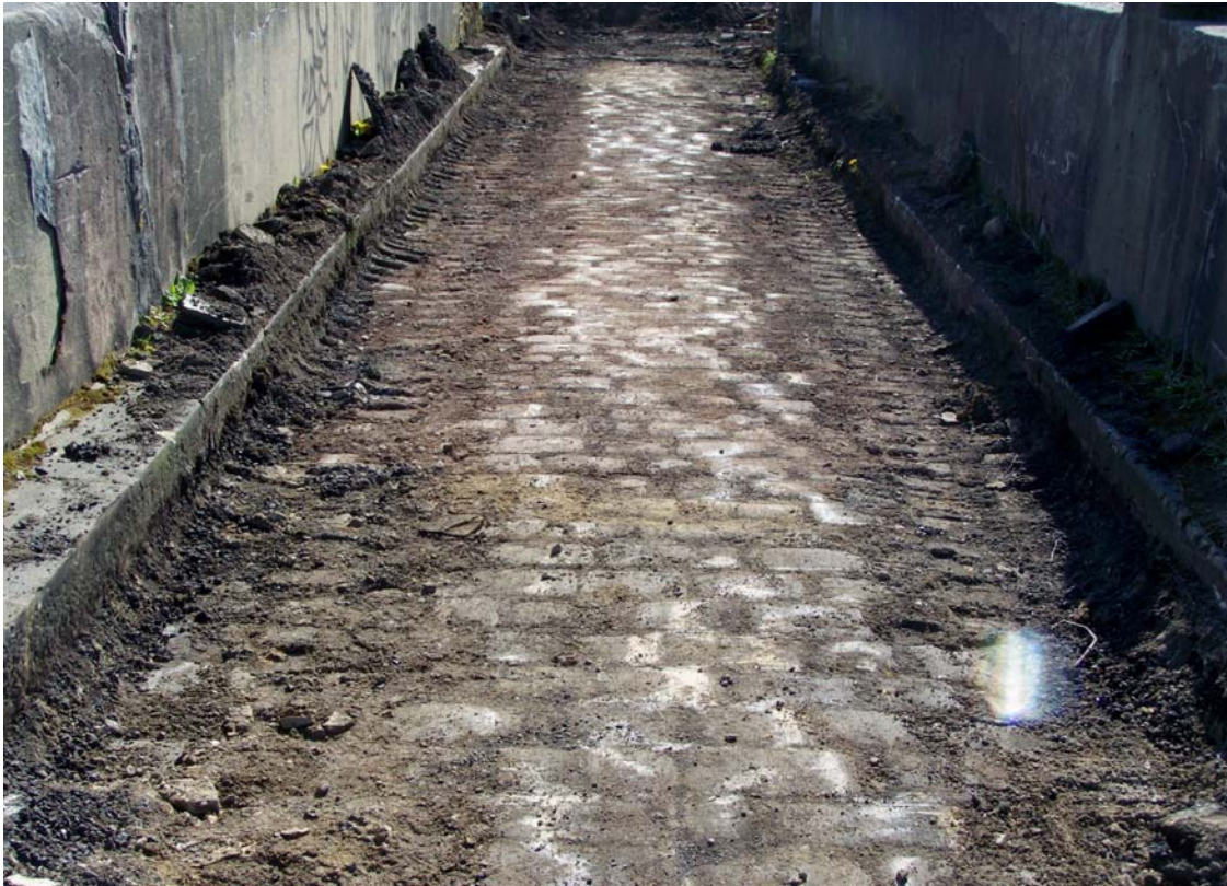
Plate 87: Cobble sett surface (15) exposed during the course of demolition (100_3611.JPG)
