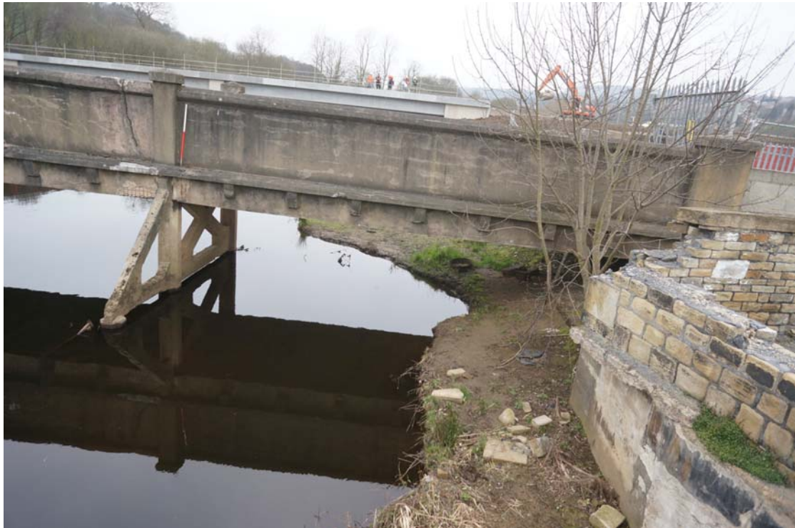
Plate 37: View from the north bank showing south-east-facing elevation and trestle (4a), and cut-water (5) (DSC00486)
