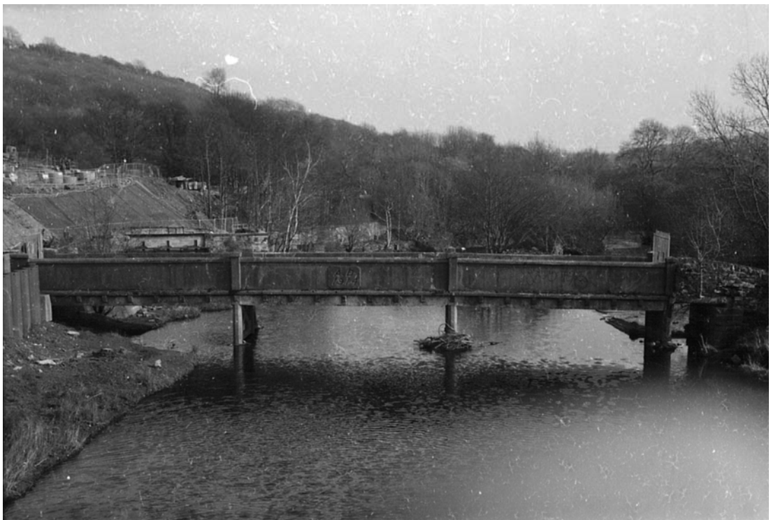
Plate 20: View from the replacement bridge showing the north-west-facing elevation of Sterne Bridge (MF SB07_01)
