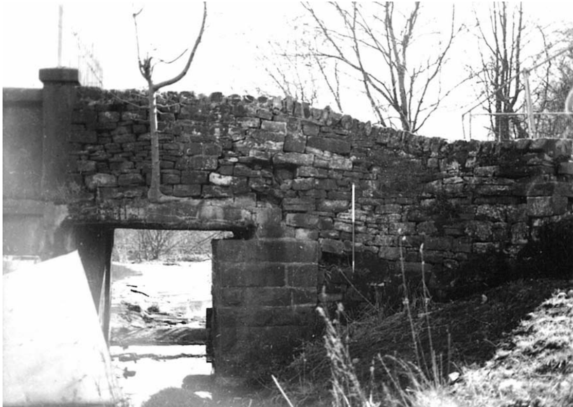
Plate 74: South-western wing wall (11) and sandstone abutment (12) (MF SB06_02)
