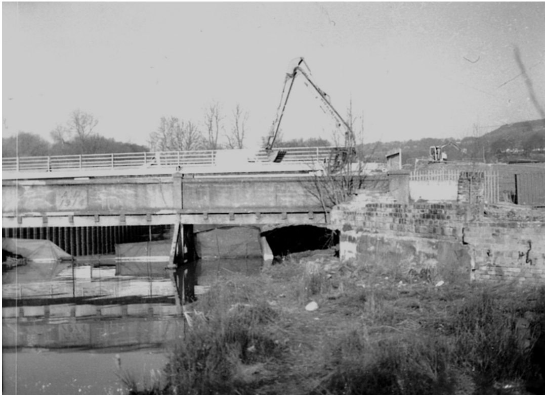
Plate 9: South-east-facing elevation of Sterne Bridge (MF SB01_10)
