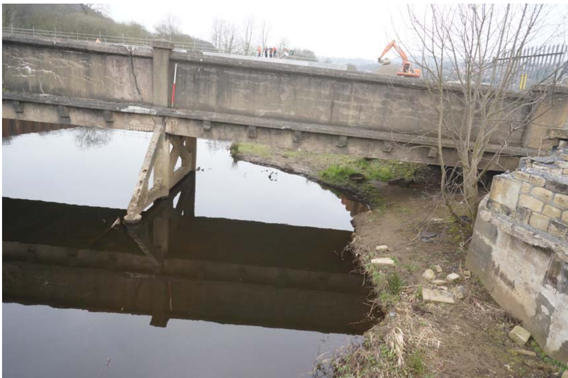
Plate 38: View from the north bank showing south-east-facing elevation and trestle (4a), and cut-water (5) (DSC00487)
