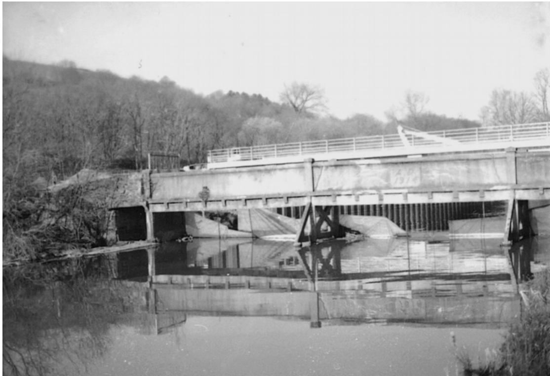
Plate 11: South-east-facing elevation of Sterne Bridge (MF SB01_13)
