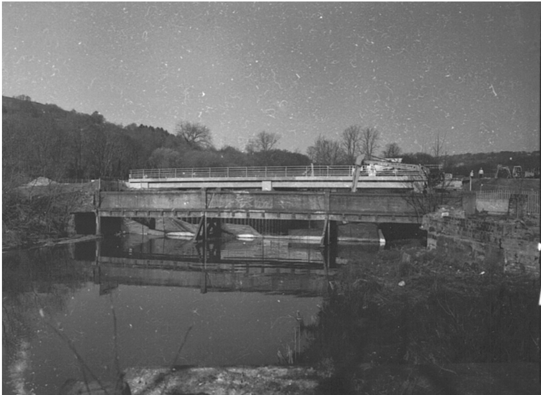
Plate 3: South-east-facing elevation of Sterne Bridge (MF SB01_02)
