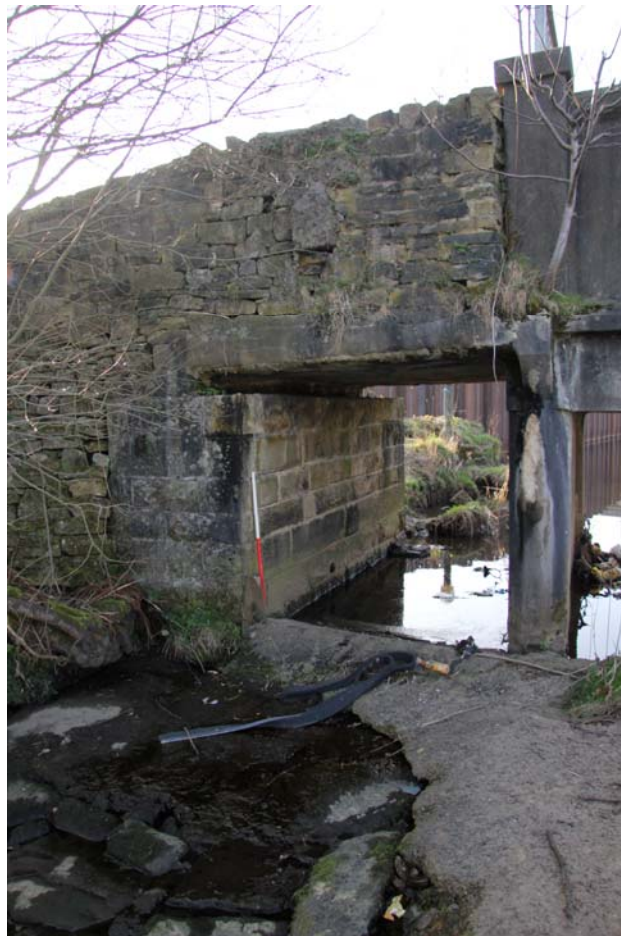
Plate 66: Interface between the south-east wing wall (11), stone abutment (12) and the later concrete parapet wall of bridge (IMG_2407)
