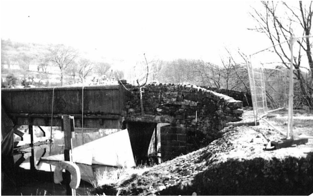
Plate 78: South-western wing wall (11) and sandstone abutment (12) (MF SB06_07)
