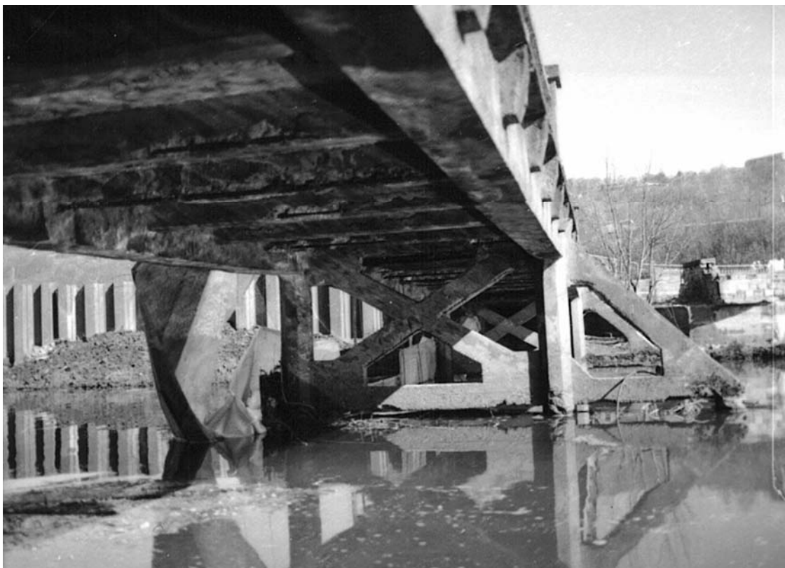
Plate 50: North-facing view showing trestles with diagonal internal bracing ( 4b ) and ( 4a ), and cut-waters ( 5a ) and ( 5 ) (MF SB02_08)
