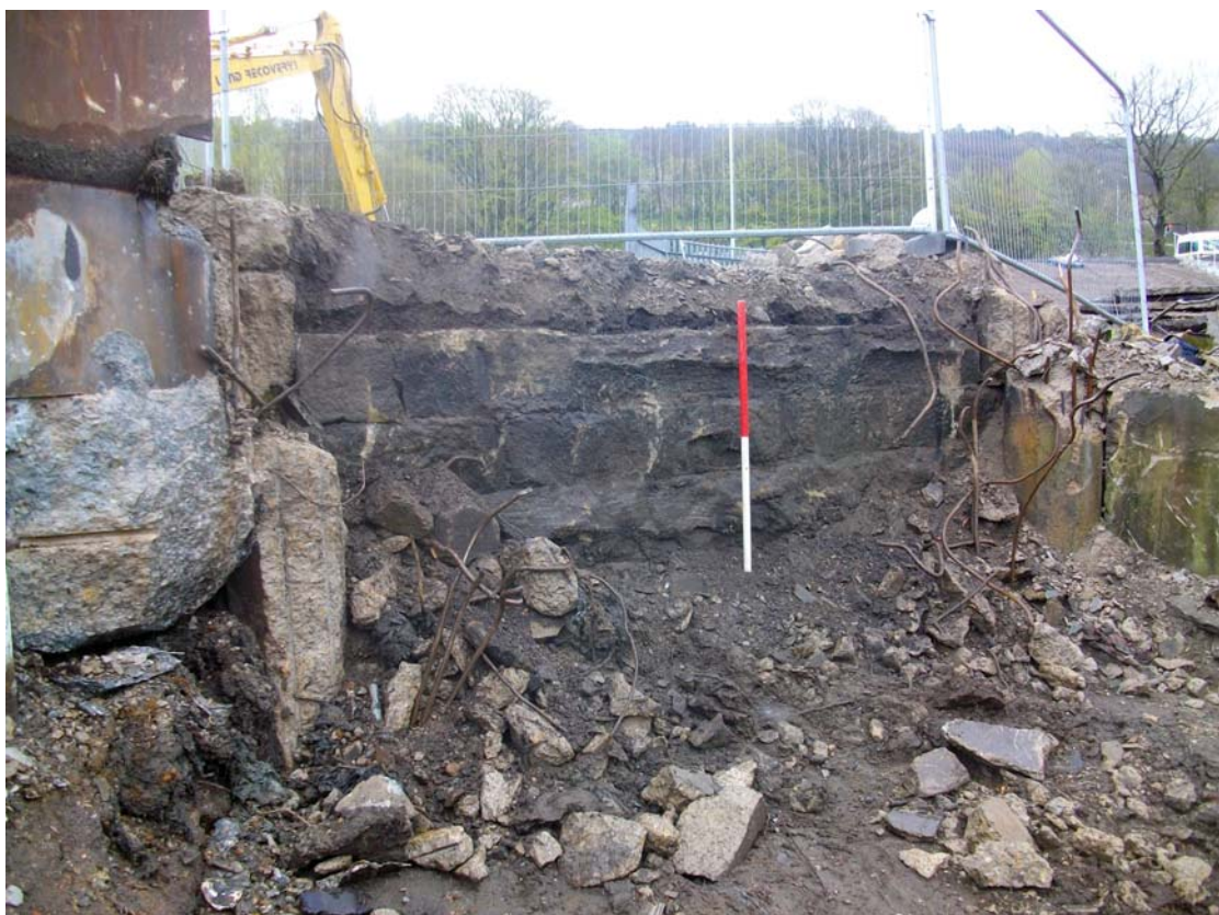
Plate 94: South-east-facing view showing the remains of the northern abutment (3) and octagonal section pillars on the east and west sides (IMG_8743)
