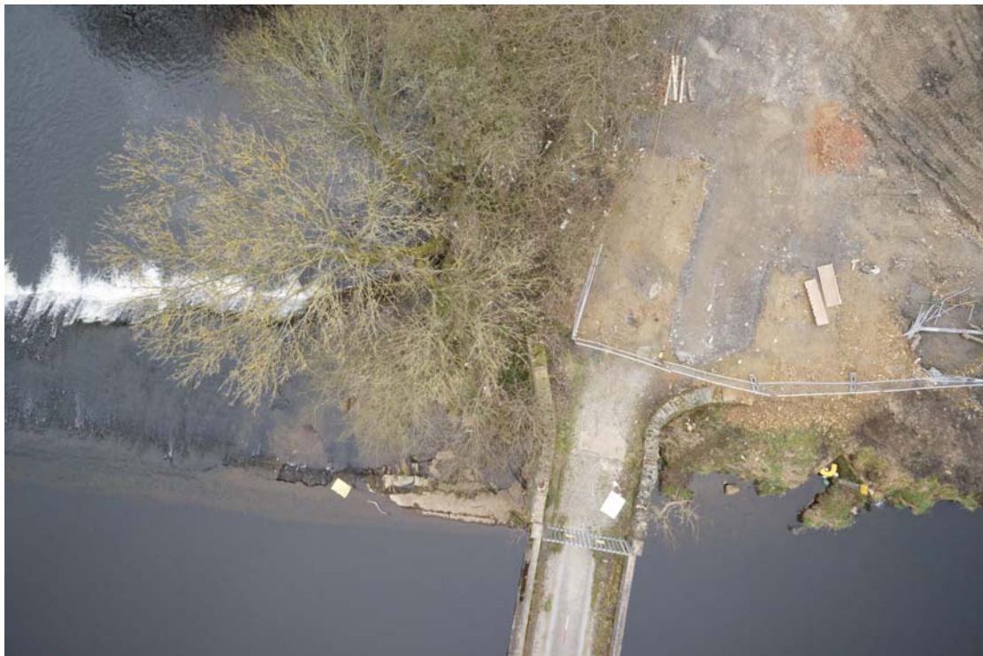
Plate 79: Aerial view showing southern bank and wing walls (11) (DSC00479)
