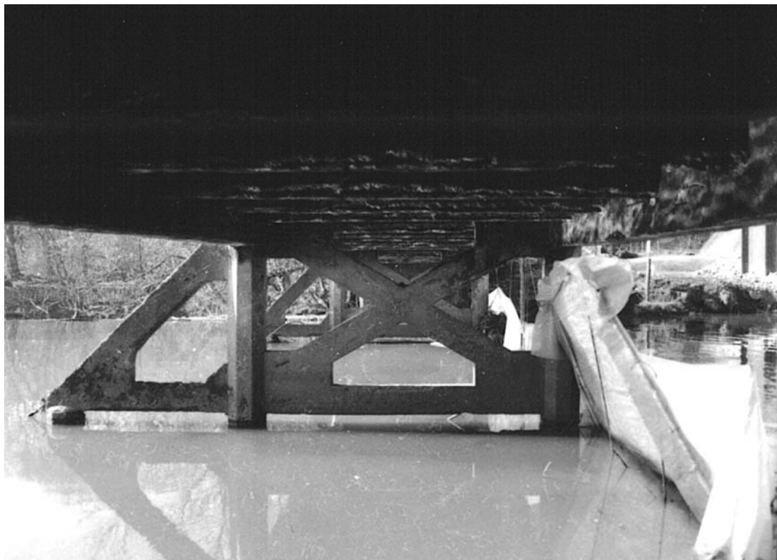
Plate 32: View from the north bank looking south, showing trestles (4a) and (4b) and cut-waters (5) and (5a) (MF SB03_03)
