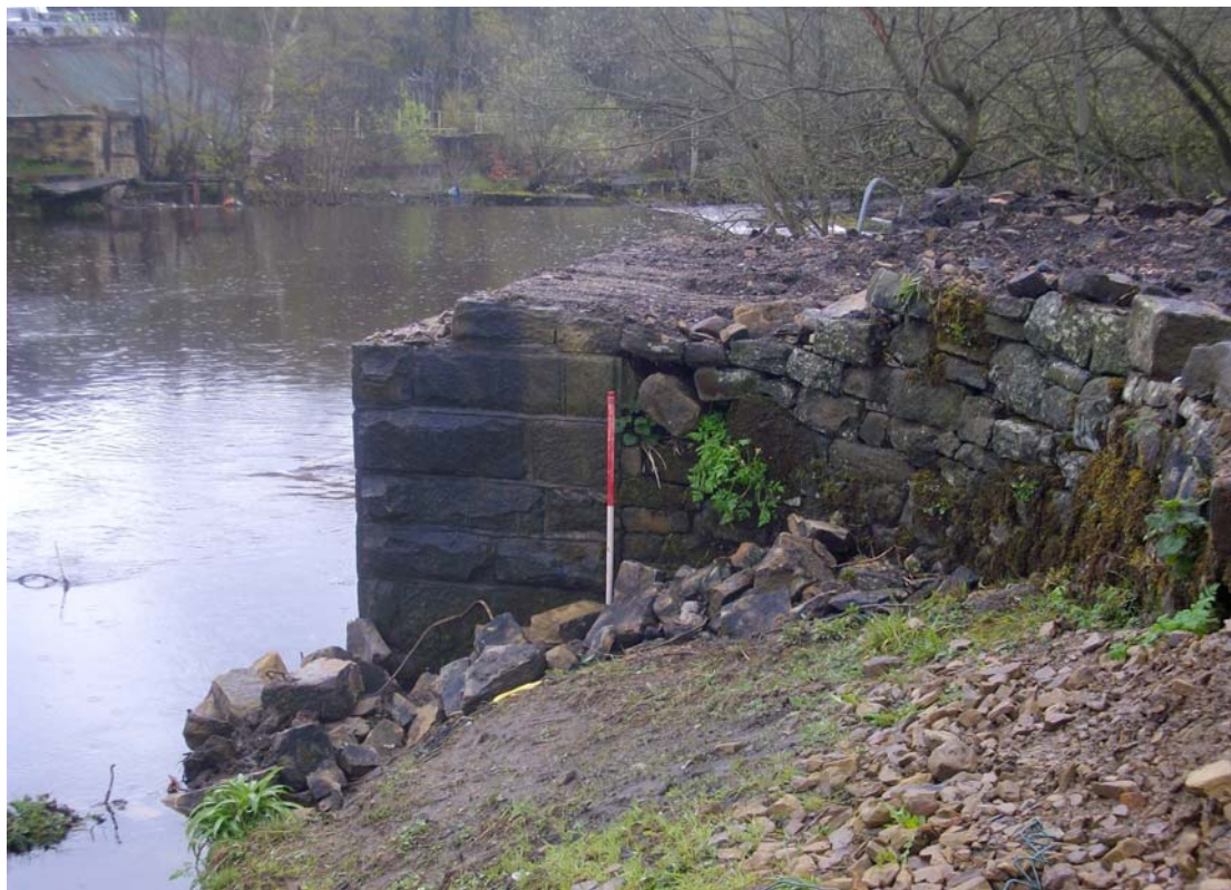
Plate 92: Interface between southern abutment (12) and remains of rubble wing wall (11) after main phase of demolition (IMG_8757)
