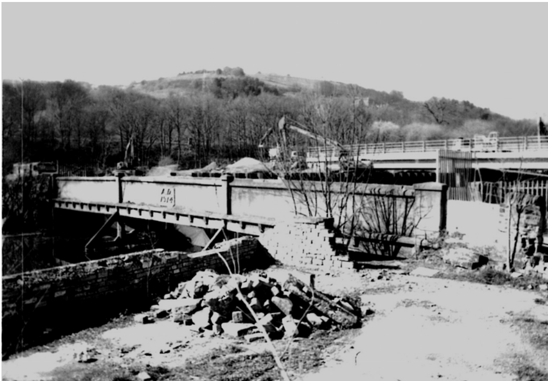
Plate 13: Stepped access (1) and vertical sandstone pillar (2) (MF SB04_08)
