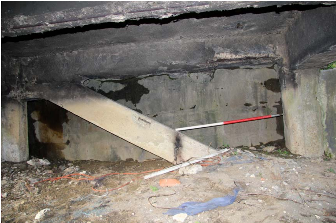
Plate 29: Remainder of earlier bridge barrel (3) behind single trestle (4) (IMG_2442)
