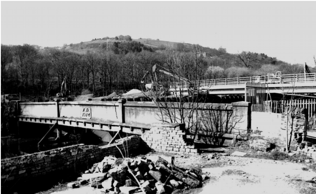
Plate 15: Stepped access (1) and vertical sandstone pillar (2) (MF SB04_15)
