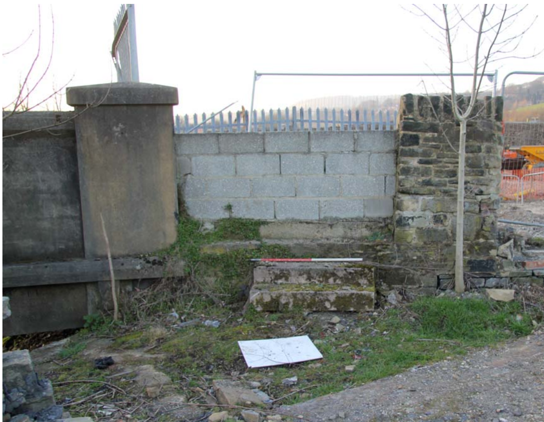
Plate 12: Stepped access (1) (IMG_2445)
