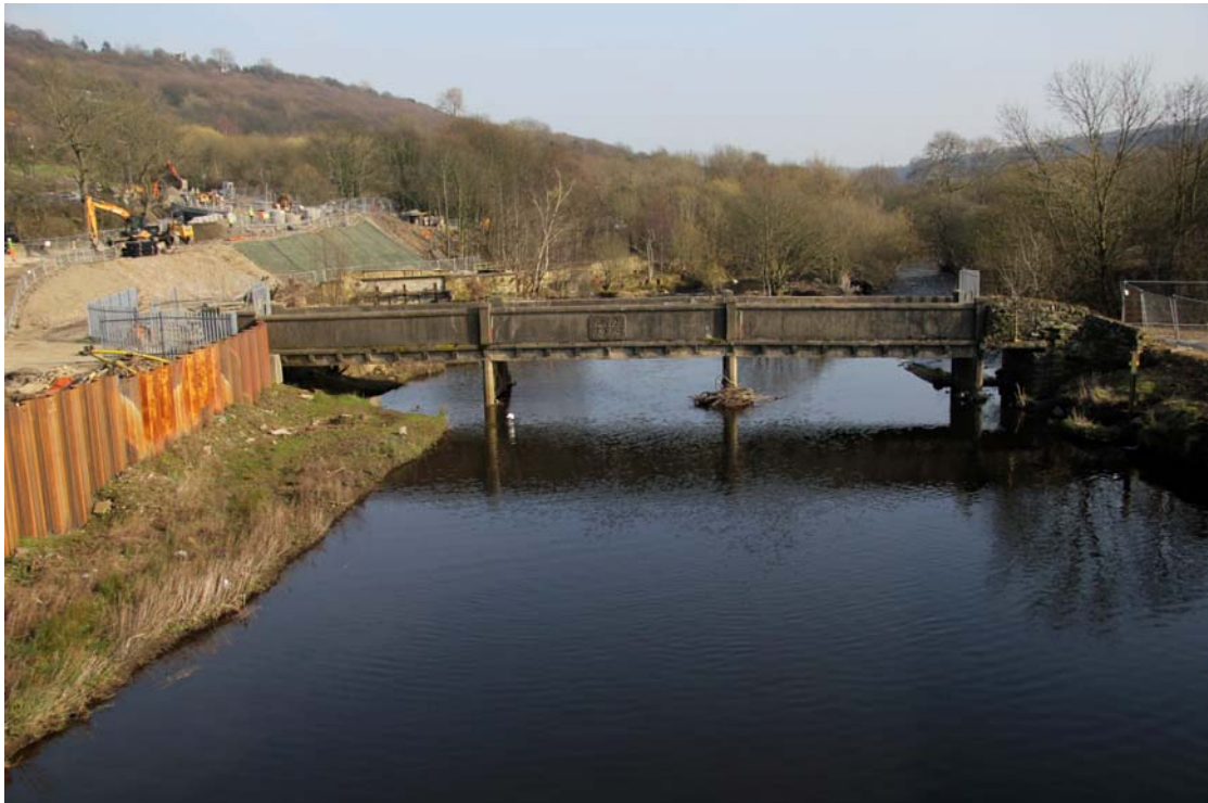
Plate 1: North-west-facing elevation of Sterne Bridge (IMG_2383)
