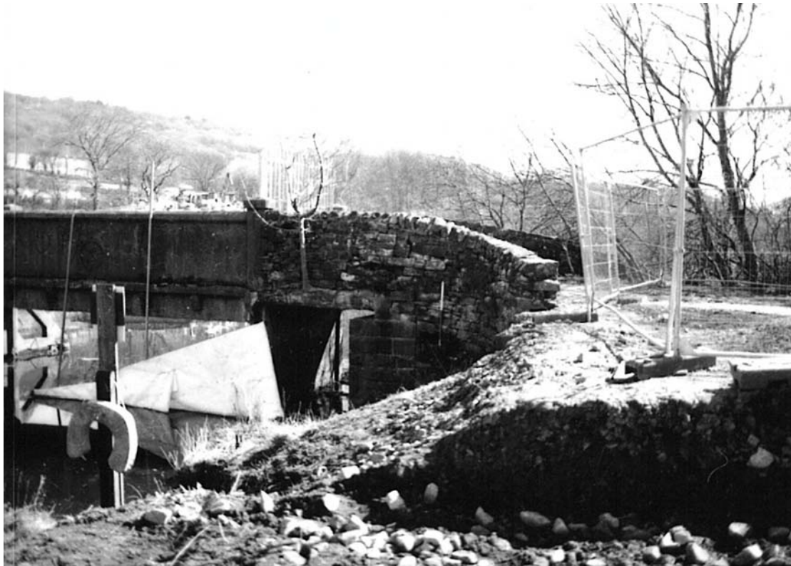
Plate 76: South-western wing wall (11) and sandstone abutment (12) (MF SB06_05)
