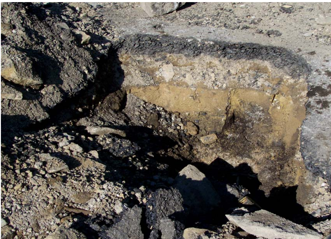
Plate 88: Bedding and made-ground layers between the cobble setts (15) and modern surface (14) on the bridge deck (100_3619. JPG)
