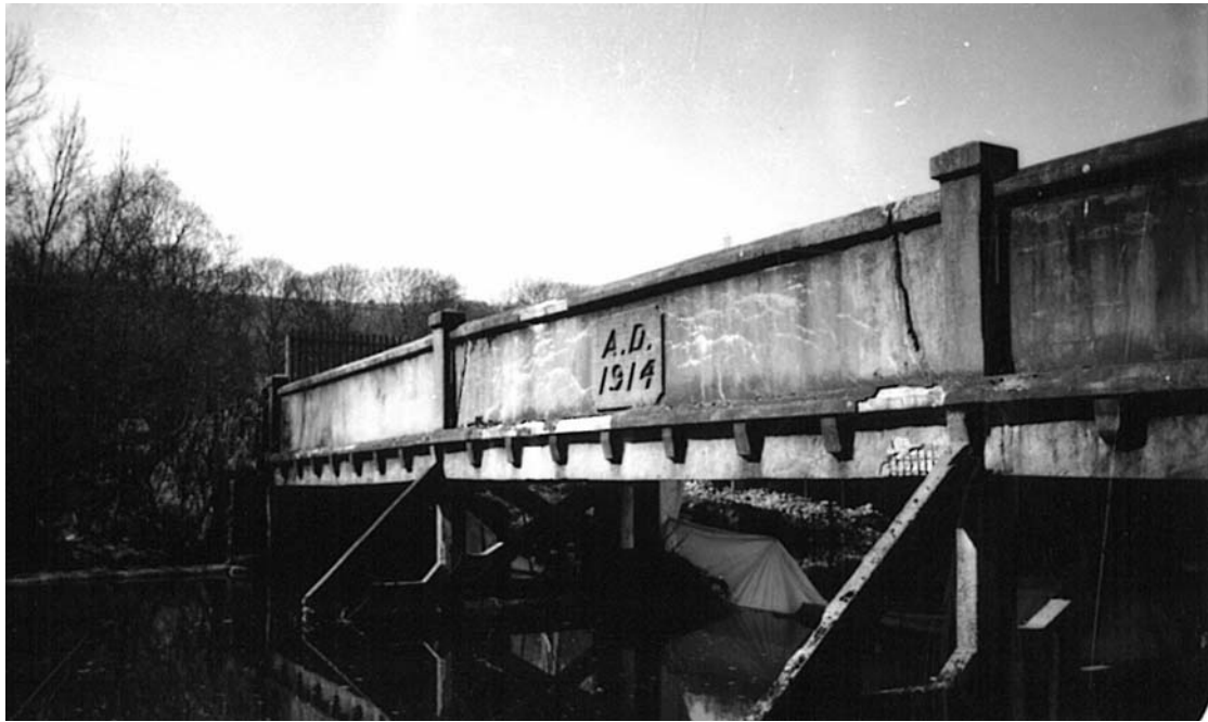
Plate 65: South-facing view showing parapet and parapet sill (10) over cross beams (8) with vertical pillars (9a-9c) and date stone (13) (MF SB06_15)
