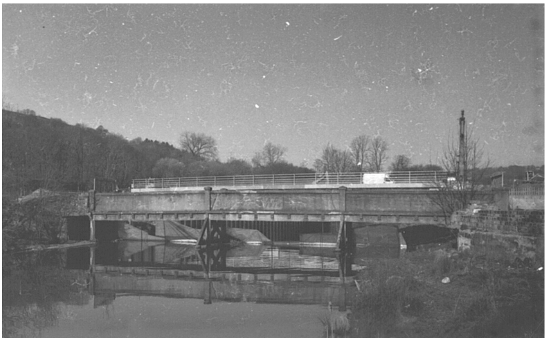
Plate 8: South-east-facing elevation of Sterne Bridge (MF SB01_08)
