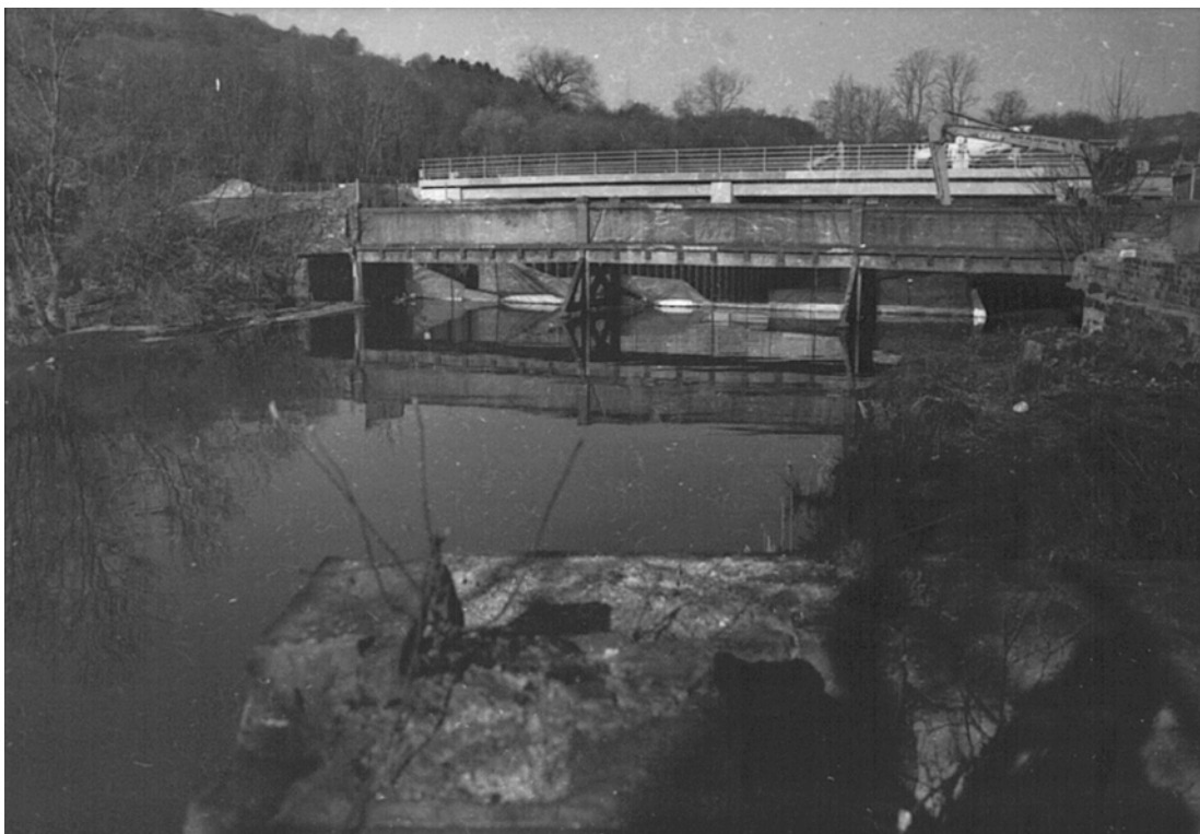
Plate 2: South-east-facing elevation of Sterne Bridge (MF SB01_01)
