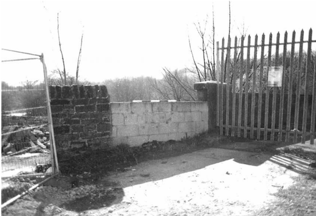
Plate 27: Blocked stepped access (1) and surviving section of eastern wing wall (2) (MF SB05_10)
