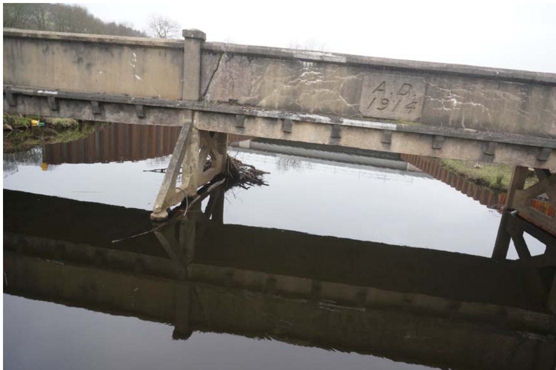
Plate 42: South-east-facing bridge elevation and trestle (4b); also showing cut-water (5a) (DSC00498)
