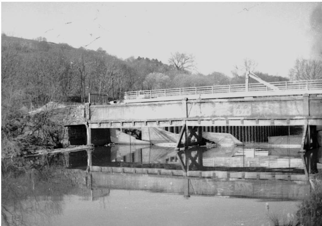
Plate 10: South-east-facing elevation of Sterne Bridge (MF SB01_12)
