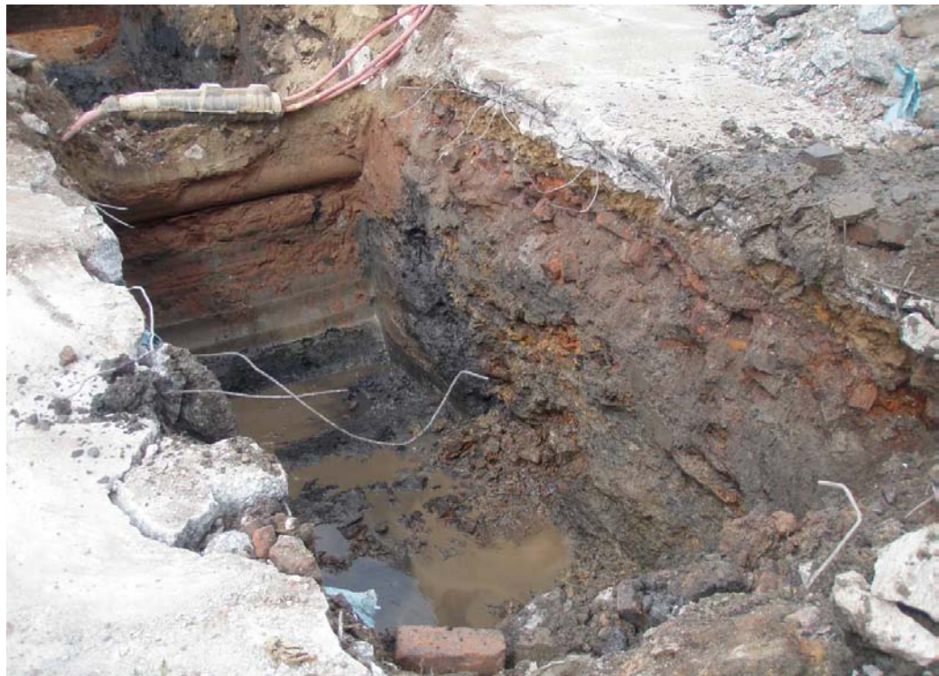
Plate 2: View across Trench 8 looking south-east, showing modern deposits and interventions in the former canal
