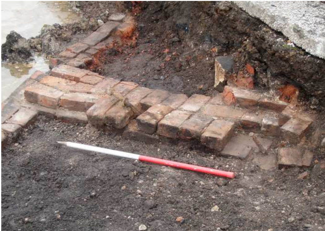
Plate 39: The remains of restraining bars set in wall 06 , with wall 07 to the rear
