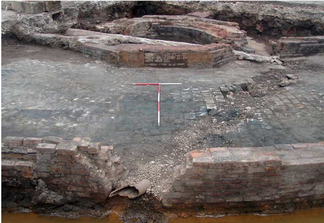
Plate 32: Drain 2010 continuing eastwards from the foundations of the chimney stack
