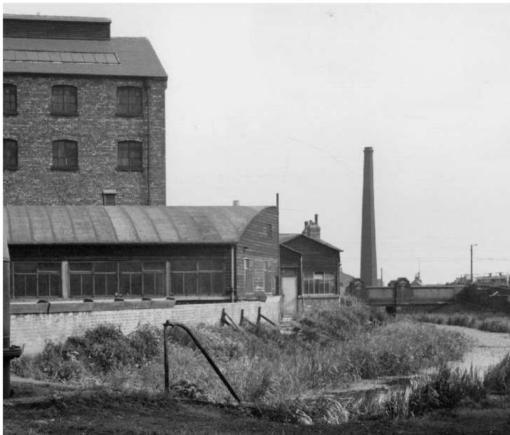
Plate 52: View along the disused Clayton Arm in 1960, showing premises occupied by the Clayton Aniline Company, and the chimney of the Clayton Chemical Works in the background
