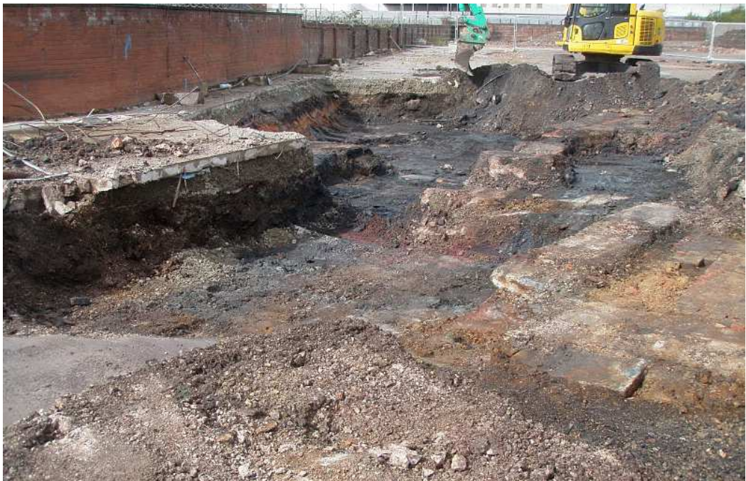
Plate 26: Excavation in the western part of Area A encountered significant ground contamination
