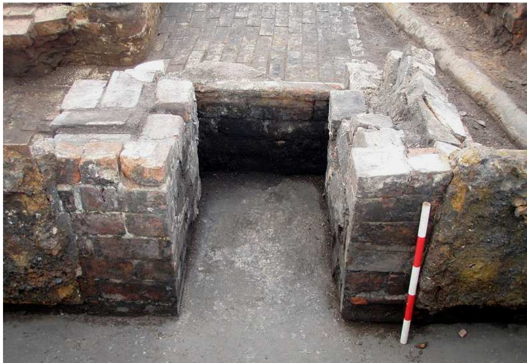
Plate 17: Housing for the blow-down valve in the western boiler bay (1071)
