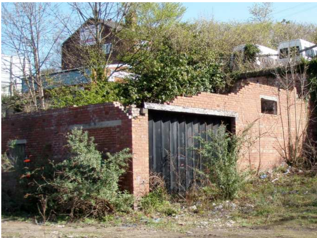
Plate 10: Building 102, looking north-east
