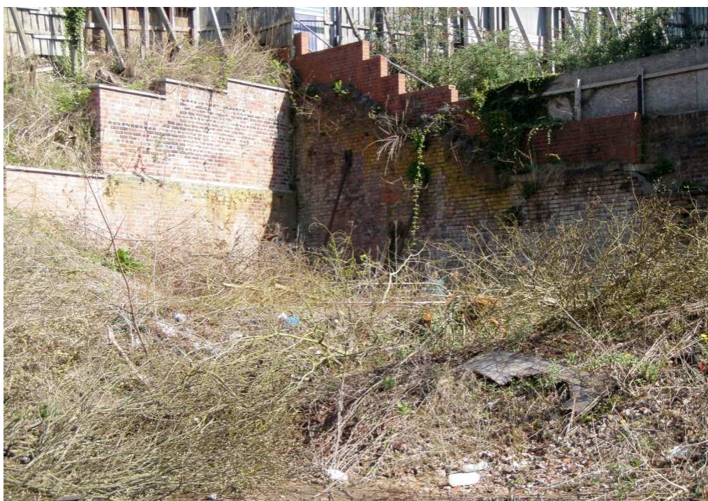
Plate 8: Wall 101 , looking north
