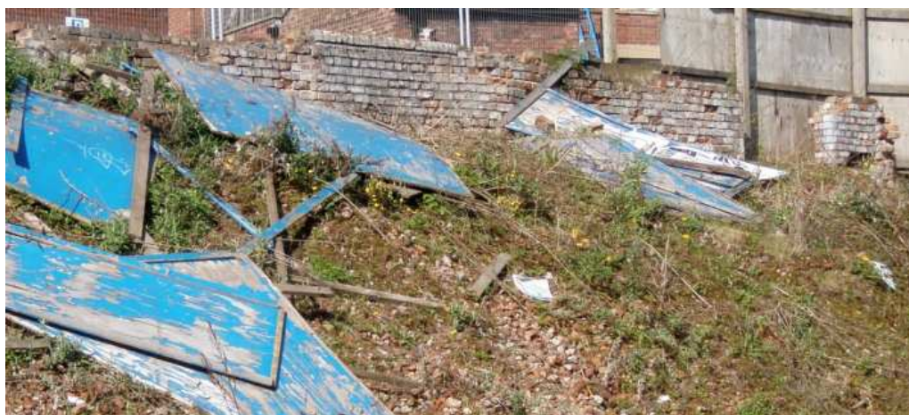
Plate 17: Wall 111, looking north-west
