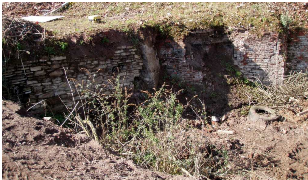
Plate 19: Wall 113 , looking south-west
