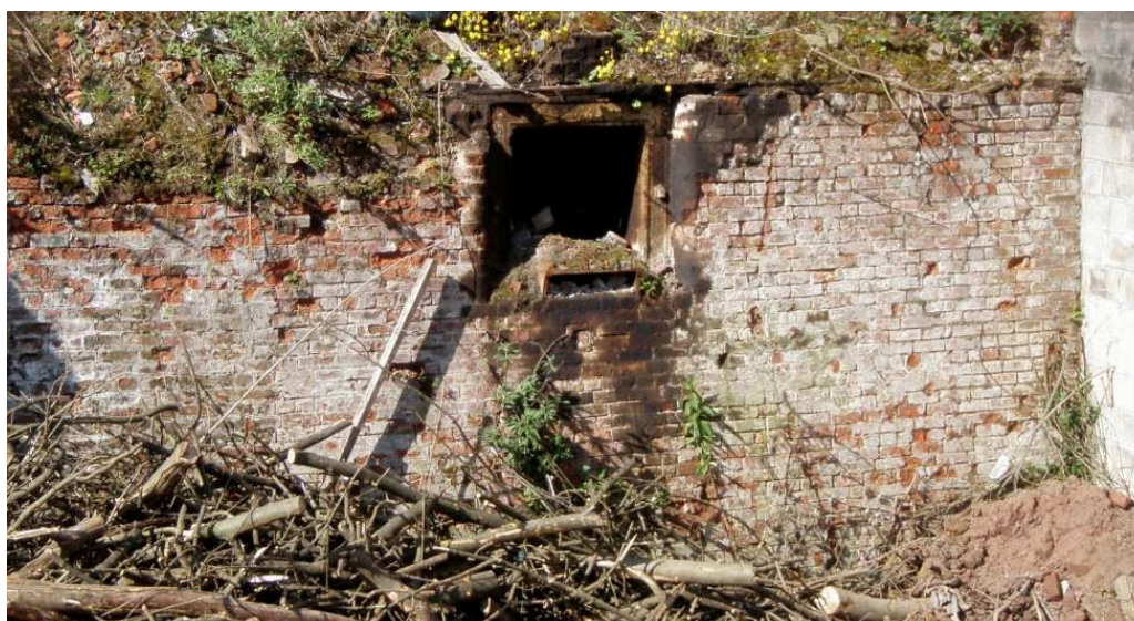
Plate 18: Wall 112, looking north-west
