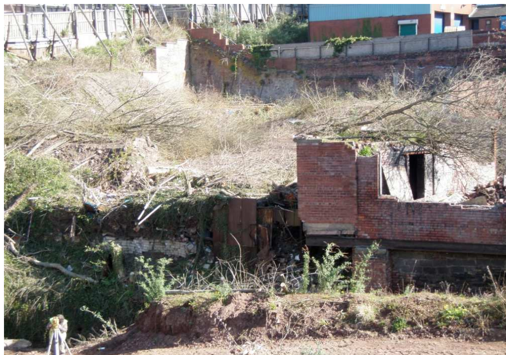
Plate 13: Wall 107, looking north-east
