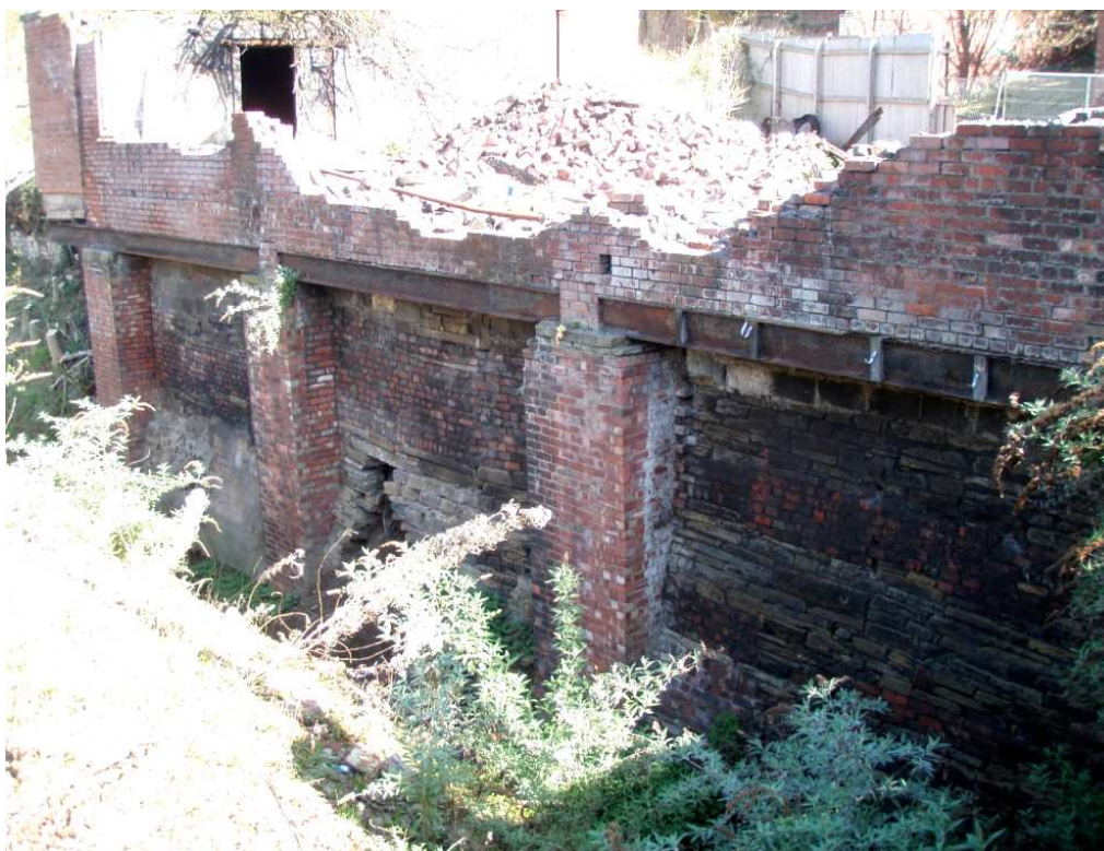
Plate 14: Culvert 108 , looking north-east
