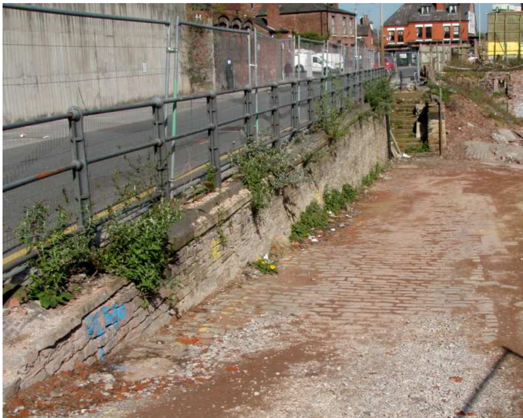
Plate 21: Wall 114 looking north
