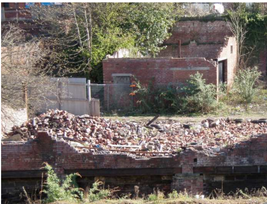
Plate 12: Building 106, looking east
