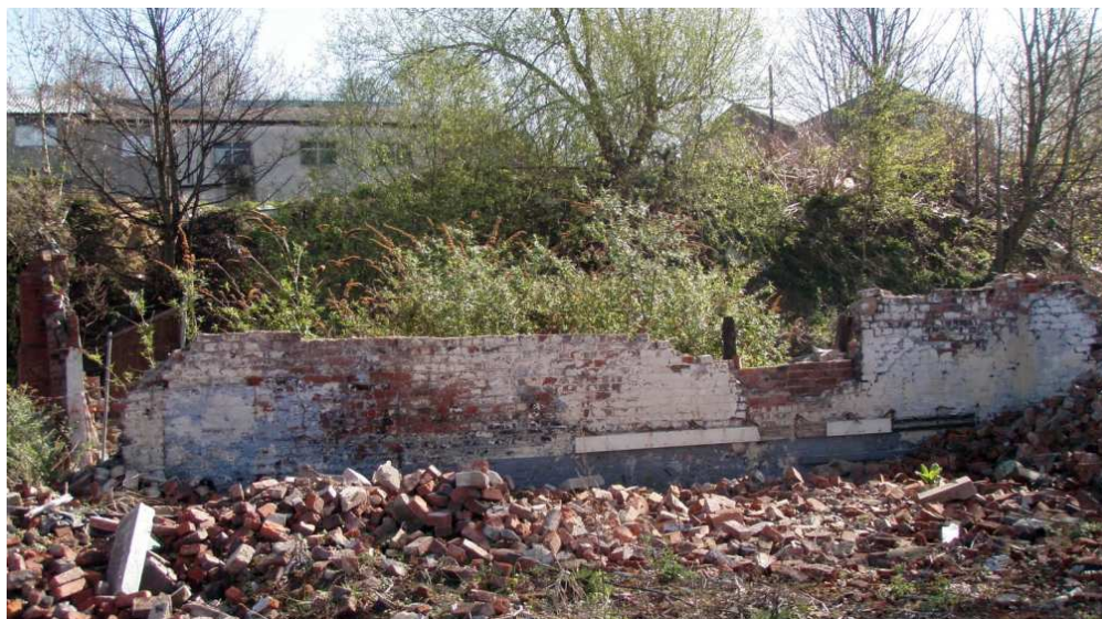
Plate 11: Building 105, looking east
