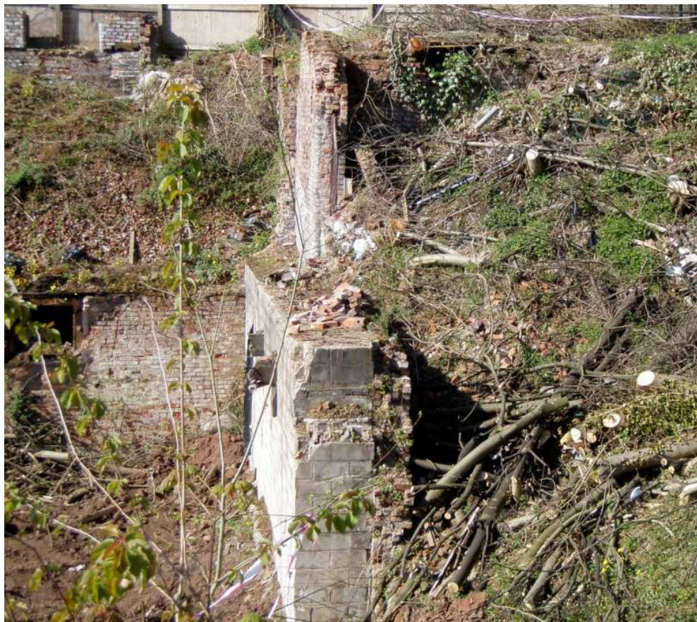
Plate 16: Wall 110, looking south-east
