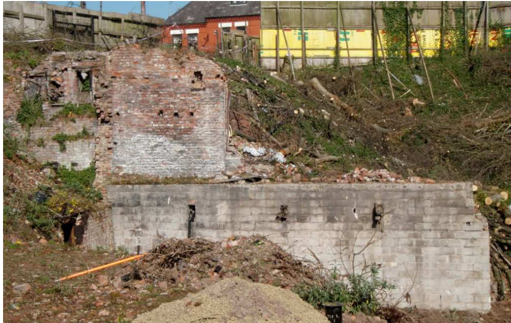
Plate 15: Wall 109, looking north-east
