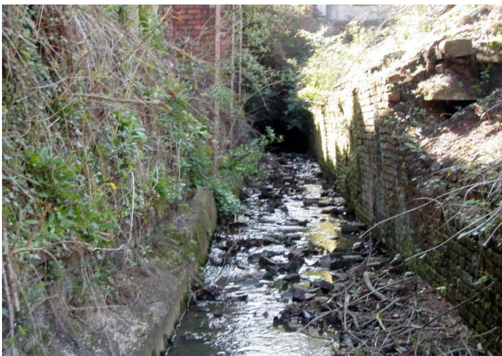
Plate 22: The open culvert for the Hempshaw Brook as it flows across the study area
