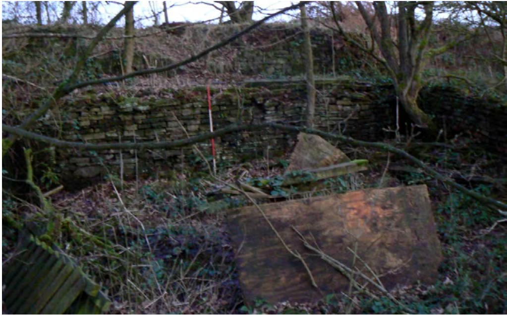
Plate 47: The south-eastern end of the Stentering Room (48A)
