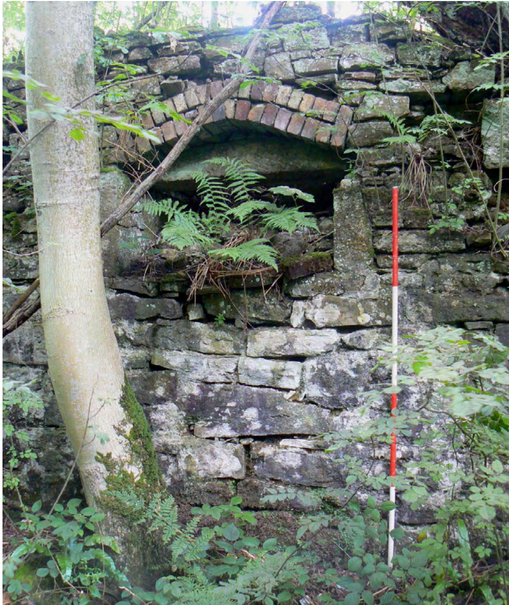
Plate 33: A remodelled aperture in the north-western wall of Room 22
