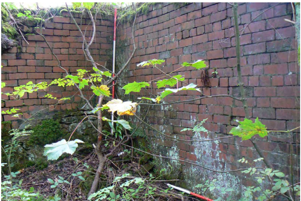
Plate 35: The extant remains of Room 22B
