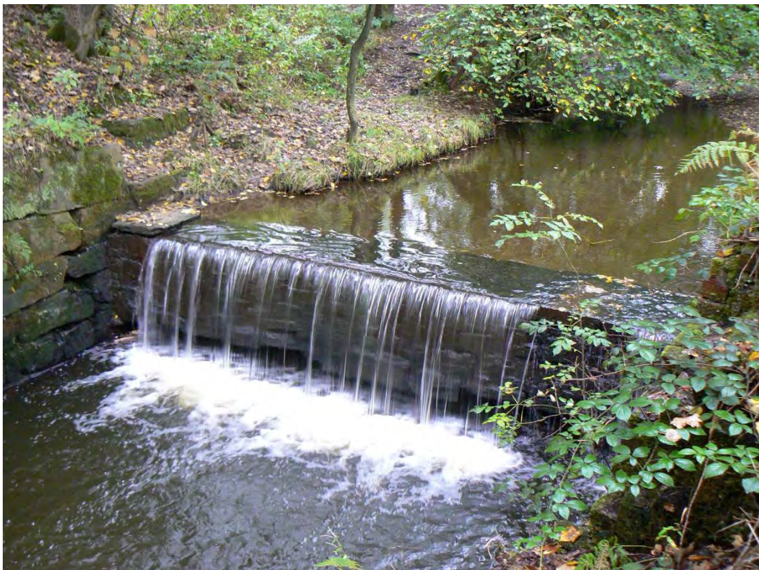
Plate 58: Weir No 1, looking south
