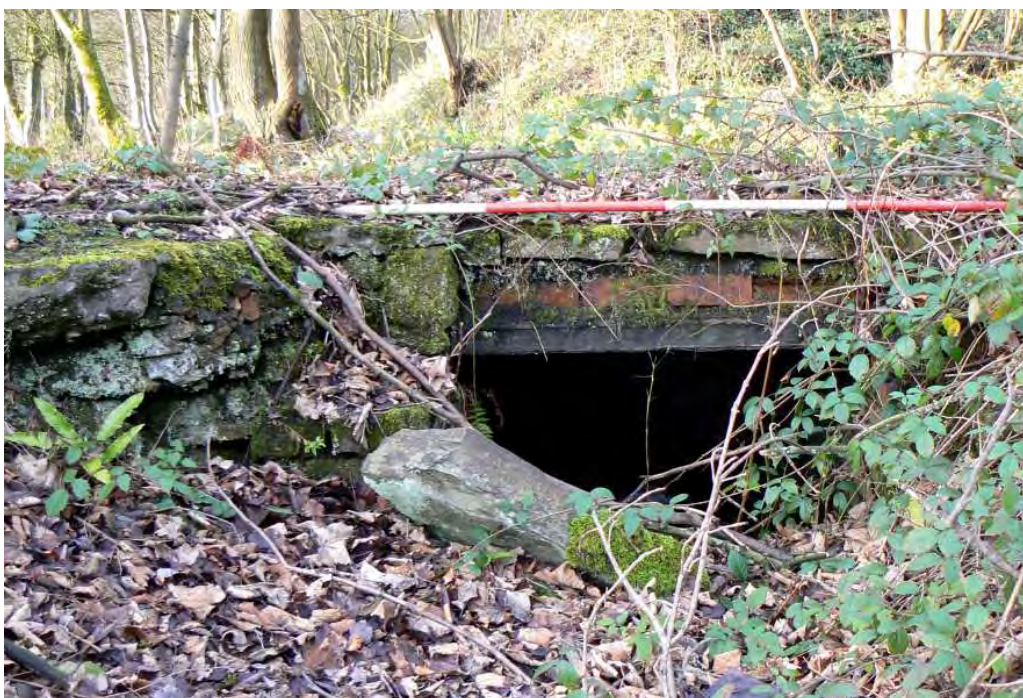
Plate 18: Remains of the south wall of the Gas Retort House, and access to the basement
