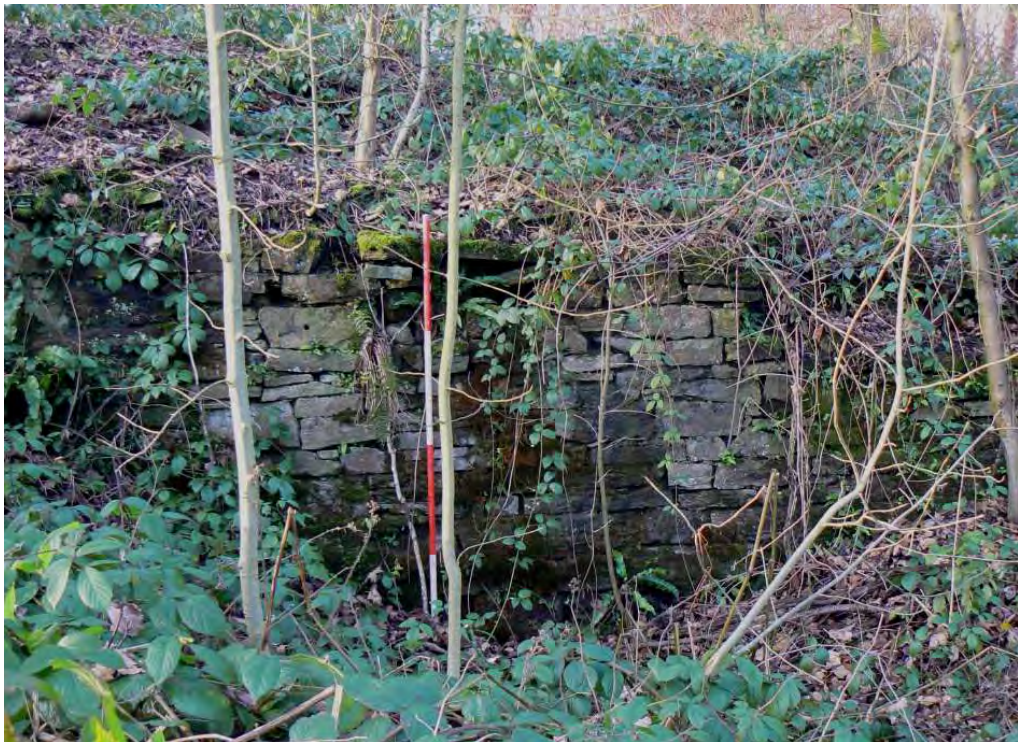
Plate 21: The internal elevation of the north wall of the Smithy
