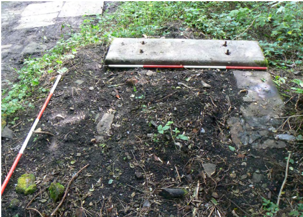
Plate 30: The probable foundation bed for a machine or small steam engine in Room 19
