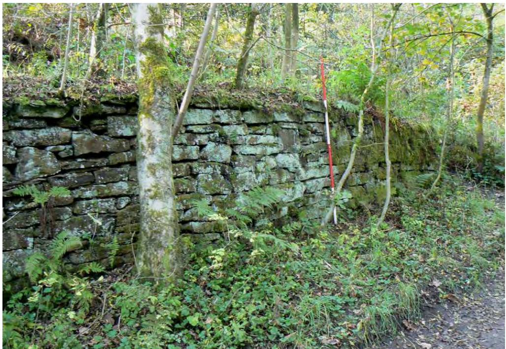
Plate 70: The retaining wall along the western side of Mill Lane at the southern end of the site
