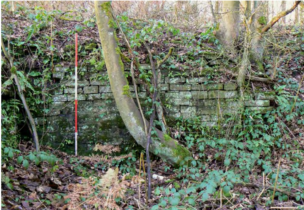
Plate 22: The internal elevation of the north wall of the Mechanics' and Joiners' Shop
