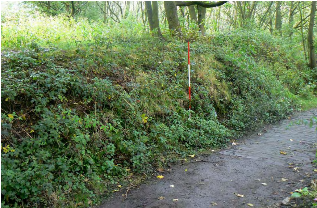
Plate 53: The raised bank of the infilled Lodge No 5, looking north-east
