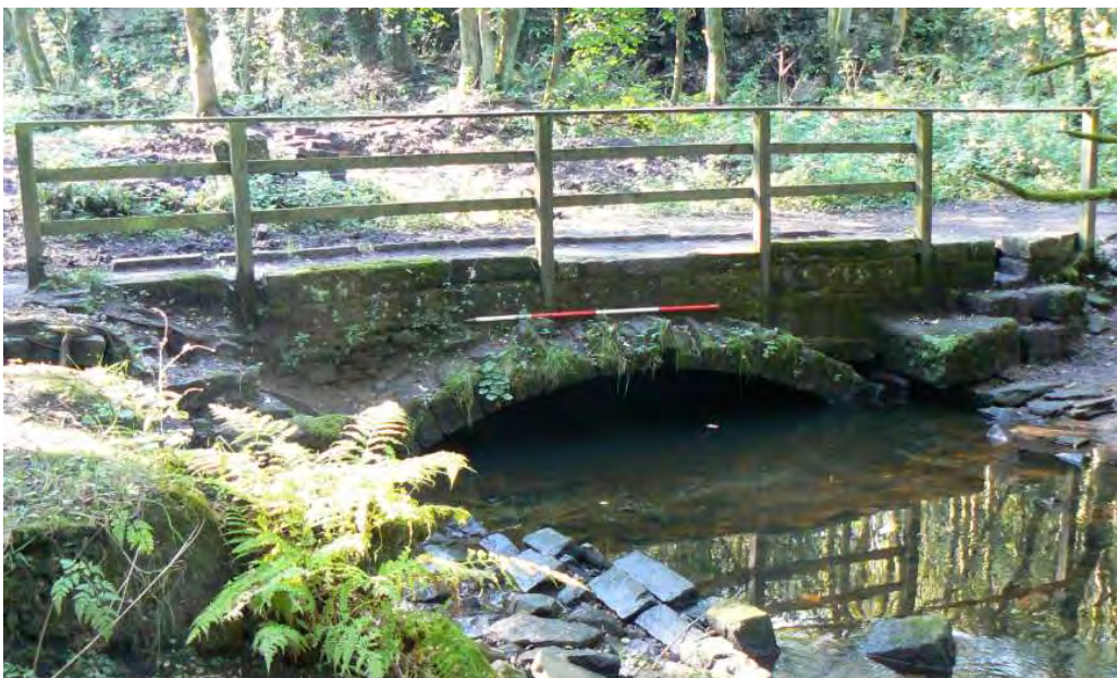
Plate 61: The eastern (downstream) end of the culvert
