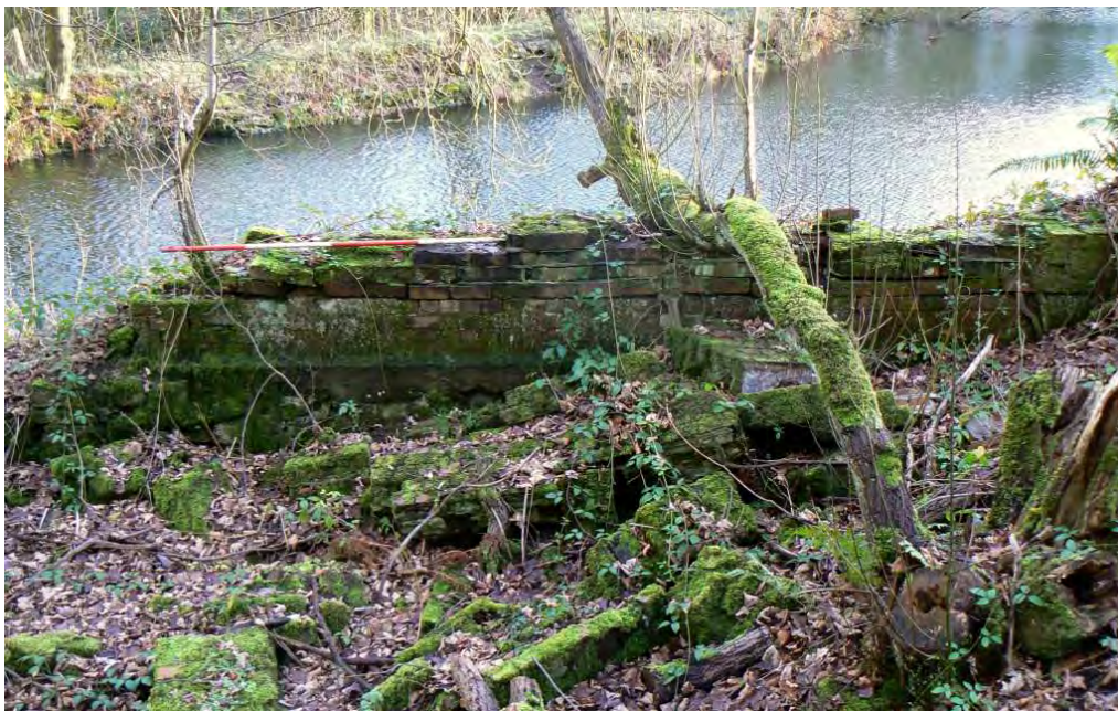
Plate 23: The southern wall of the Copper Roller Store
