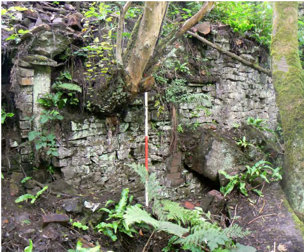
Plate 29: The western wall of Building 16/19
