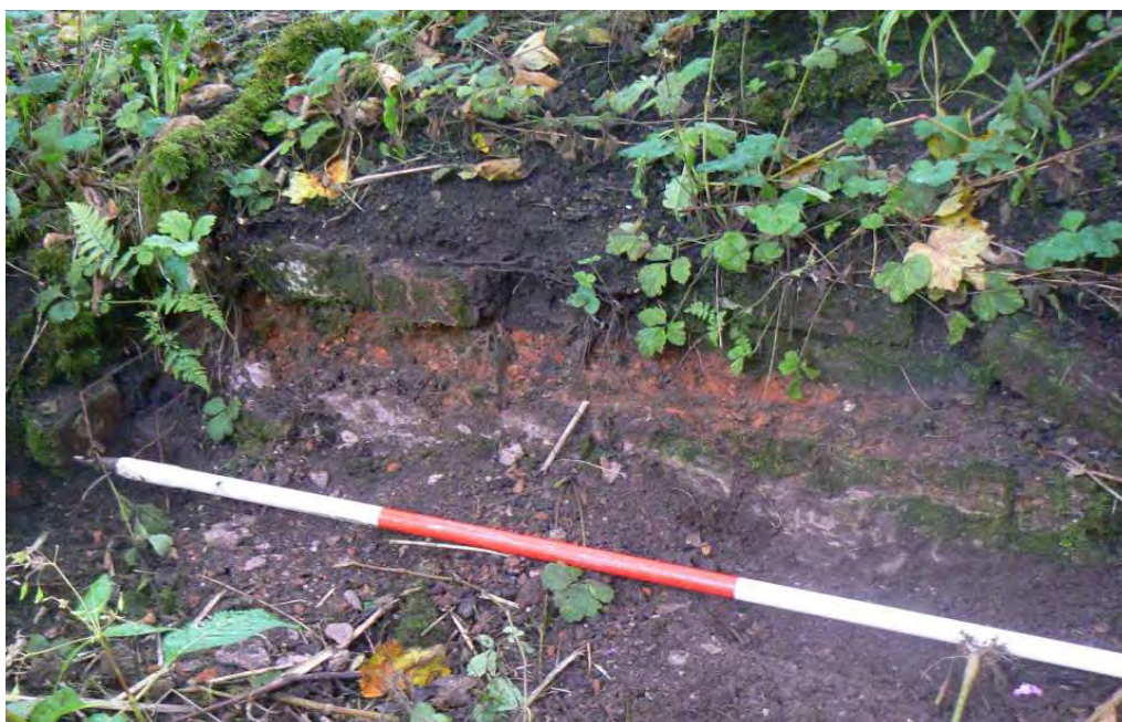
Plate 49: Foundations of the cottages on Mill Street, looking north-west
