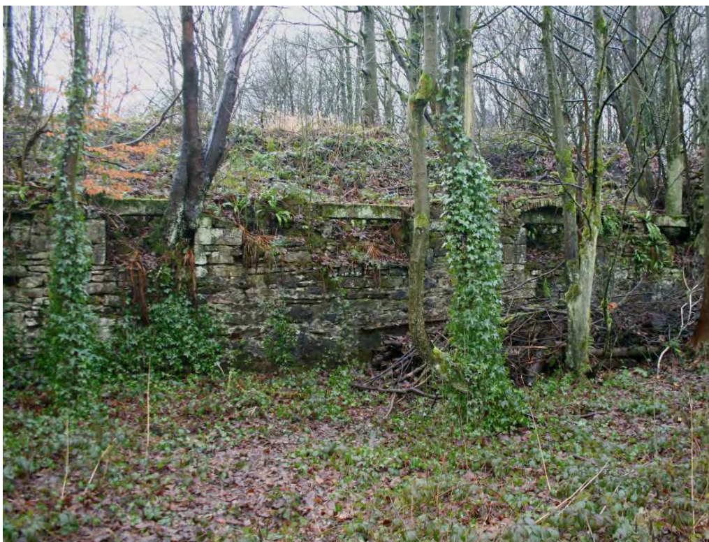
Plate 32: The north-western wall of Room 22
