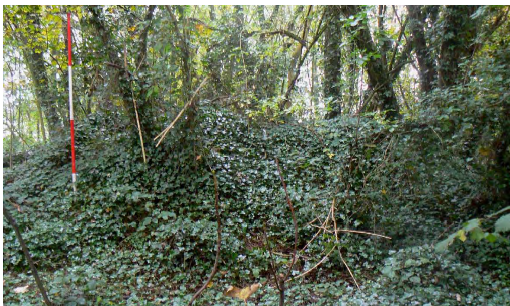
Plate 20: Probable demolition rubble on the site of the gasometer
