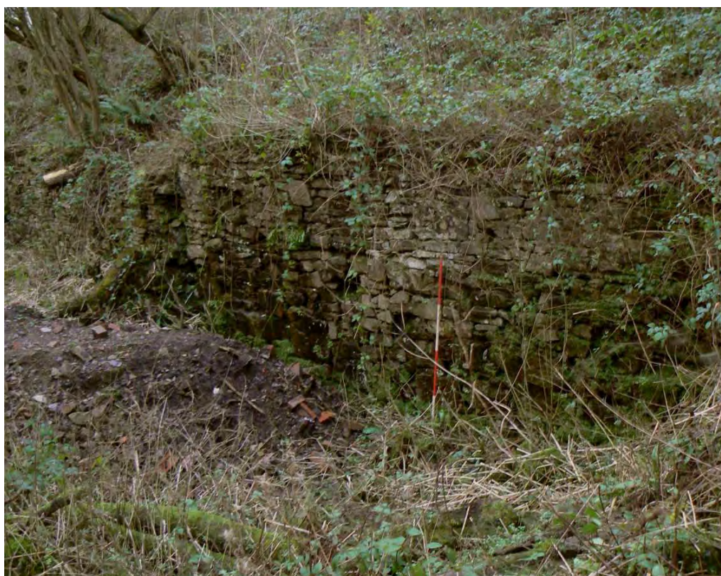
Plate 46: A section of the north wall of Kier House (44), looking north-east
