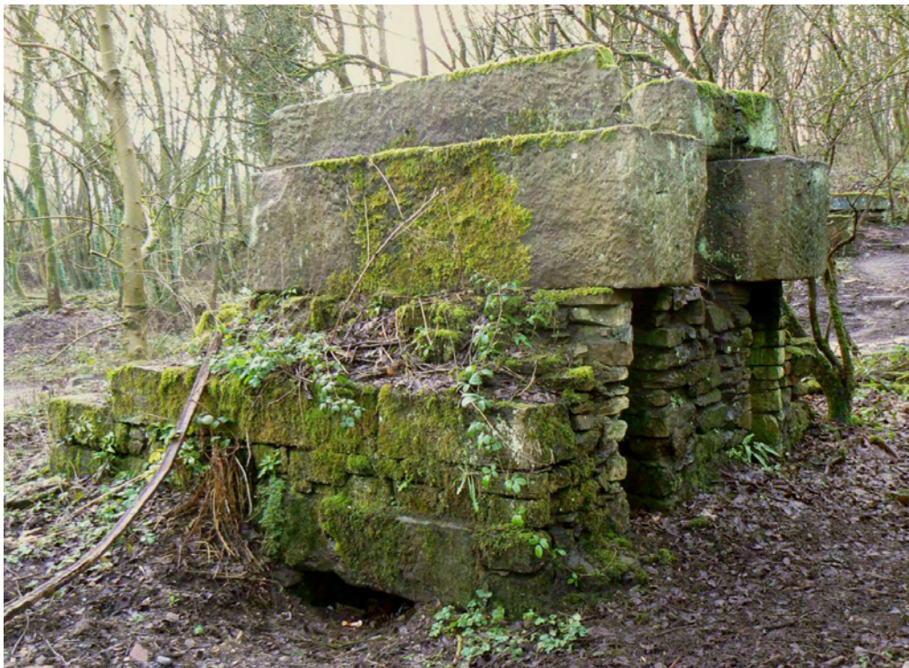
Plate 43: The remains of the foundation bed for a steam engine in Room 36
