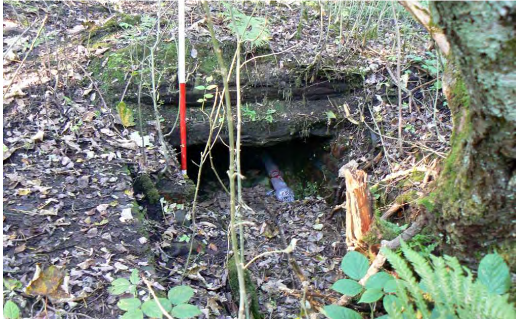
Plate 64: Remains of the culvert leading to the filter beds
