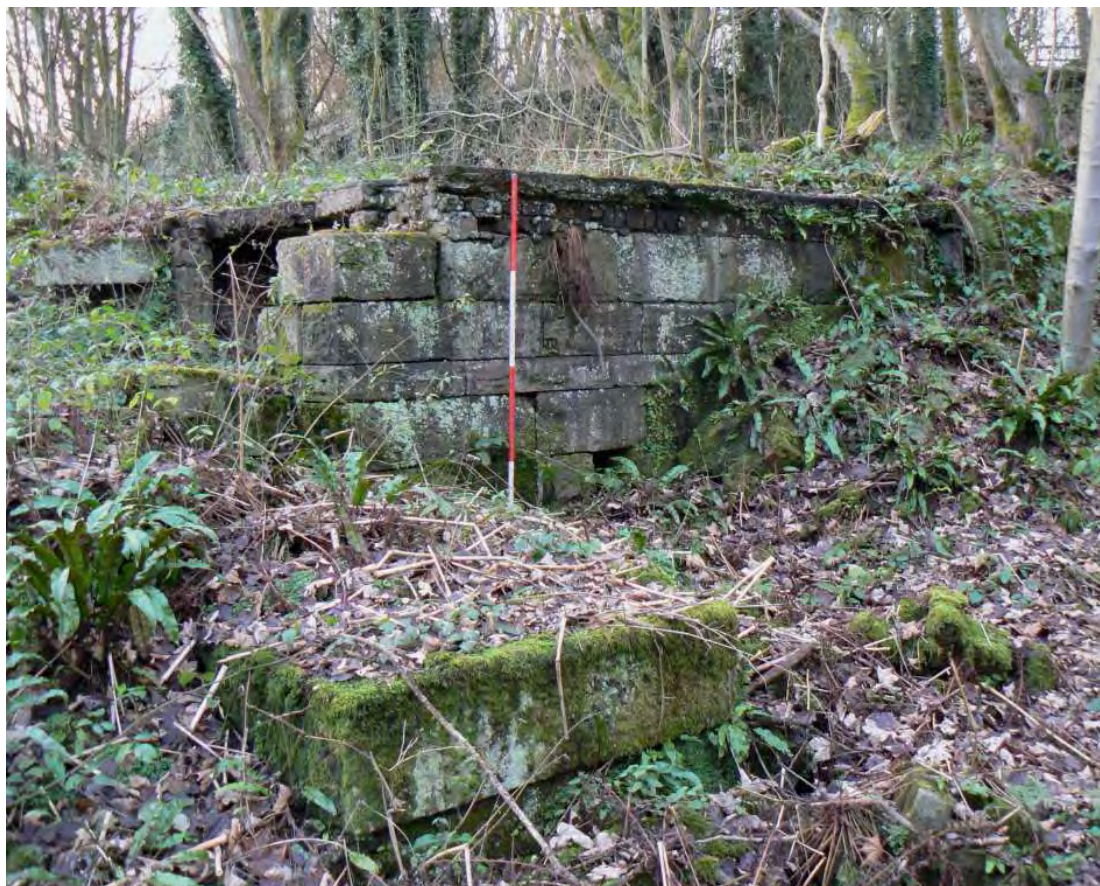
Plate 28: Substantial remains of Room 15
