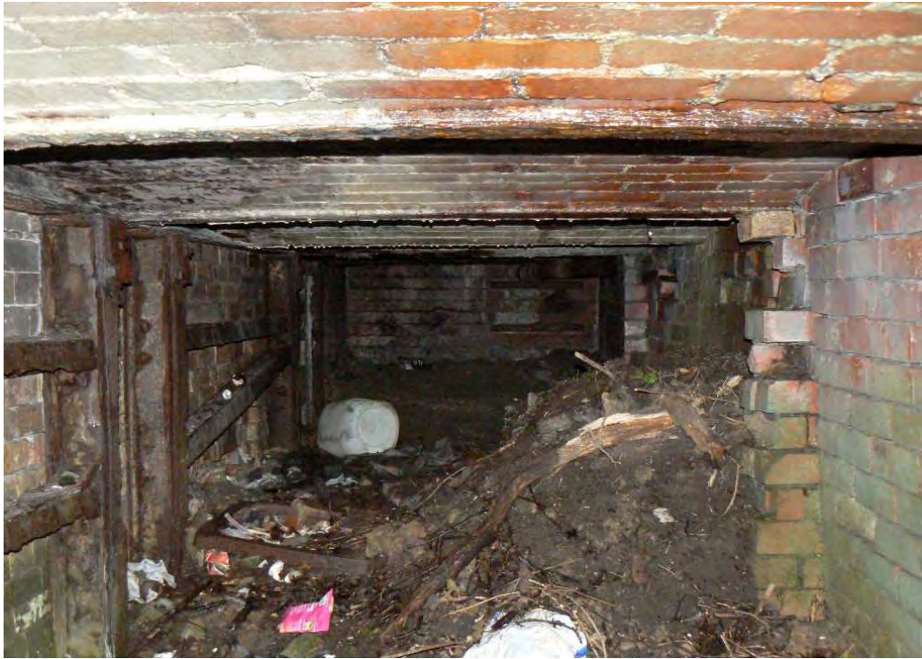
Plate 19: The Gas Retort House basement
