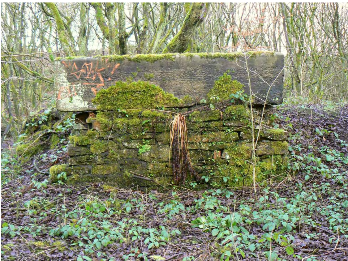
Plate 40: Western stone foundation block for a steam engine in the New Print Shop
