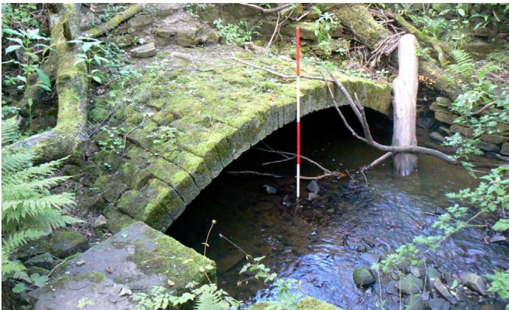
Plate 60: The western (upstream) end of the culvert
