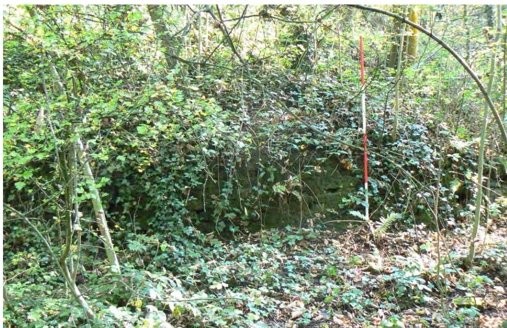
Plate 56: The revetment wall along the northern side of Lodge No 6, looking south-east
