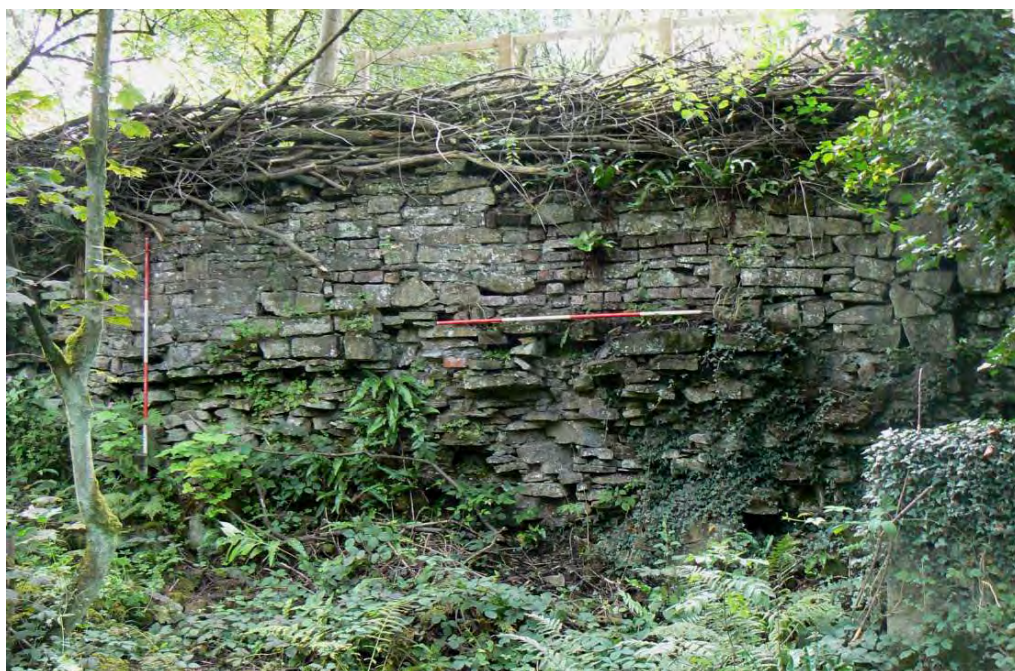
Plate 31: The northern wall of Room 21
