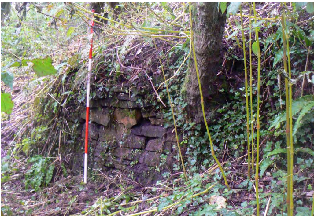
Plate 54: A section of the stone-built revetment wall for Lodge No 5, looking north-west
