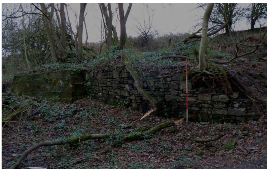
Plate 41: Extant fabric of the Plaiting-down Room (31), looking north-east
