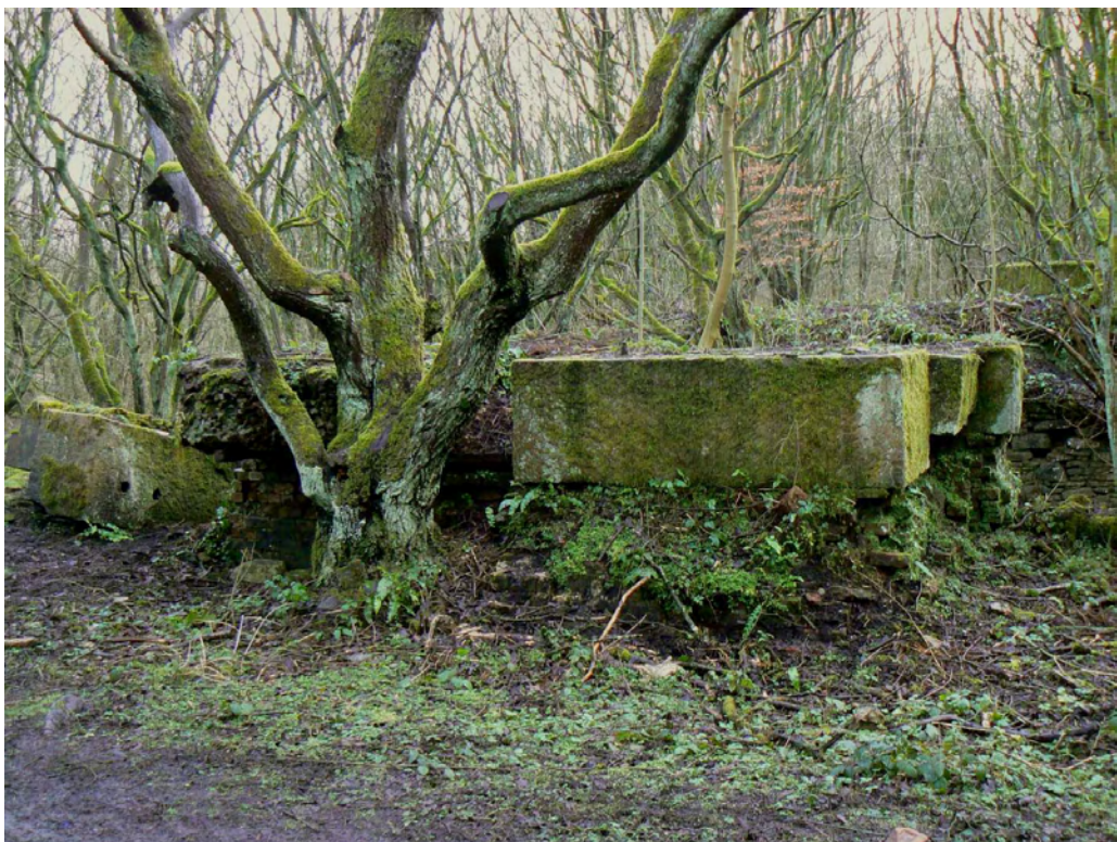
Plate 42: The remains of the foundation bed for the steam engine in the Grey Room (33)
