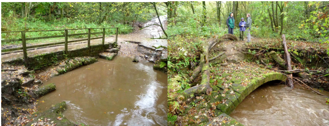
Culvert arch and bridge on east side of former works.
