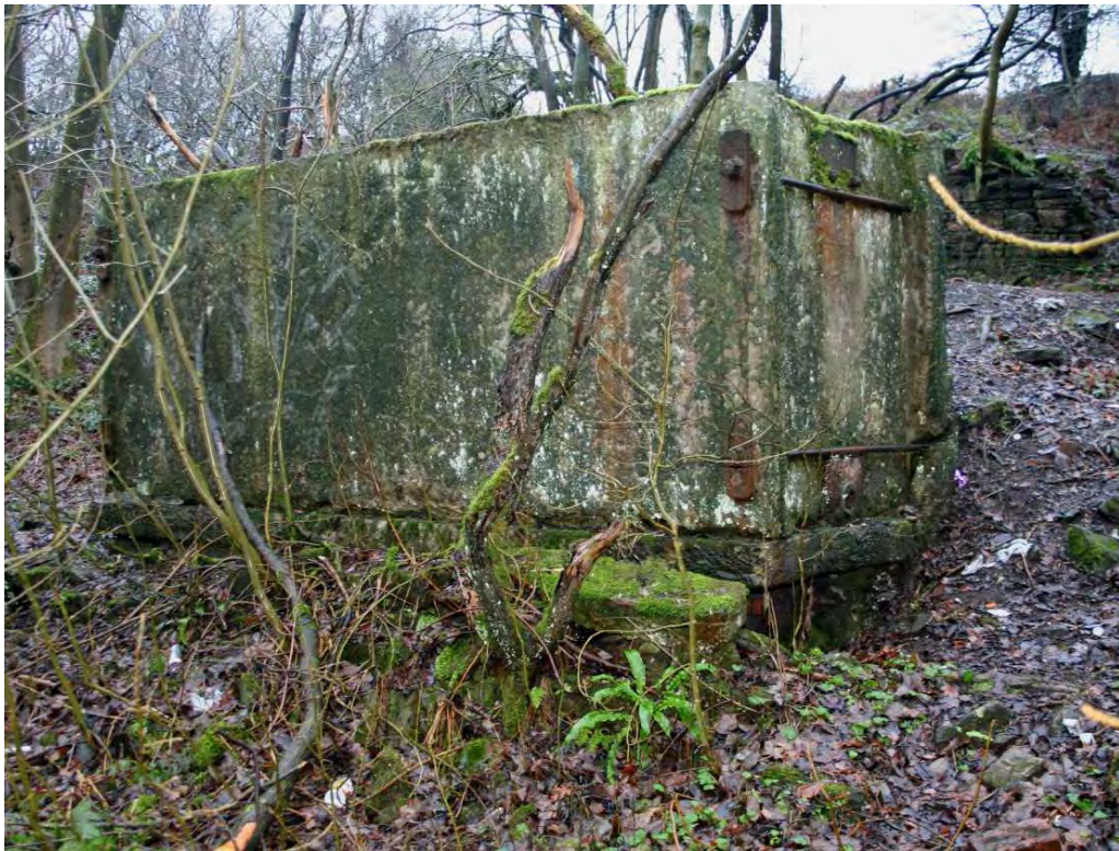
Plate 45: The chemic-mixing cistern in the Chemic Shed 43B
