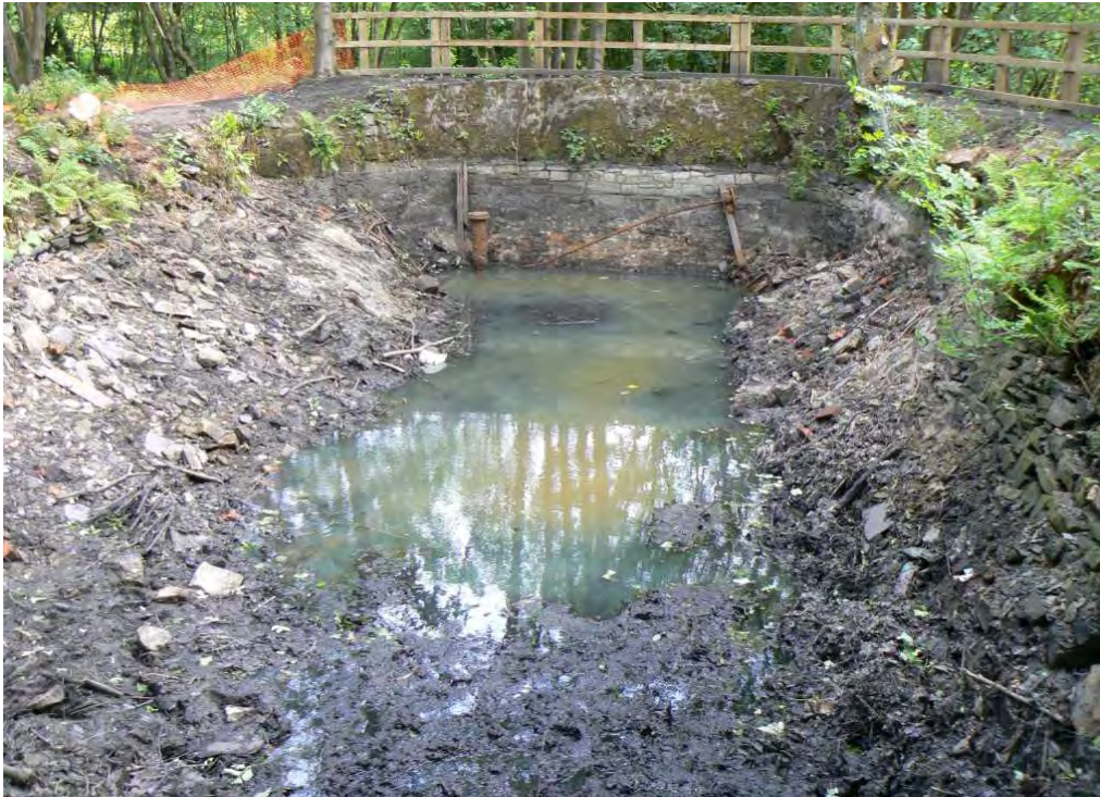
Plate 51: Lodge No 3, looking north-east during its conversion to a dipping pond
