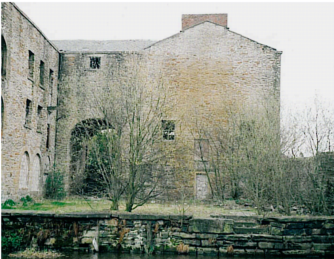
Plate 11: View of the north-facing elevation of west block in 2001 (courtesy of C Baker)
