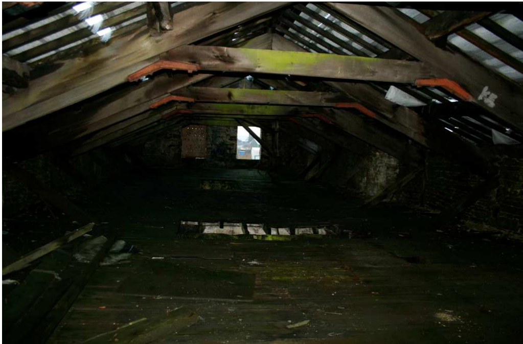
Plate 14: The roof structure and crane in the principal warehouse block
