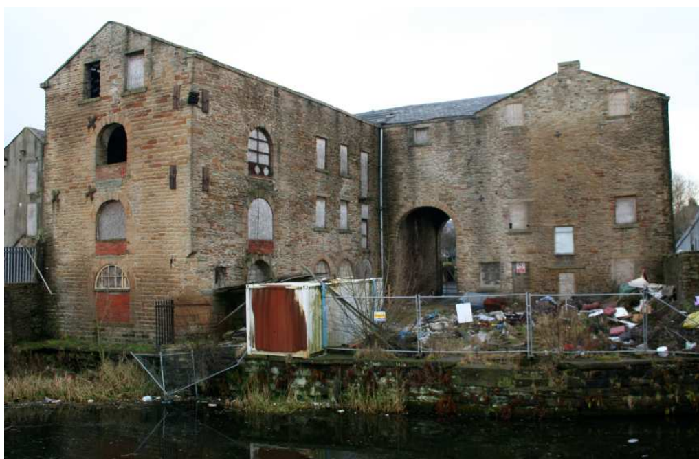
Plate 6: The north gable elevation of the warehouse, fronting onto the canal
