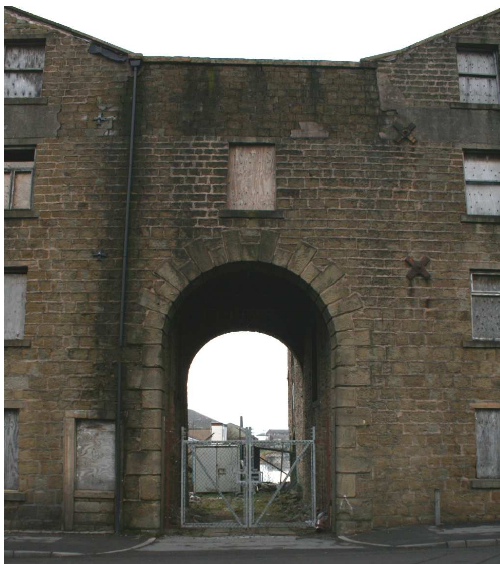
Plate 13: Detail of the central arch and the linking range
