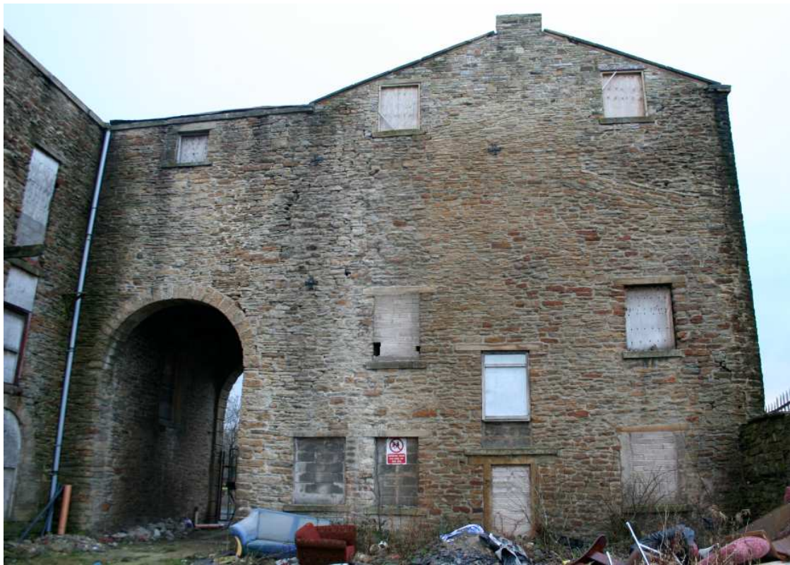
Plate 10: Current view of the north-facing elevation of west block
