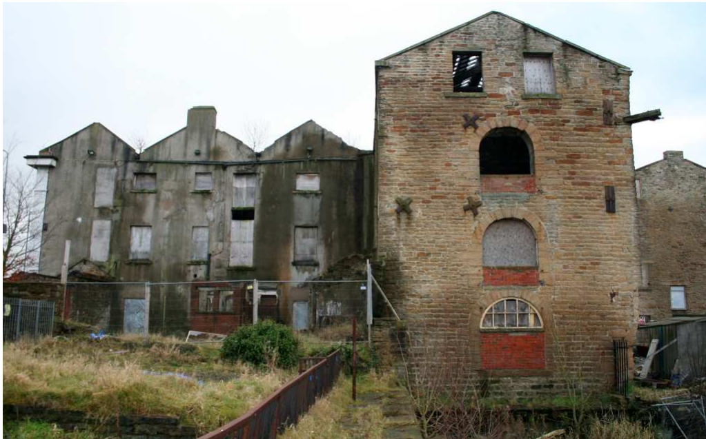
Plate 7: The north gable elevation, showing the Commercial Hotel to the left
