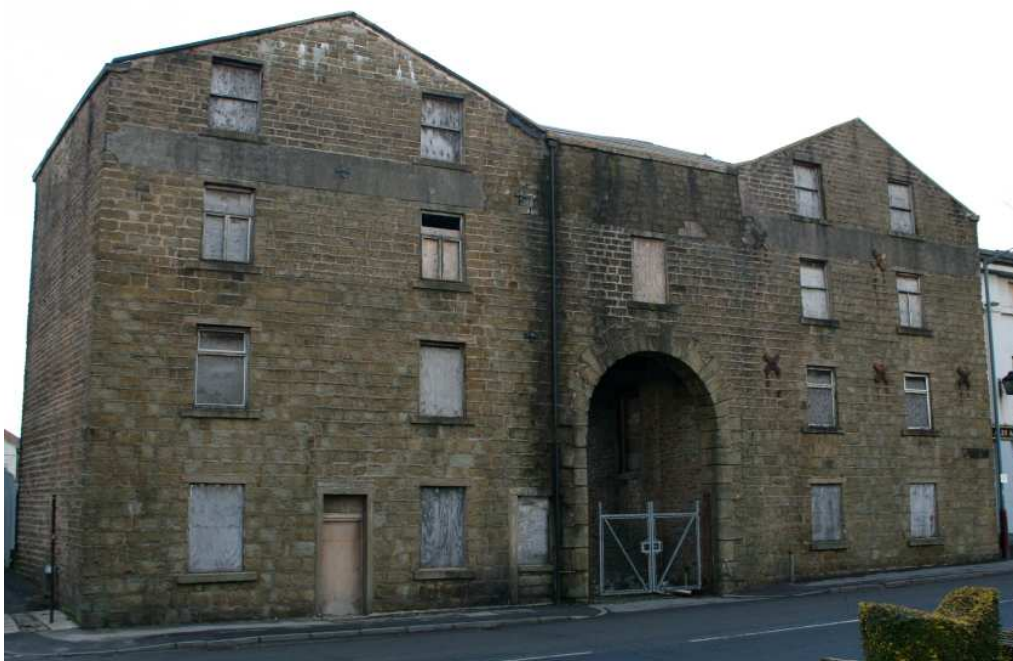
Plate 9: The south-facing elevation of the warehouse, fronting onto Blackburn Road
