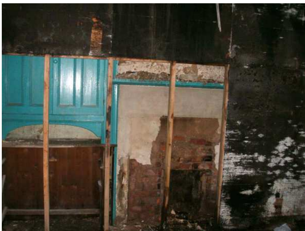
Plate 12: The remains of a cupboard and fireplace surviving behind modern cladding in the western room on the ground floor of the western block (courtesy of C Baker)
