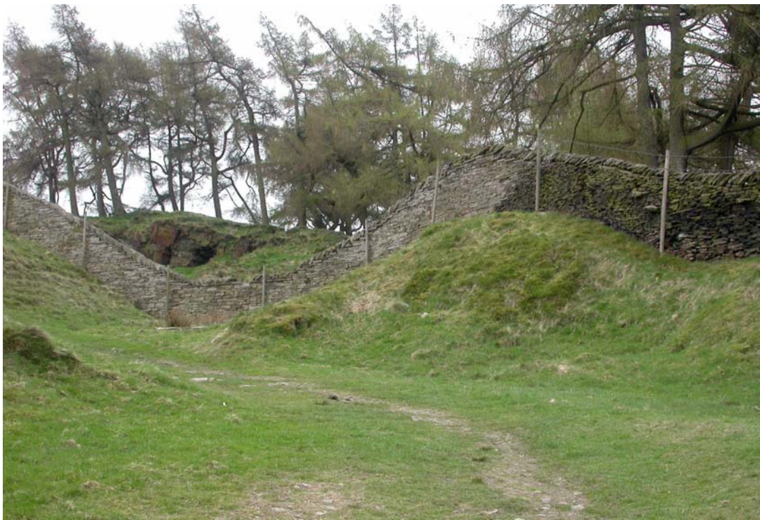
Repaired Hase Bank Wall (Recent Works 19)
