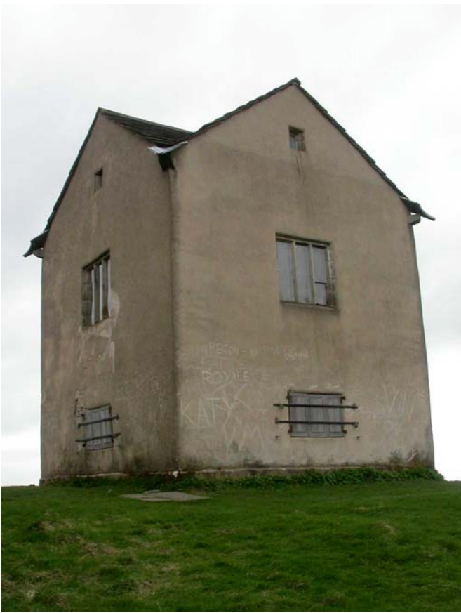
Restored Paddock Cottage - looking north (Recent Works 21)
