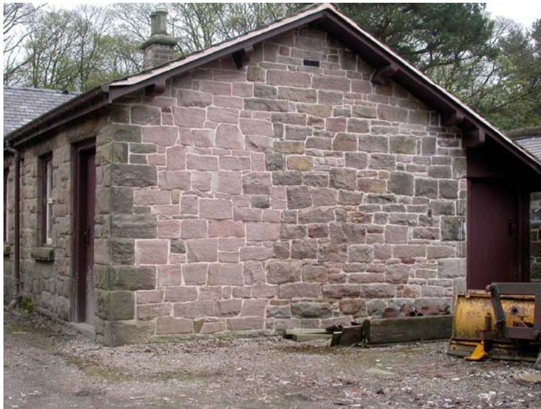
The Kennels following refurbishment - showing repairs to the eastern wall (Recent Works 5)
