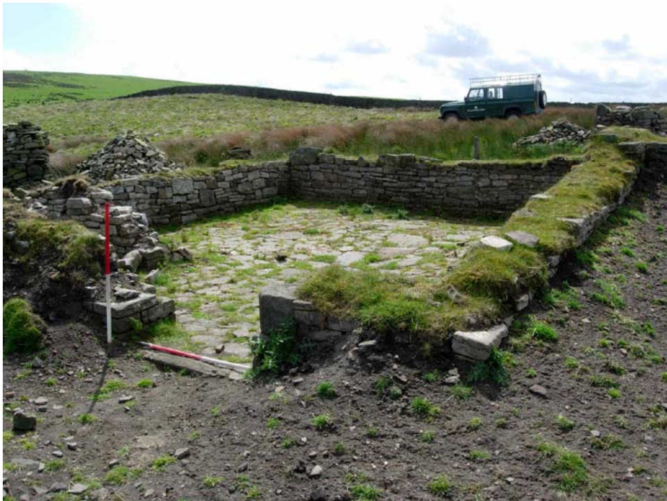
The Stag House following excavation
