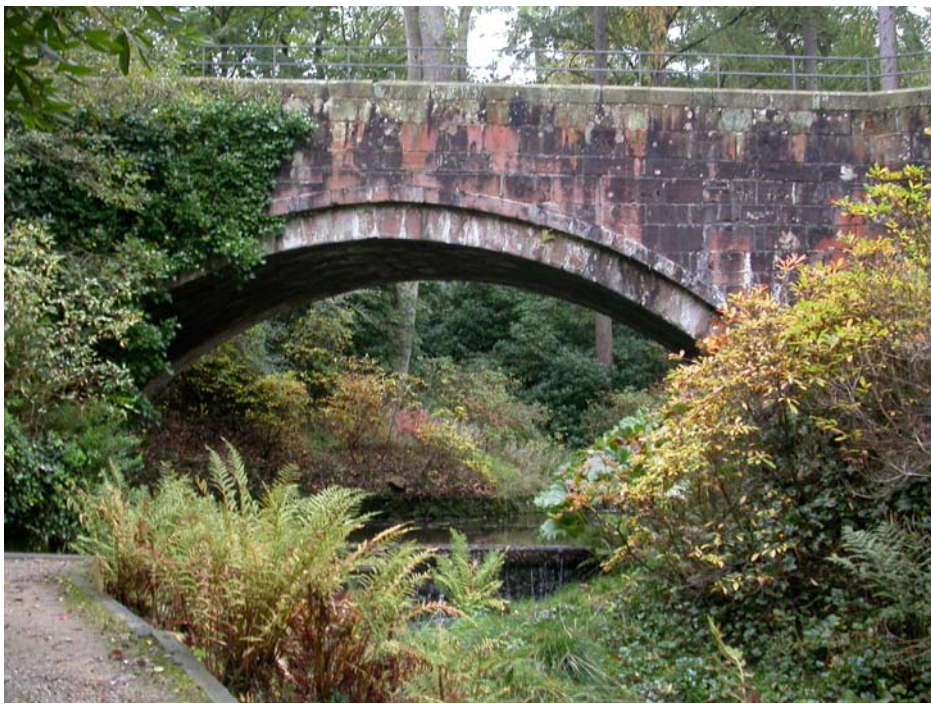
Hampers bridge over Killtime (c 1751). If the arch included in the c1740 plan was built and subsequently reused, the present structure may have reclaimed the stone, which may explain the numbered blocks in the bridge.
