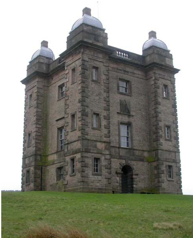
The cage following a major programme of restorations (Recent Works 5)
