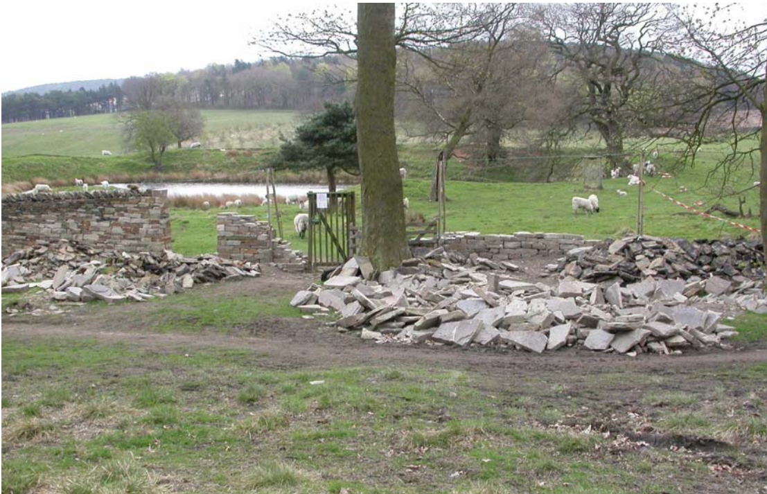
Wall by Drinkwater Round during restoration (Recent Works 24)
