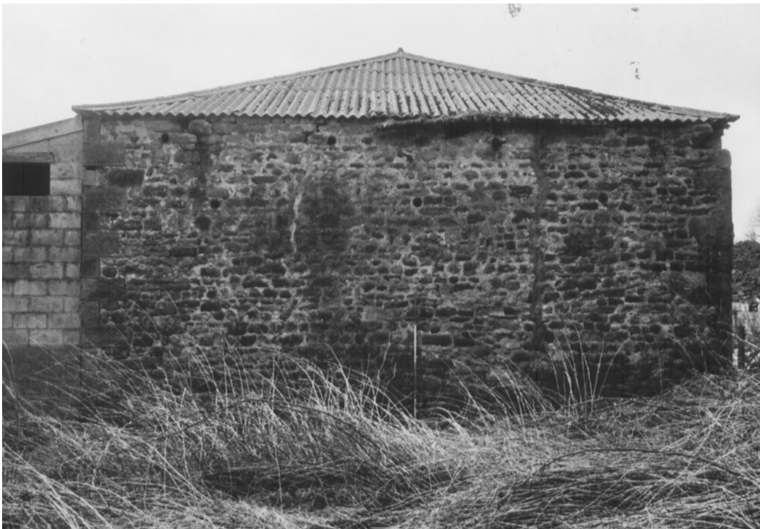
Plate 4: The north elevation of the barn
