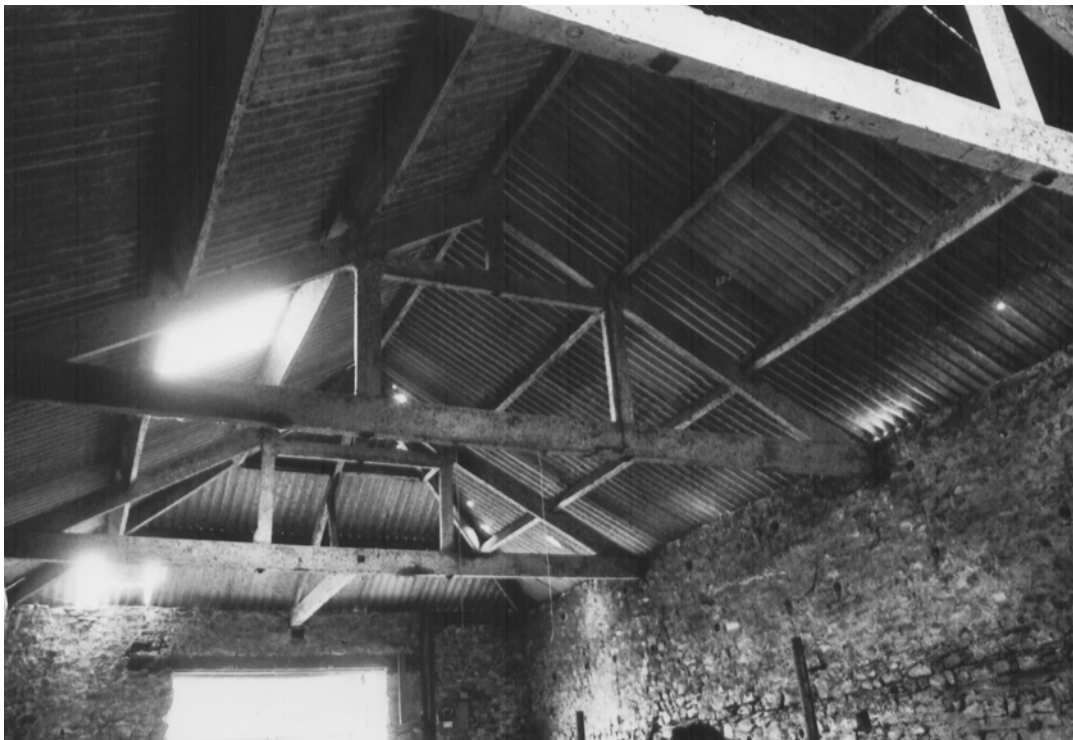
Plate 8: Detail of the roof trusses at the south end of the building
