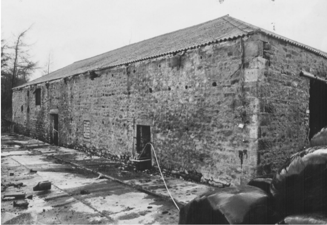
Plate 3: The west elevation of the barn
