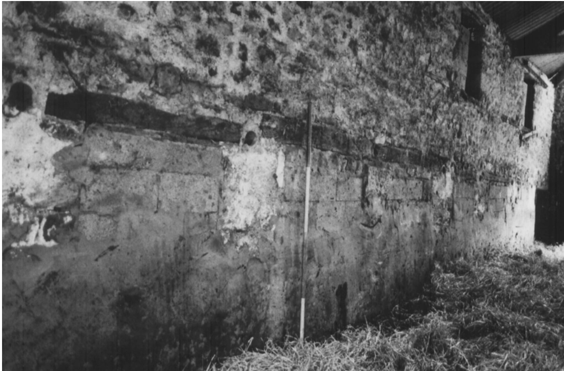
Plate 9: Detail of the blocked windows on the east elevation
