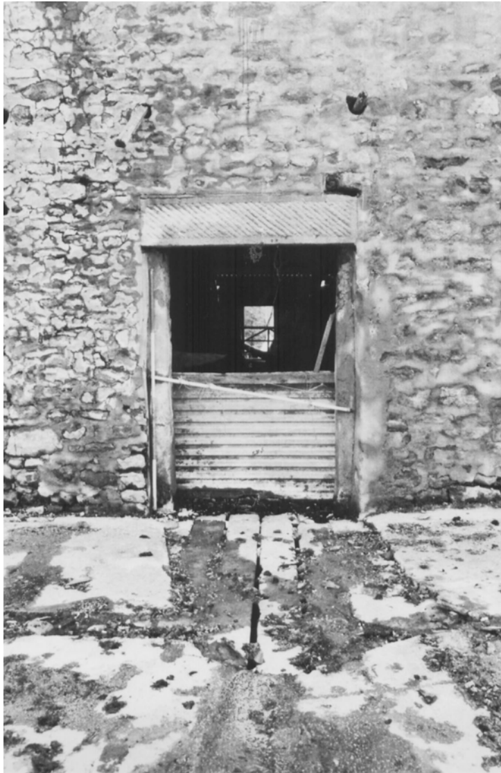
Plate 6: Detail of a partially blocked door on the west elevation, featuring a “rusticated” sandstone lintel
