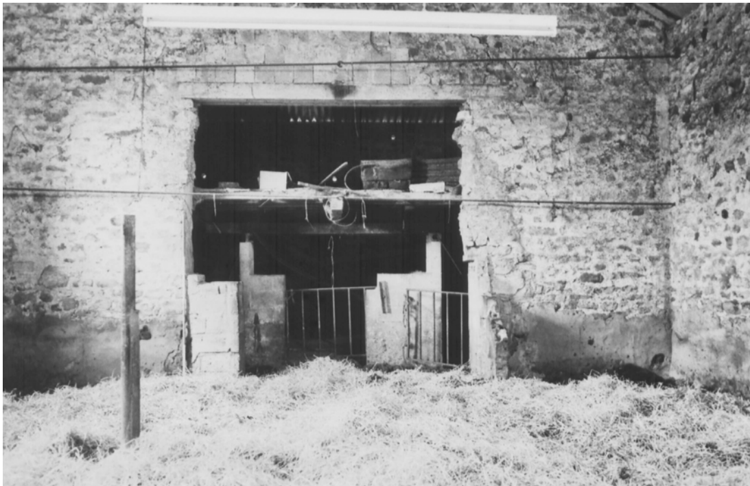
Plate 10: The entrance to the shippon at the north end of the barn
