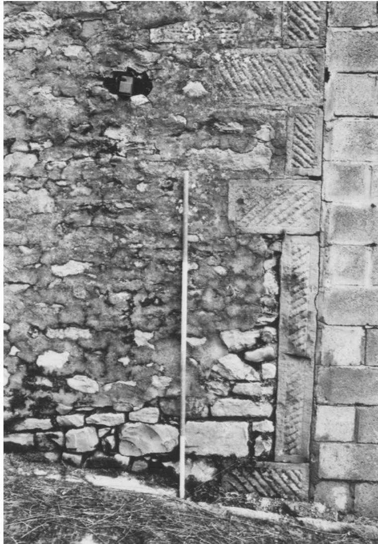
Plate 5: Detail of the “rusticated” sandstone quoins on the south elevation
