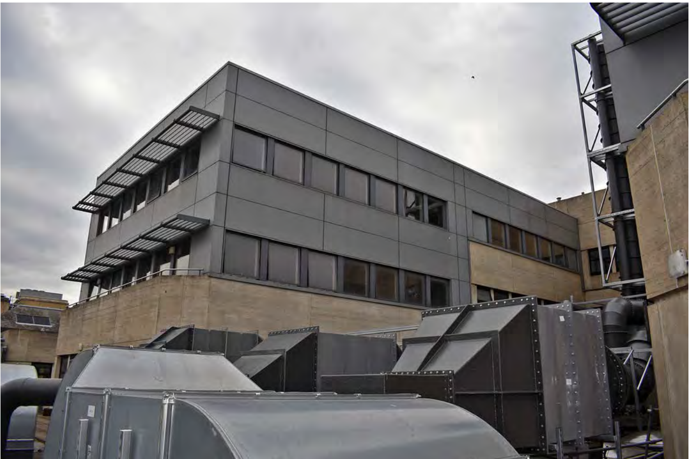
Plate 10: Additional floor, or 'pods' built onto the south range of the Tinbergen Building, looking north-west
