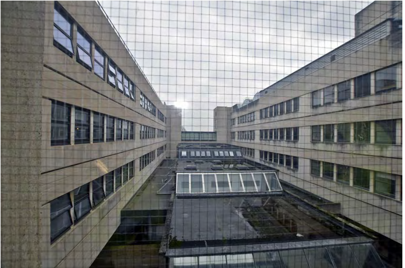
Plate 29: Level E of the Tinbergen Building, looking east
