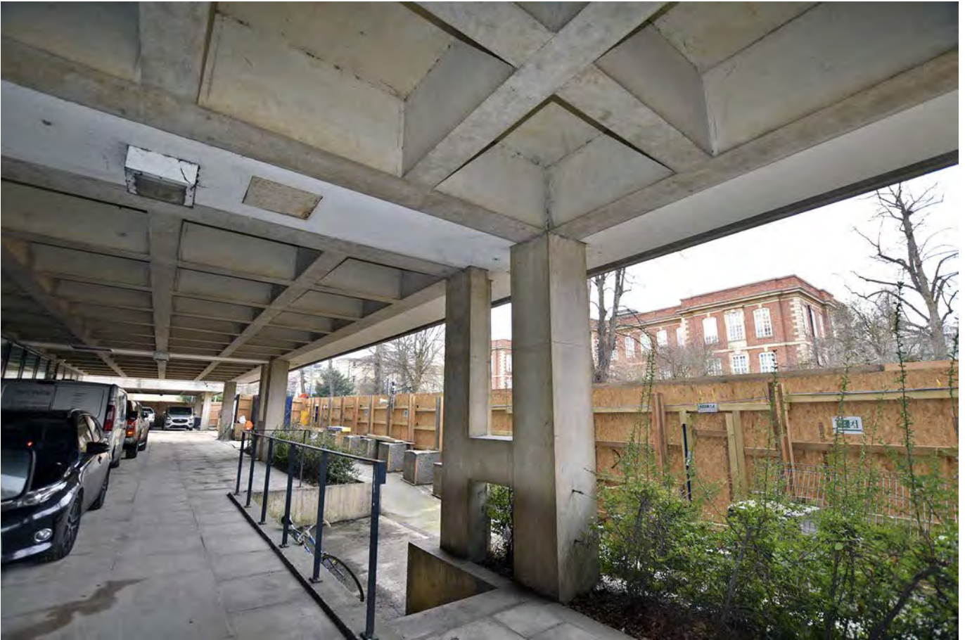
Plate 9: Covered walkway area at Level A on the north side of the Tinbergen Building, looking north-west
