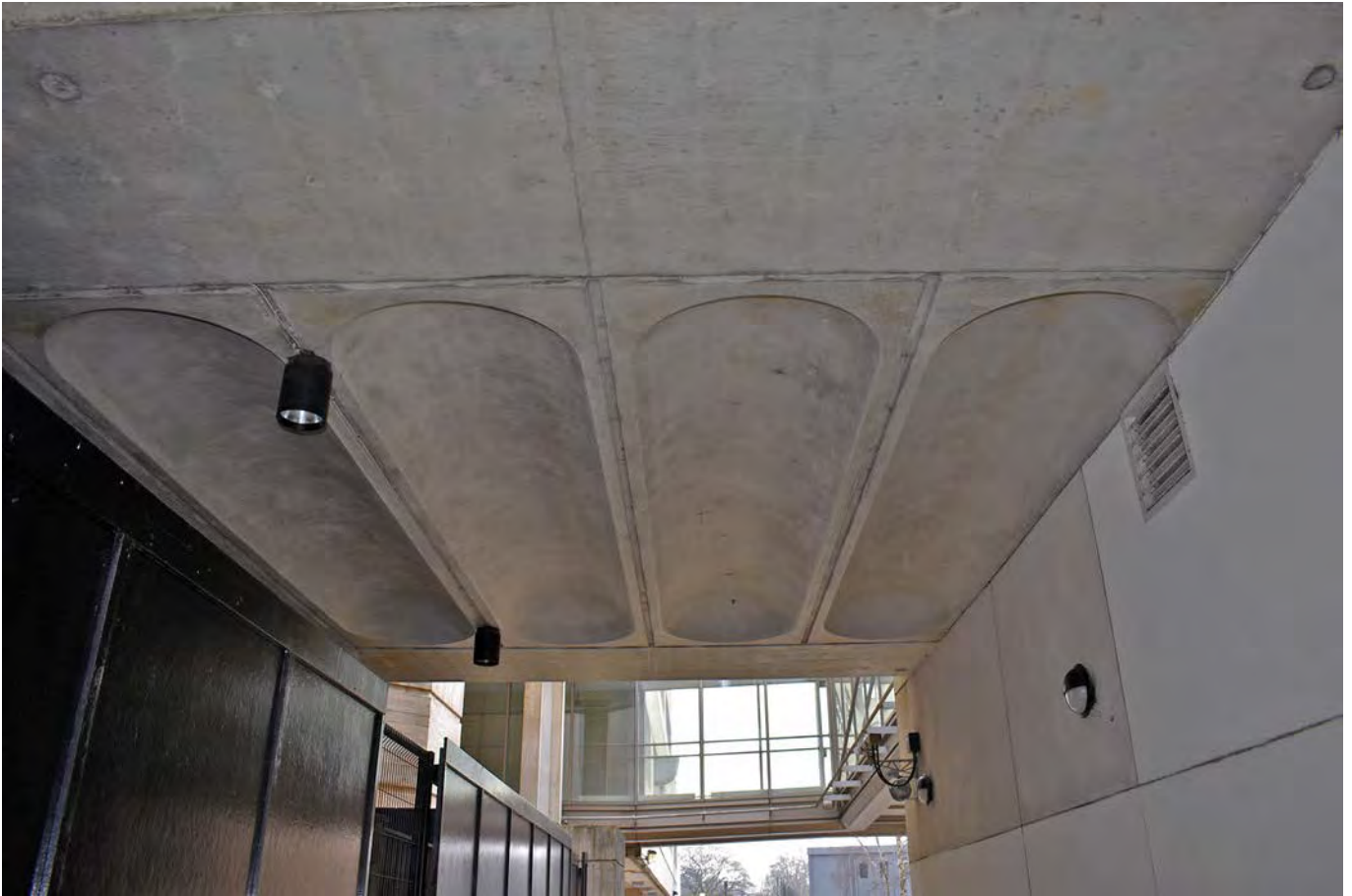
Plate 13: Underpass on west side of Level A of the Tinbergen Building, looking south
