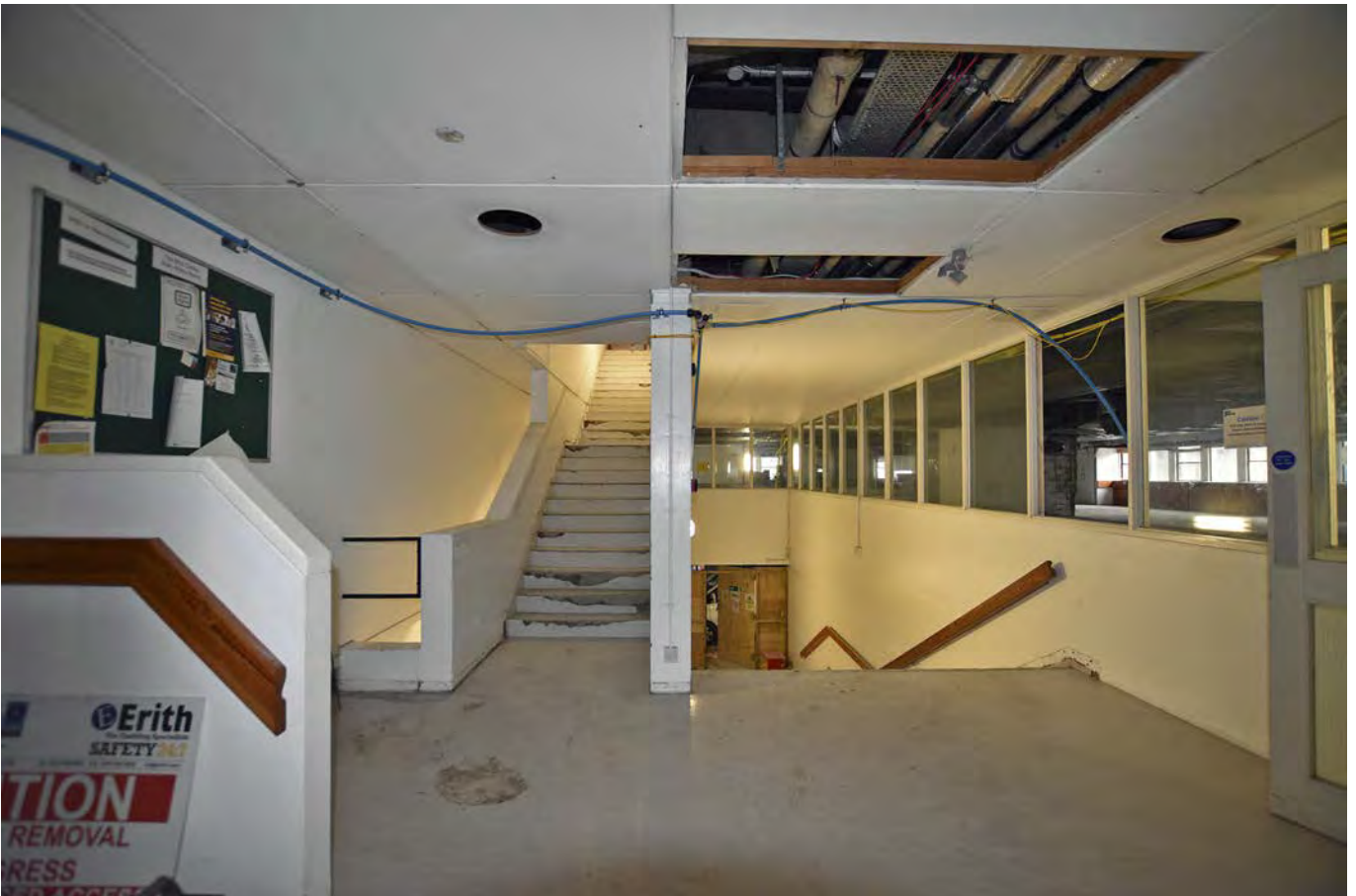
Plate 26: Level E of the Tinbergen Building, looking east
