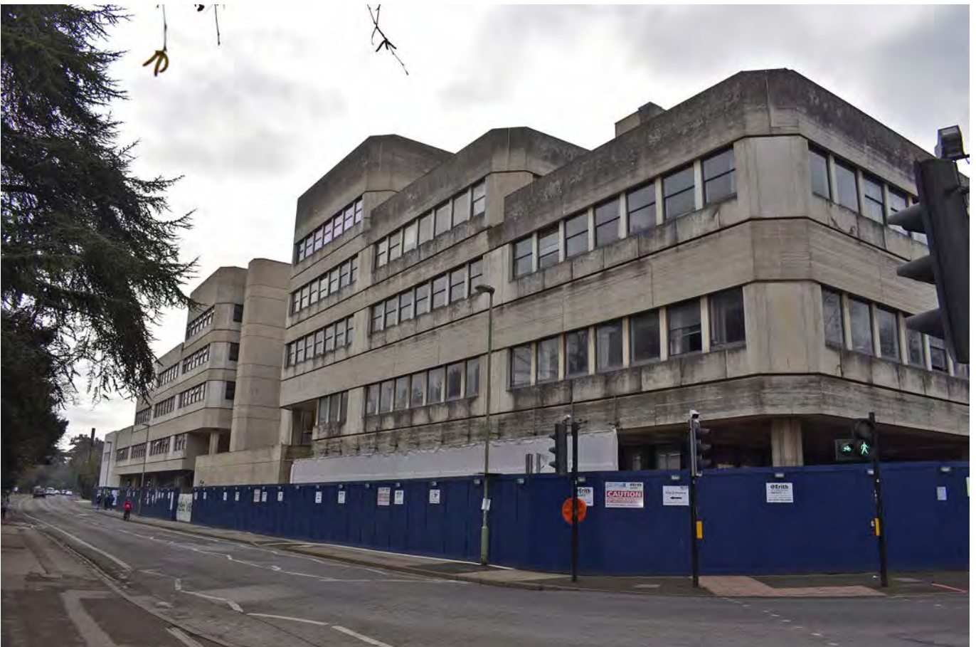
Plate 2: East facing range of the Tinbergen Building, looking south-west
