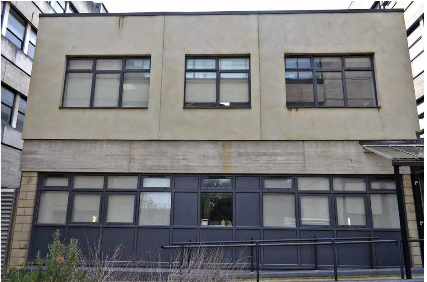
Plate 11: Structure built into the central east to west divide of the Tinbergen Building, looking west
