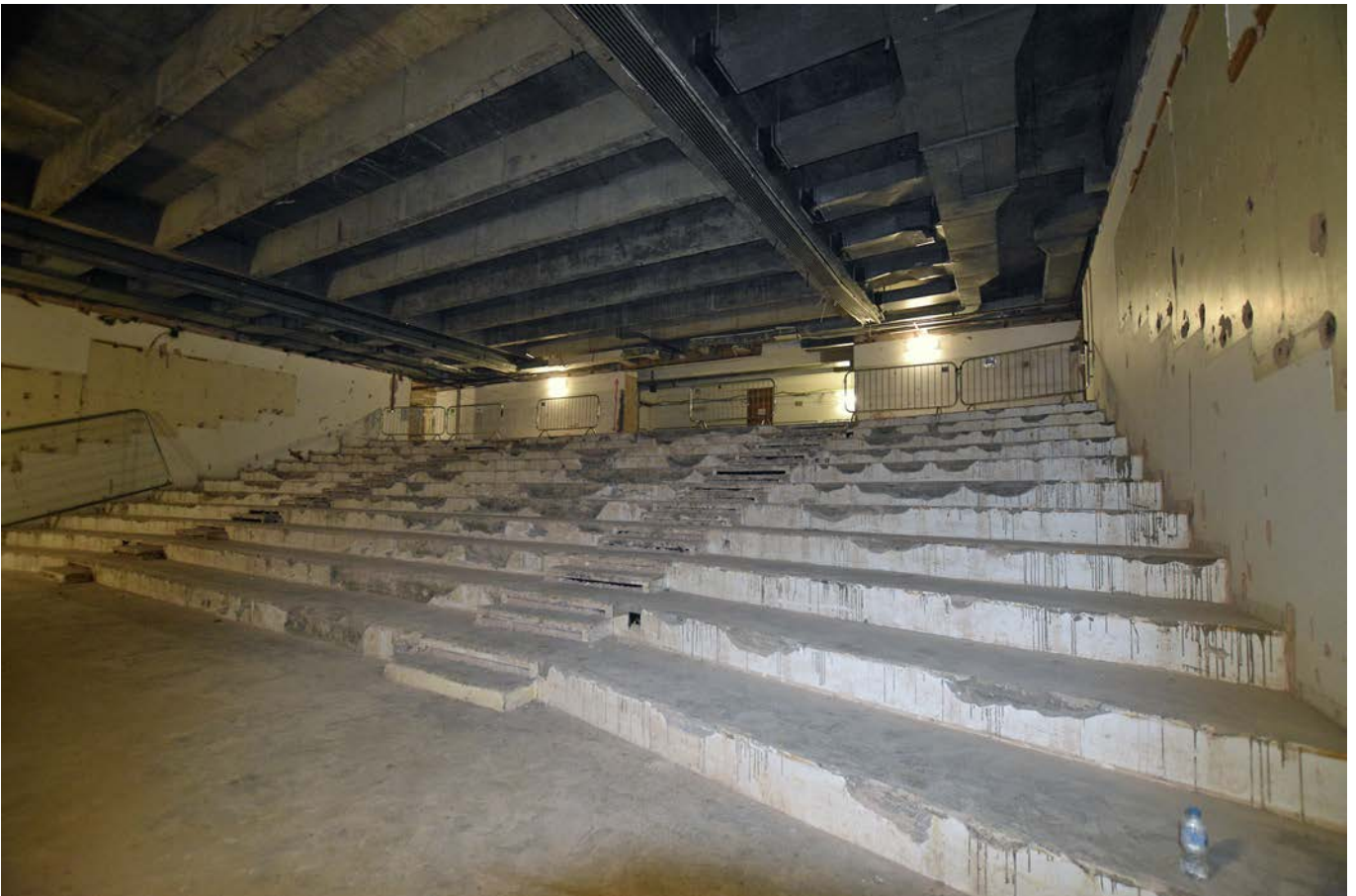
Plate 18: Lecture theatre in Level A of the Tinbergen Building, looking north-east
