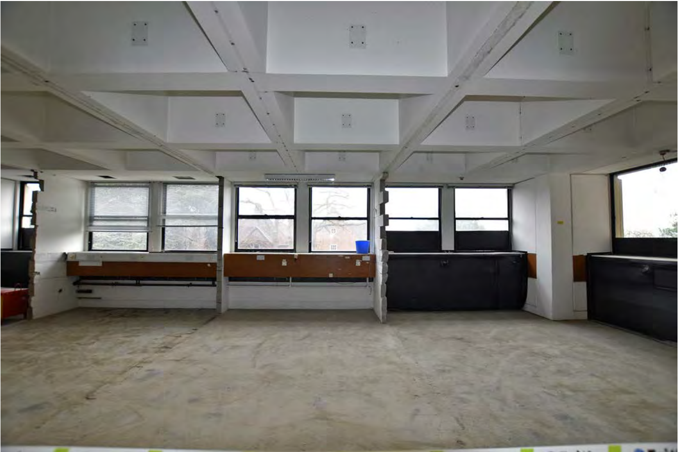
Plate 25: Level D of the Tinbergen Building, looking east
