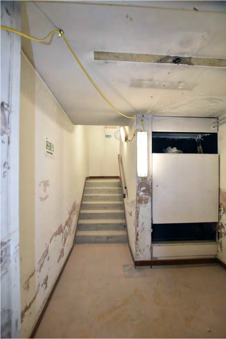
Plate 27: Level B of the Tinbergen Building, looking west
