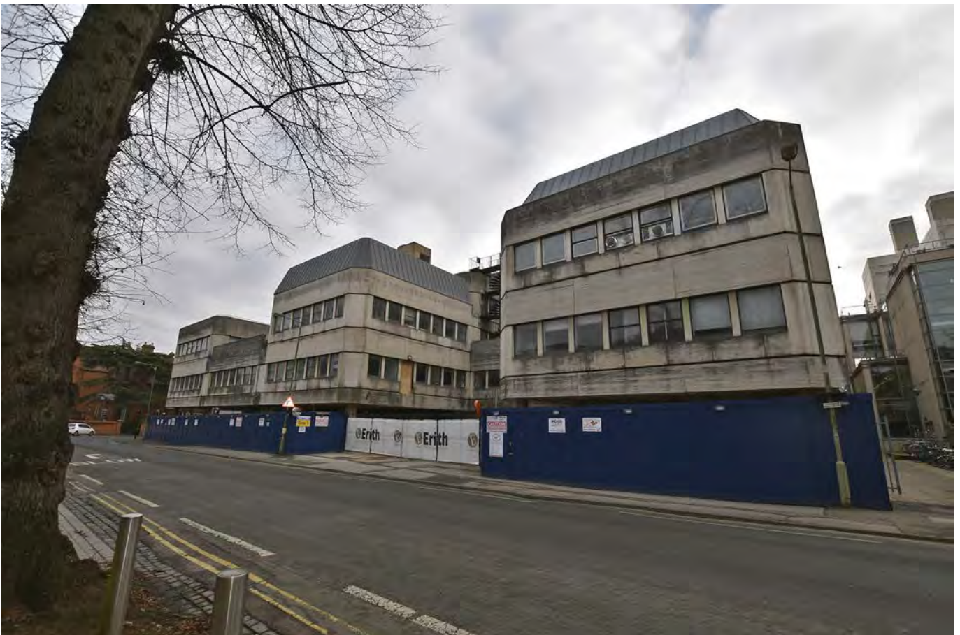
Plate 6: North facing range of the Tinbergen Building, looking south-east
