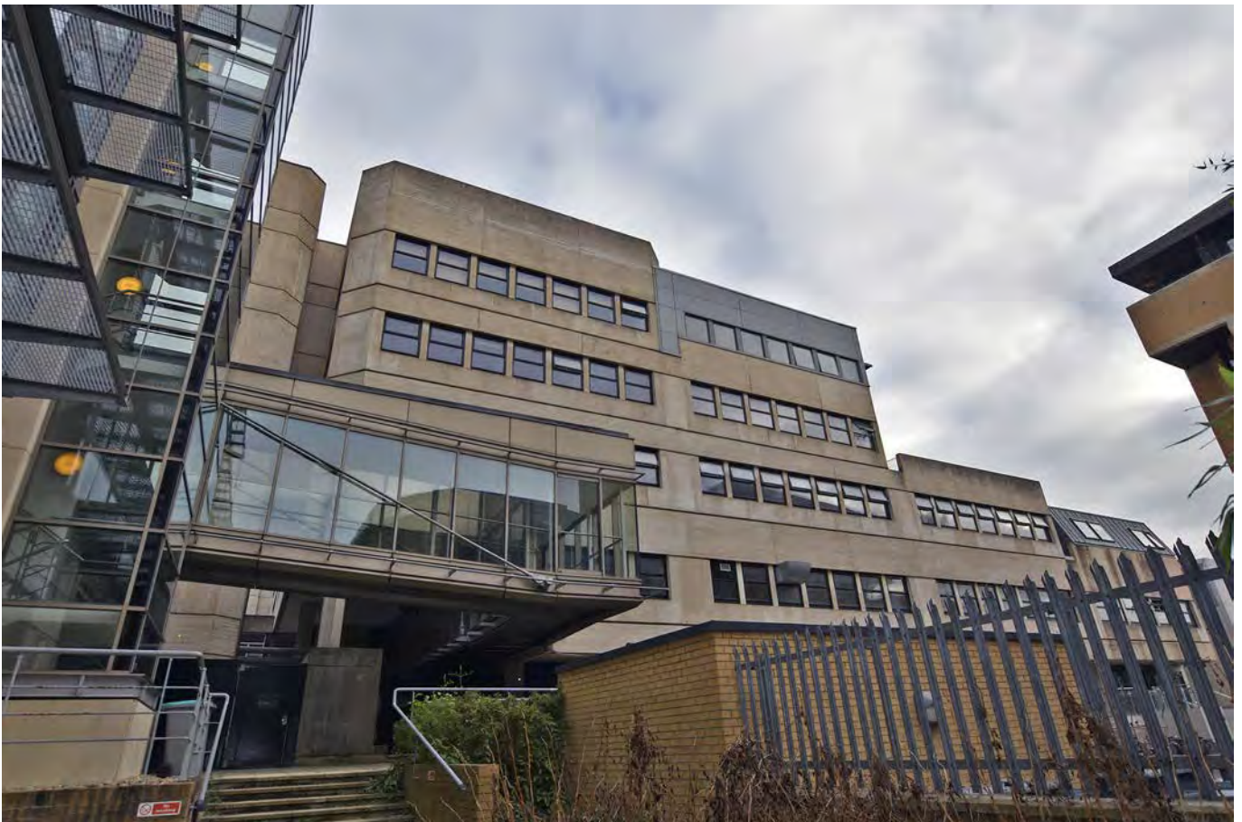
Plate 12: The west range of the Tinbergen Building, looking south-east
