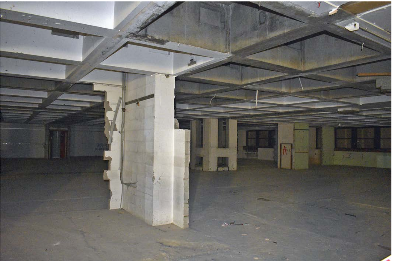
Plate 20: Level B of the Tinbergen Building after asbestos removal, looking south-west
