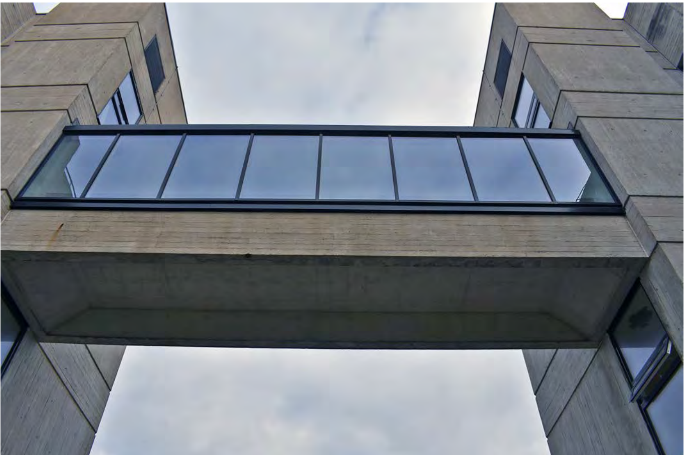
Plate 4: Walkway between stair turrets at Level E in the east range, looking west
