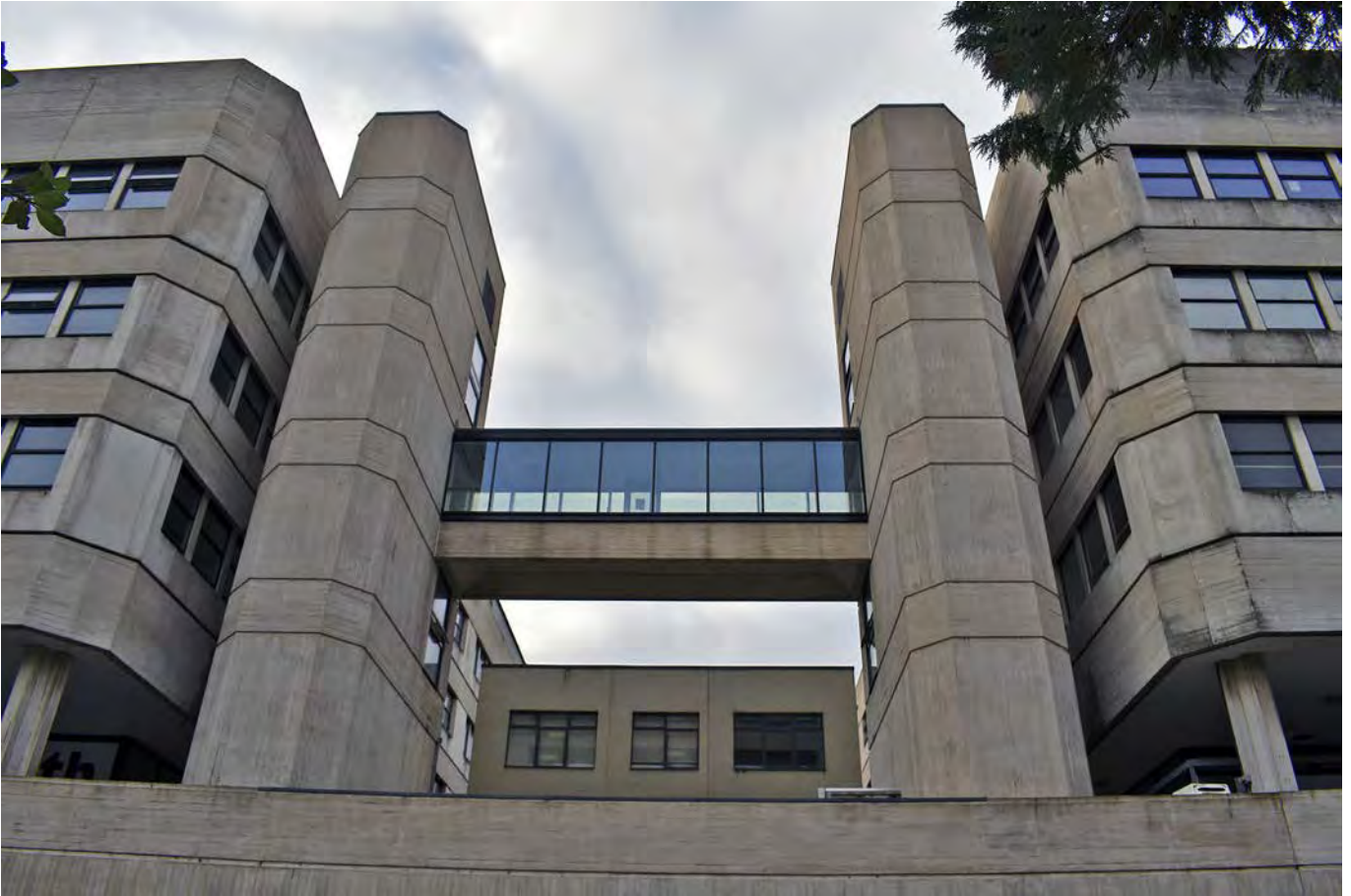
Plate 3: Central recess in the east facing range of the Tinbergen Building, looking west
