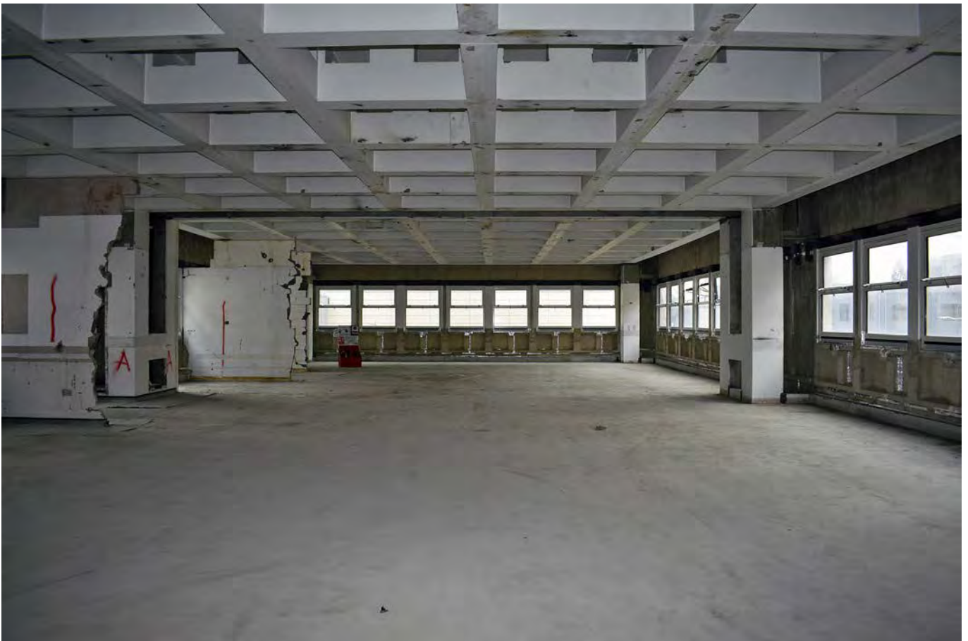
Plate 24: Level E of the Tinbergen Building, looking north
