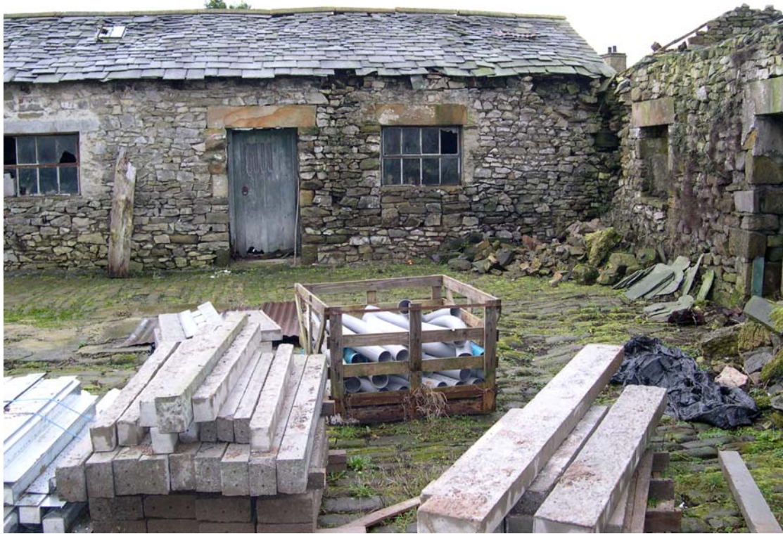
Plate 8: The west elevation of Building Five
