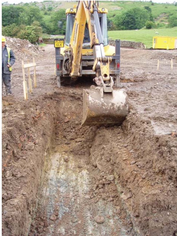
Plate 10: Working shot taken during excavation of Trench 1, looking west
