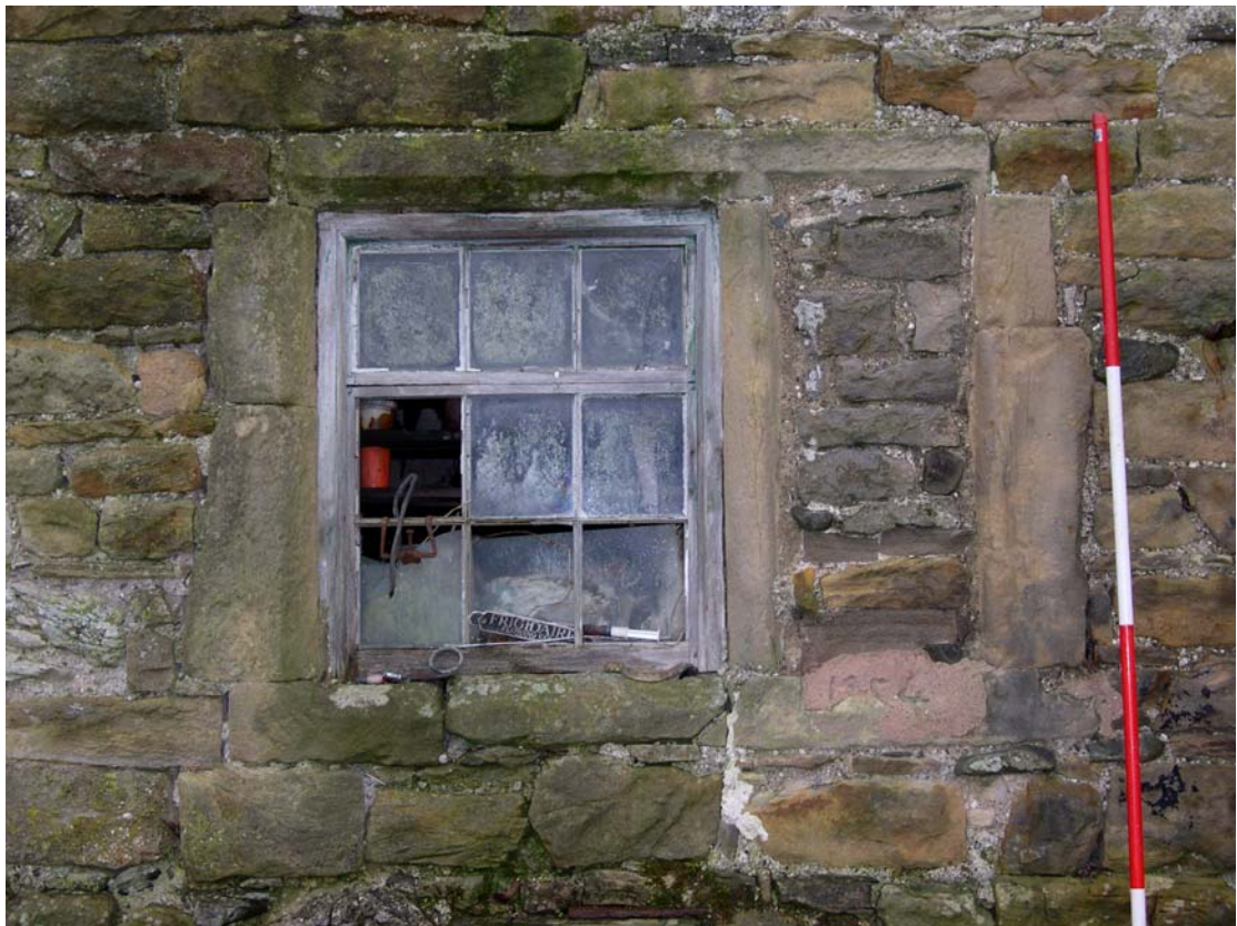
Plate 3: Detail of the chamfered and rebated mullioned windows
