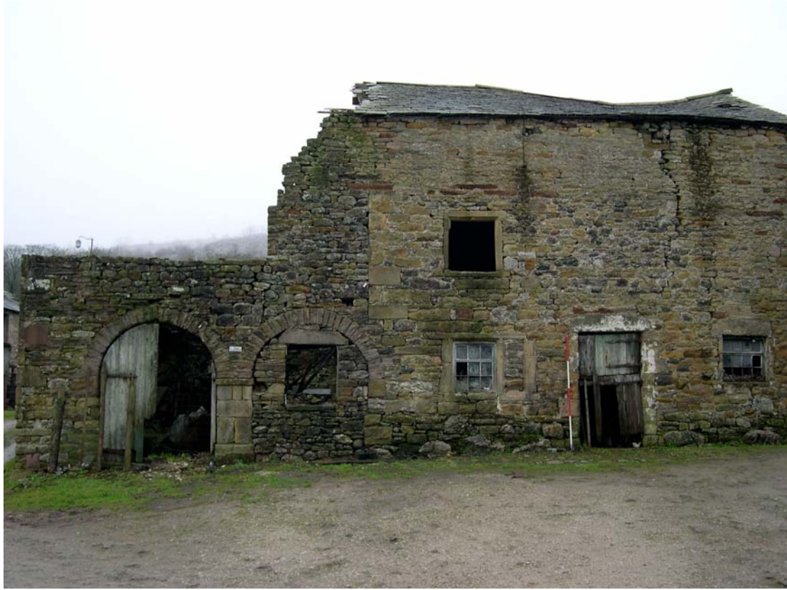
Plate 2: The east elevation of Building One , with the south extension to the left of the plate
