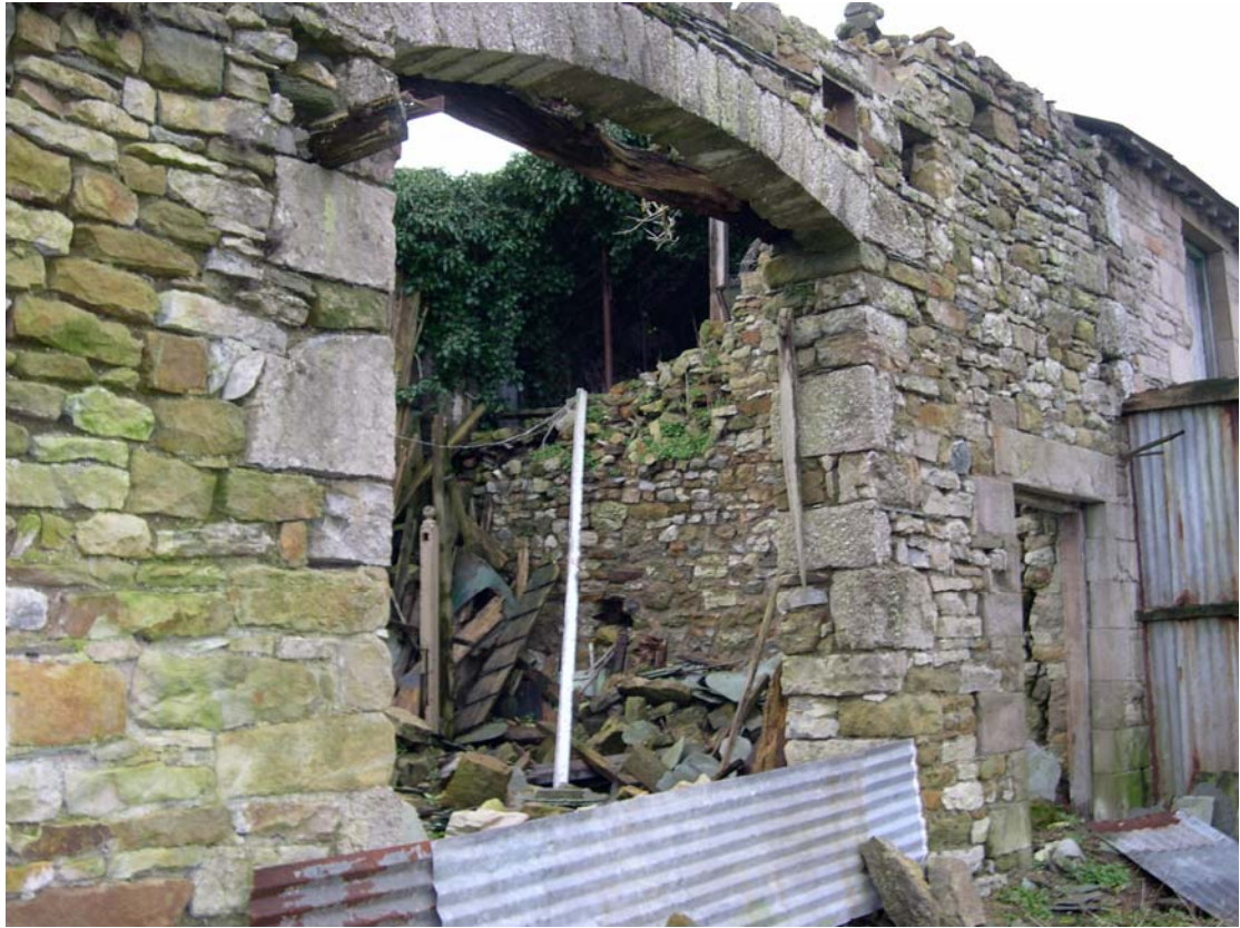
Plate 6: Detail of a wagon door on the north elevation of Building Three
