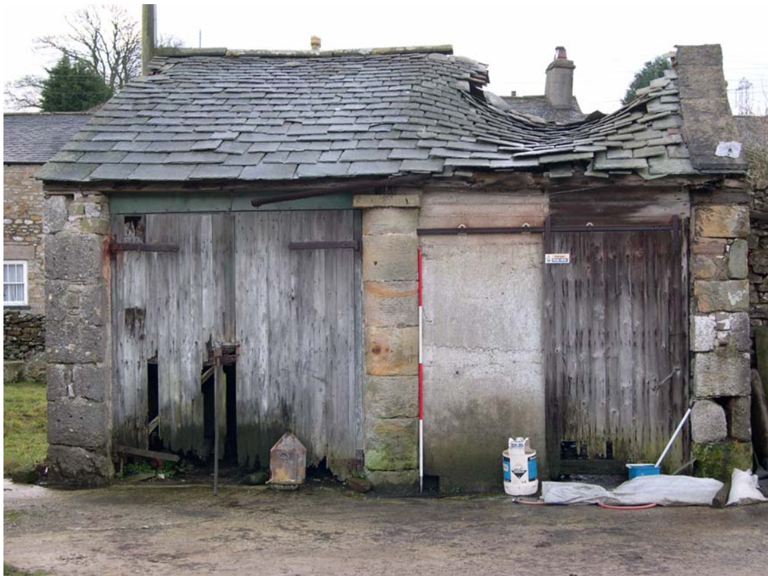
Plate 9: The west elevation of Building Six
