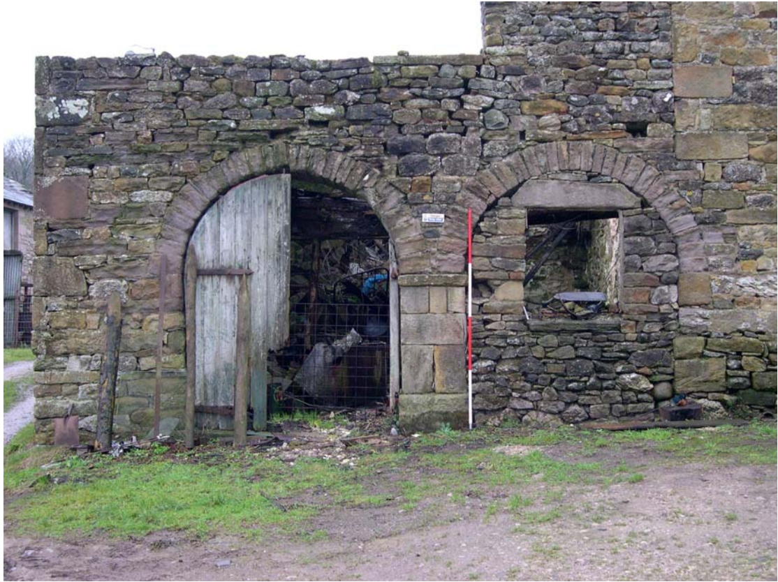
Plate 4: The double-arched wagon door of the south extension
