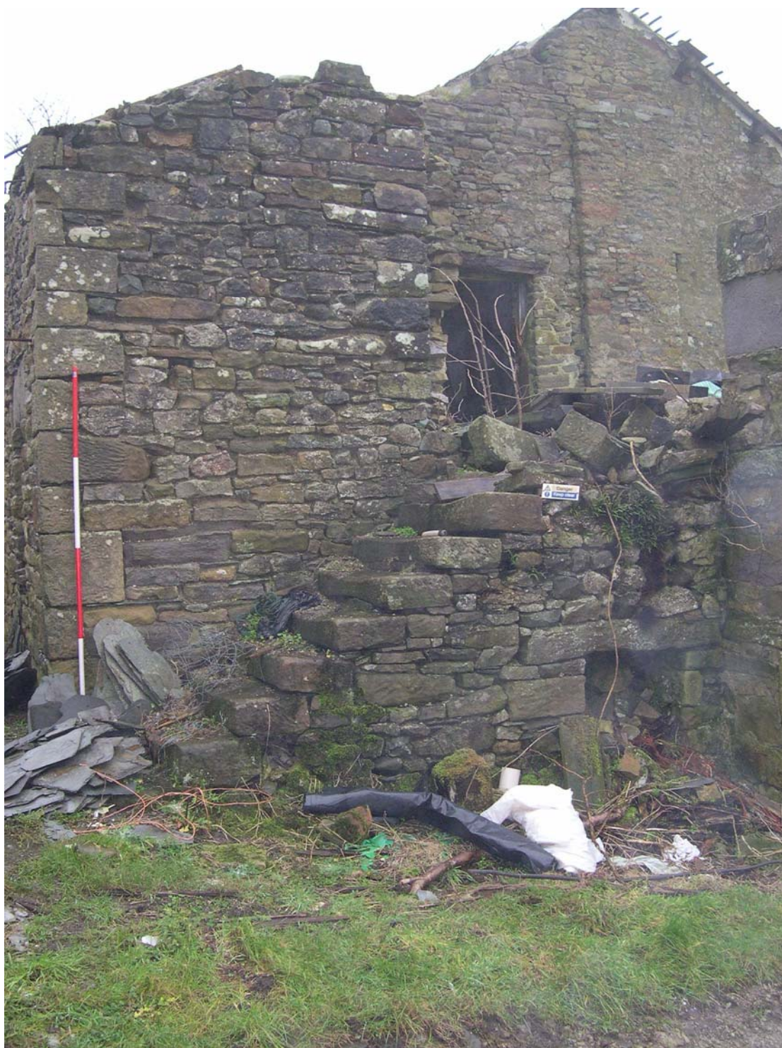
Plate 5: The outshut with its external stone staircase
