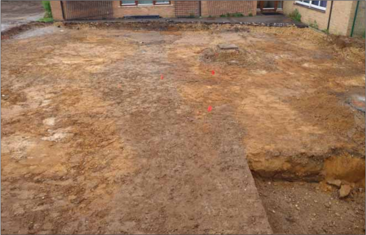
Plate 7: Pre Excavation shot of Ditches 149/173 and 151/175
