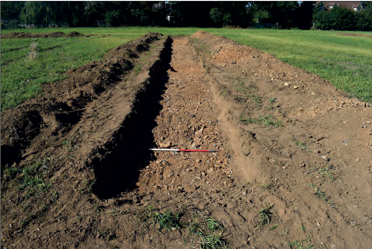
Plate 5: Trench 59 showing natural flints and Peddars Way ditches (middle and far distance). Looking north-west.
