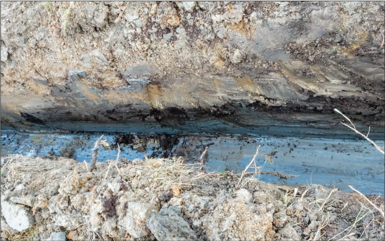
Plate 3: Section of pipe trench showing the peat layer
