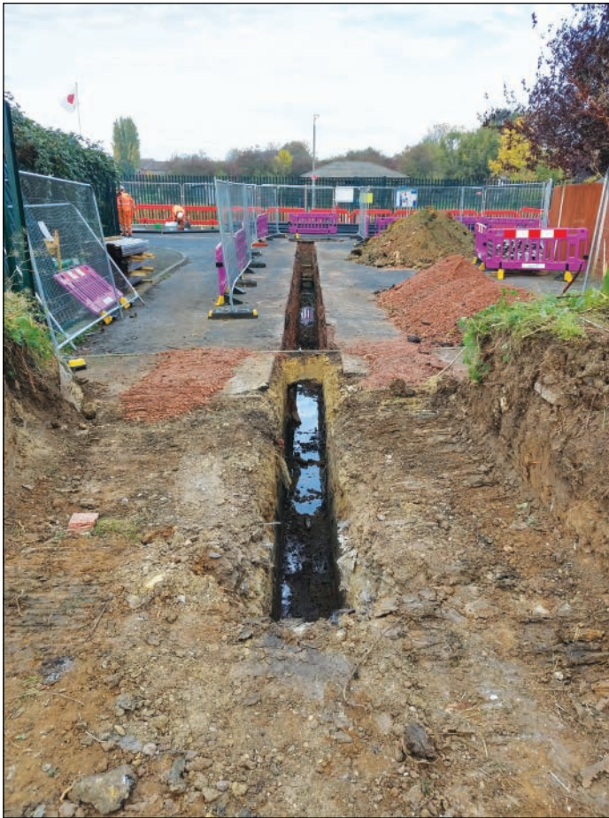
Plate 1: View north-west into Churchill Road at the start of the pipe trench
