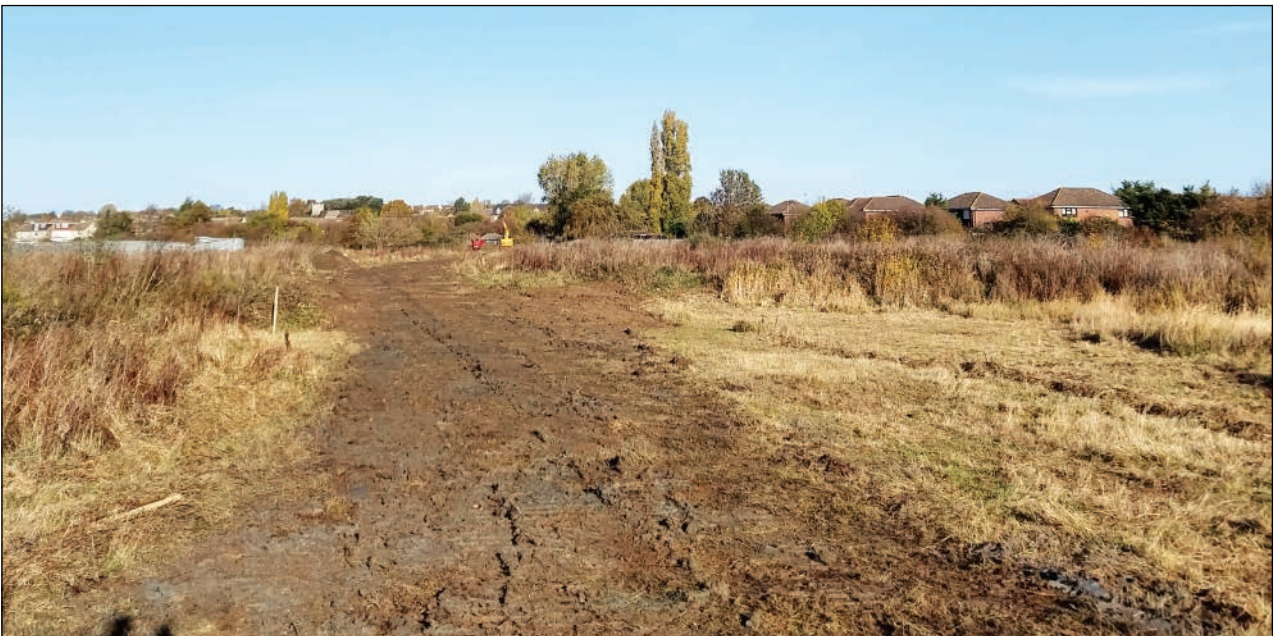
Plate 4: View north-west across backfilled pipe trench
