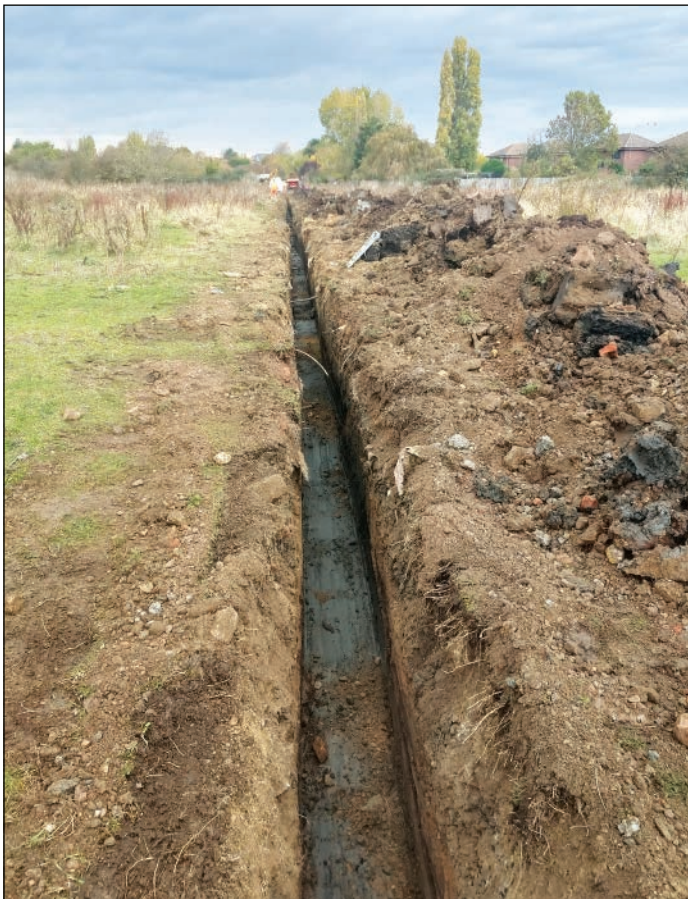
Plate 2: View south-east down the pipe trench, with modern debris evident in the spoil
