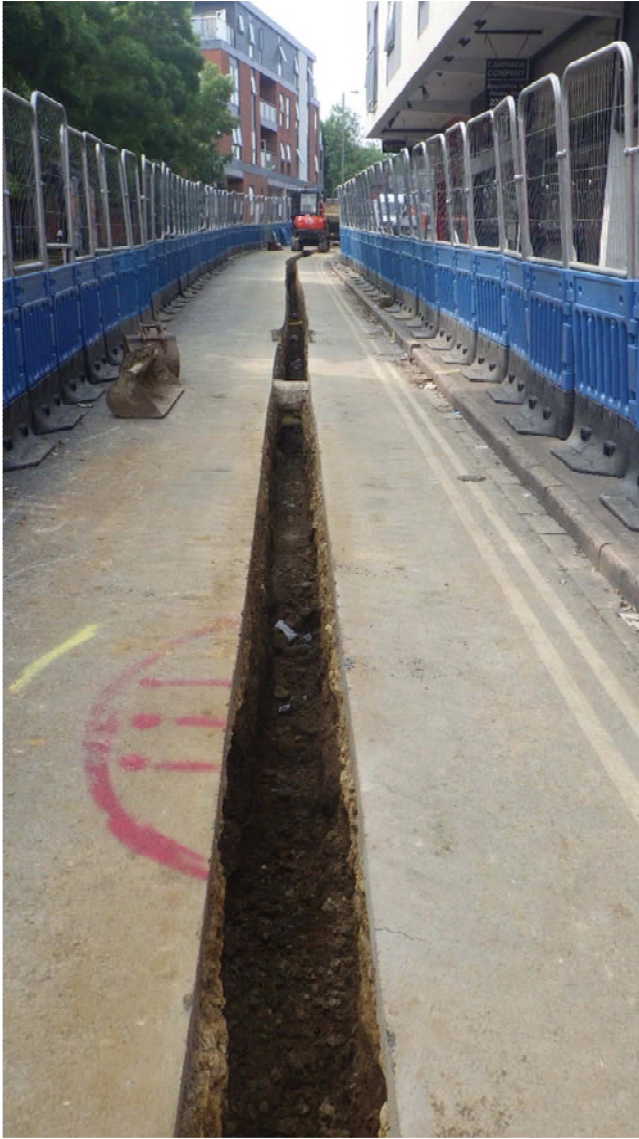
Plate 1: Excavations for the new water main
