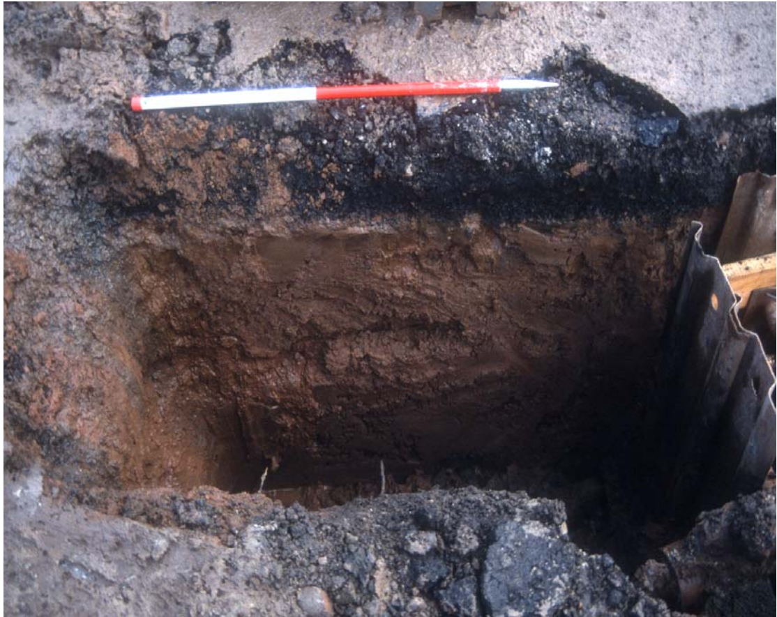
Plate 1: West-facing section of manhole
