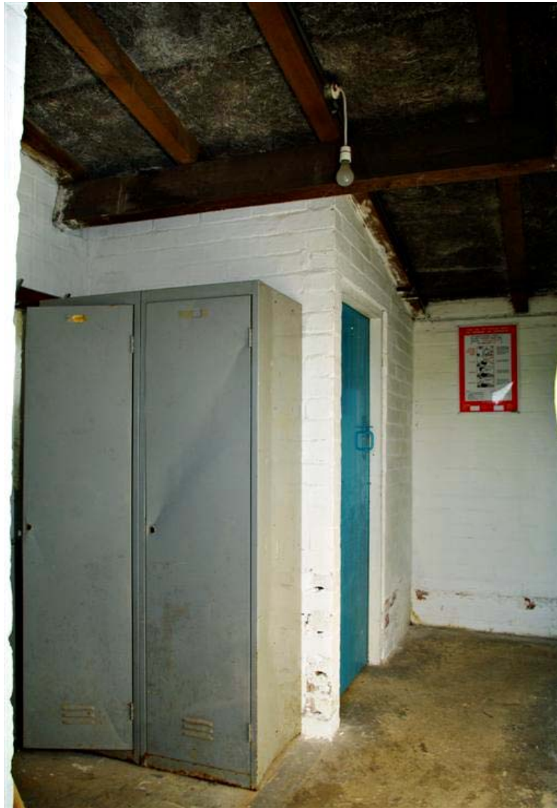
Plate 8: General appearance of the interior of the west end of Fisherman's Hut, with the toilet cubicle in the corner.
