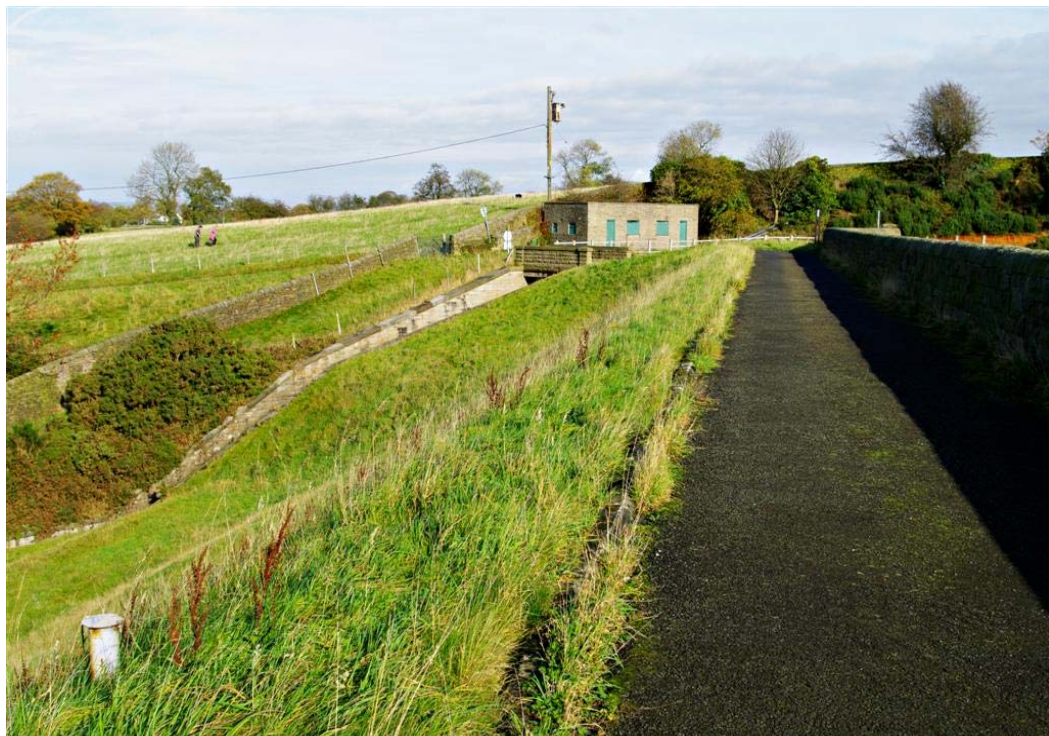
Plate 4: General view of the area around the Fisherman's Hut, with the Bollinghurst Reservoir wall in the foreground.
