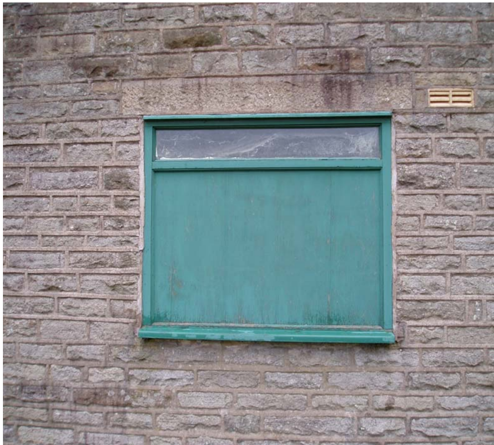
Plate 7: Window detail in the front elevation of the Fisherman's Hut.
