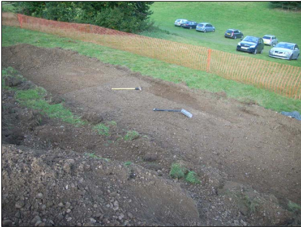
Plate 5: working shot of Ditch 1 under excavation, looking north east
