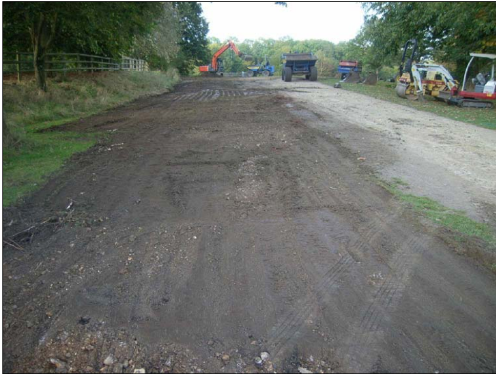
Plate 7: View of topsoil strip across the north of site after rotovation of the grass, looking north east
