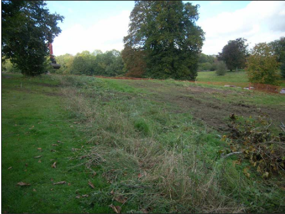
Plate 3: Area of main watching brief after the removal of trees and modern fence, looking north east
