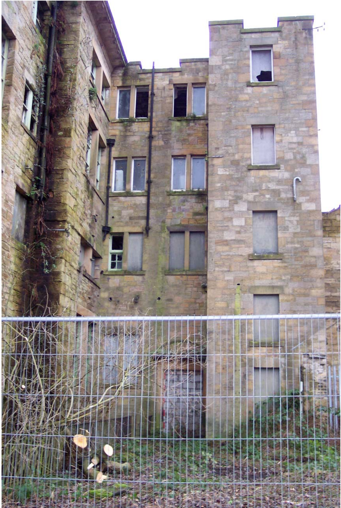
Plate 1: The east elevation of the Toilet Block
