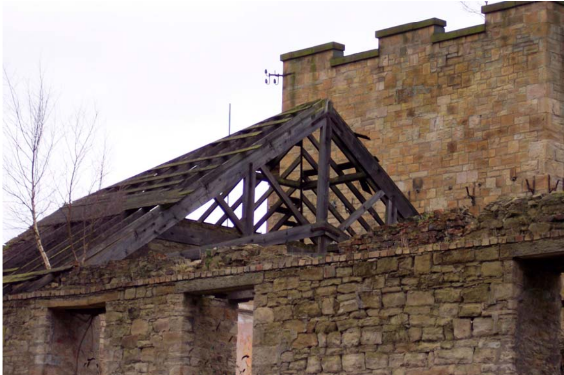
Plate 7: Detail of the roof-truss at the east end of the Annex roof showing surviving roof detail
