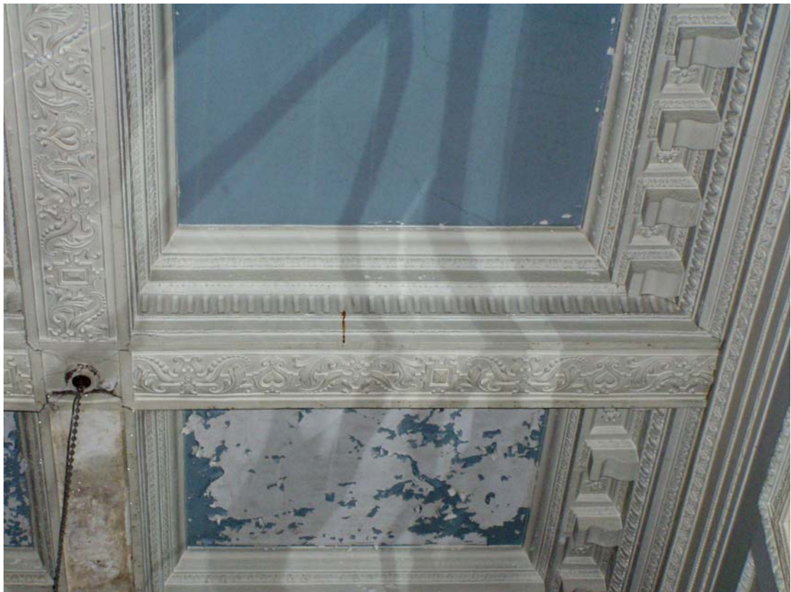
Plate 19: Detail of the ceiling compartments in the Best Dining Room (23)
