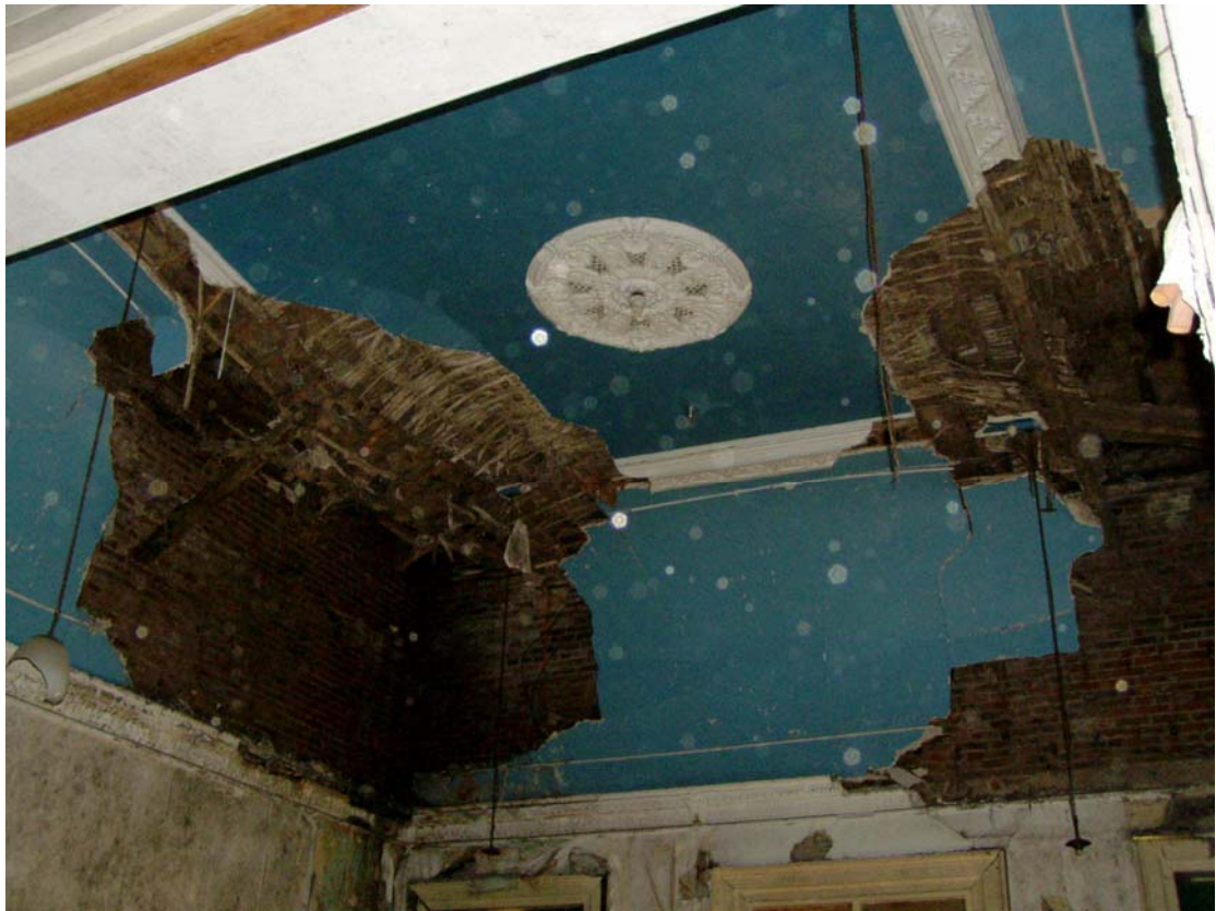
Plate 10: General view of the ceiling plasterwork in the Entrance Hall (29)
