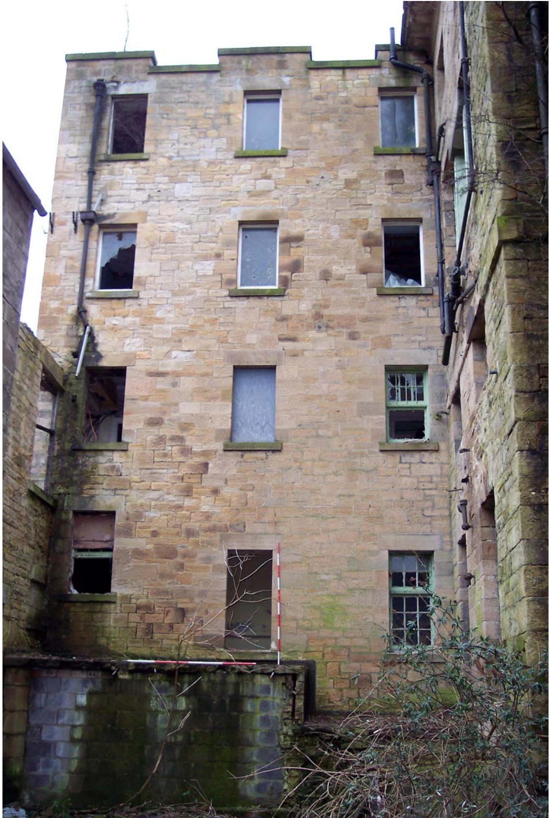
Plate 2: The west elevation of the toilet block
