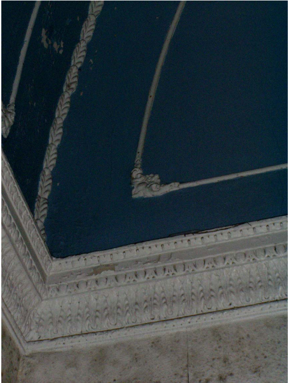
Plate 12: Detail of the cornice in the Entrance Hall (29)
