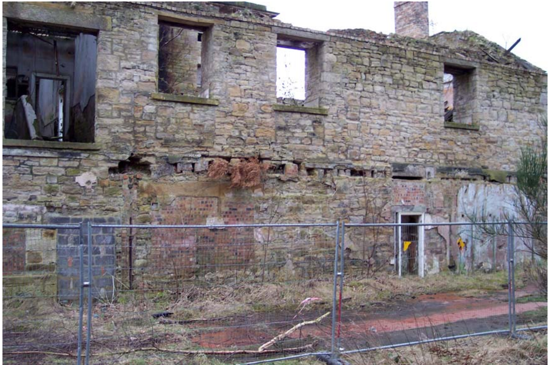
Plate 5: The north elevation of the Annex, east end
