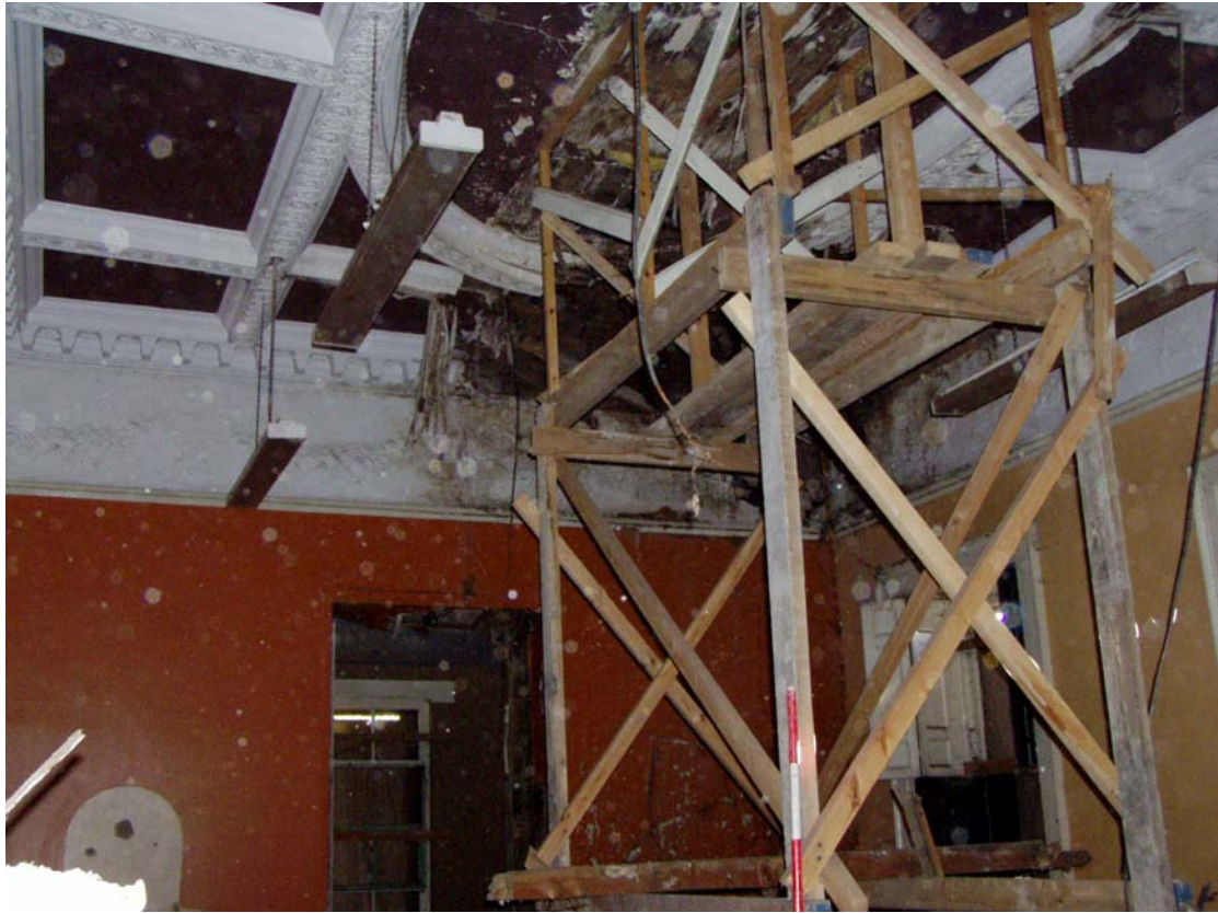
Plate 20: General view of the ceiling plasterwork in the Common Dining Room (28)
