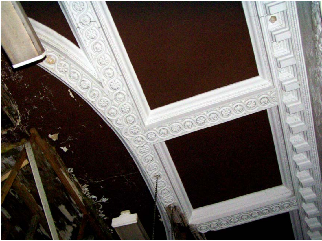
Plate 22: Detail of the ceiling compartments in the Common Dining Room (28)
