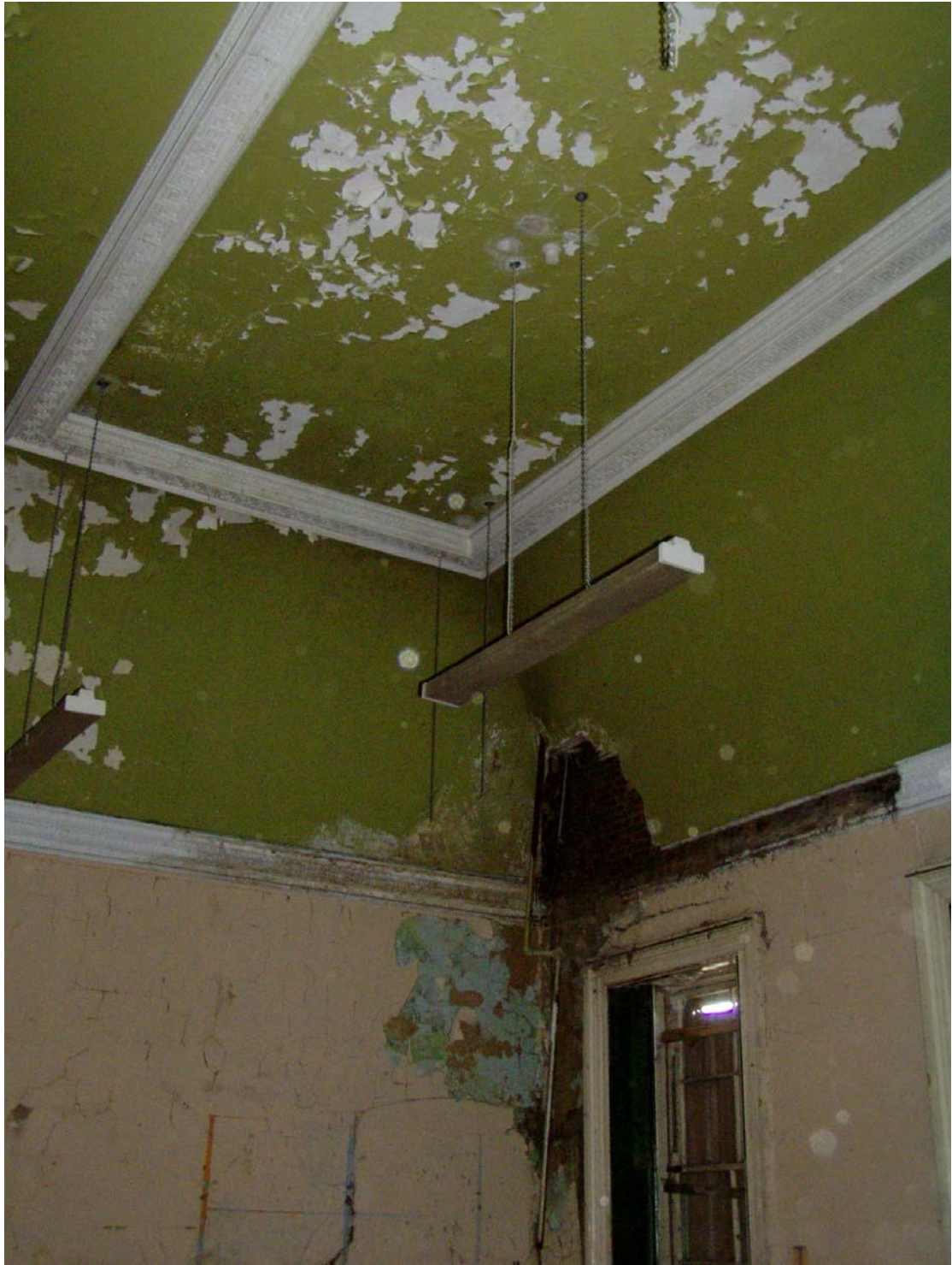
Plate 13: General view of the ceiling plasterwork in the Drawing Room (30)
