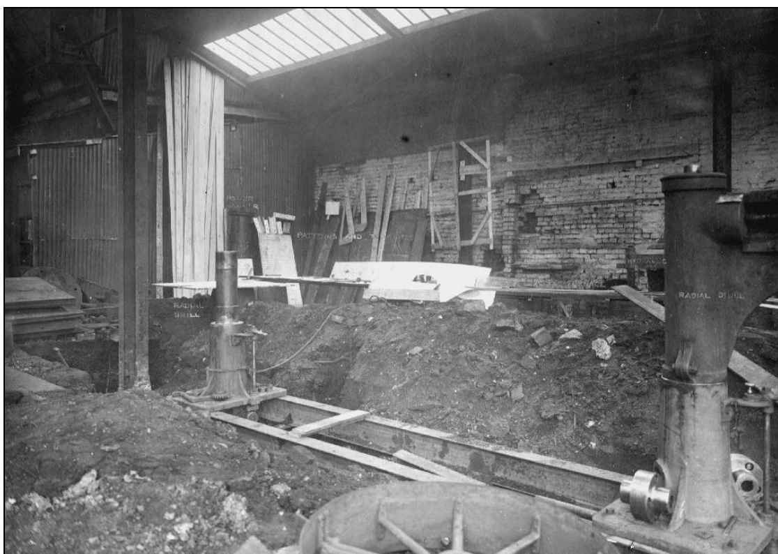
Plate 8: Baxendale's Iron Foundry, Kenyon Street, 1903
