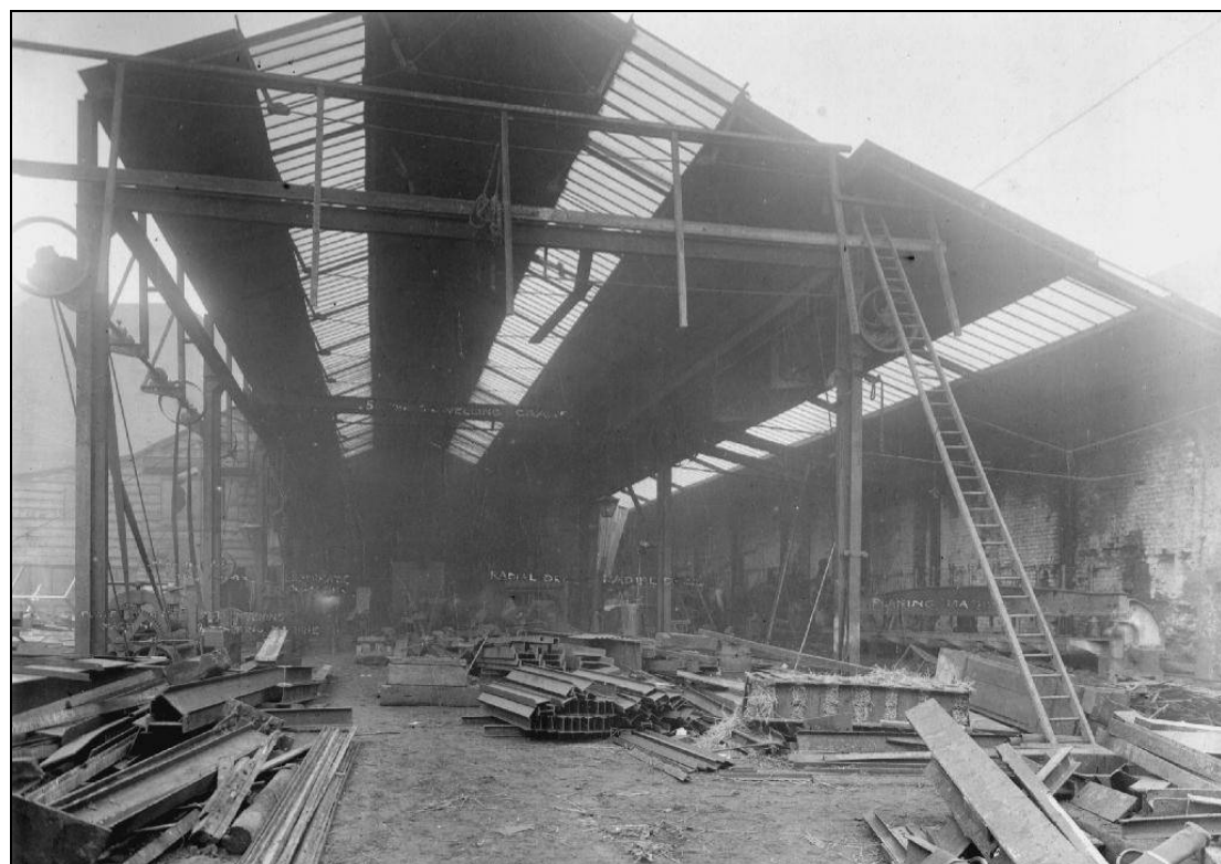
Plate 10: Baxendale's Iron Foundry, Kenyon Street, 1903
