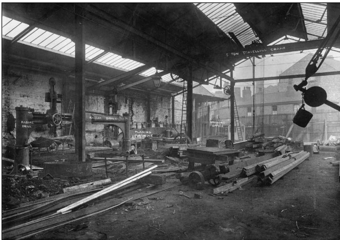
Plate 7: Baxendale's Iron Foundry, Kenyon Street, 1903
