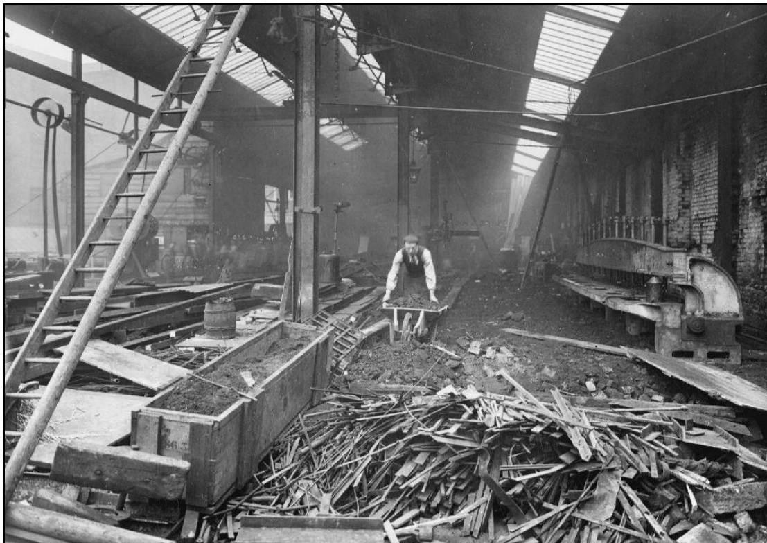
Plate 12: Baxendale's Iron Foundry, Kenyon Street, 1903
