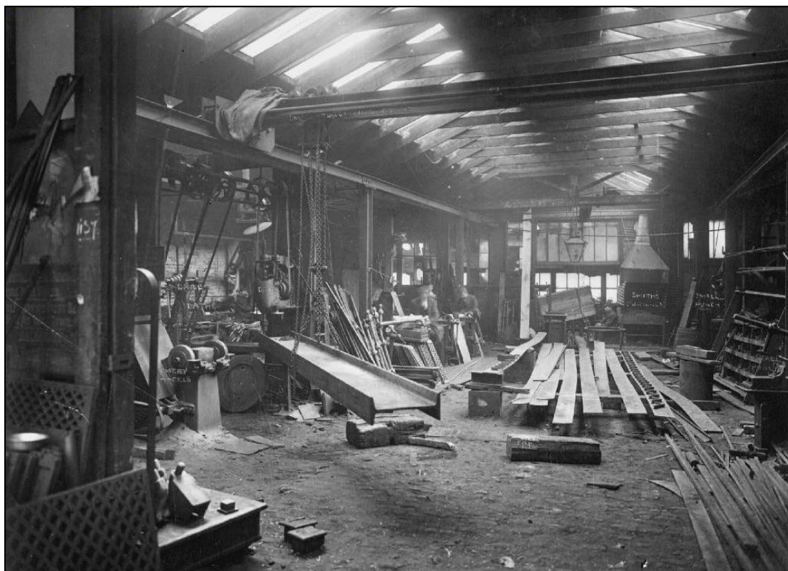
Plate 9: Baxendale's Iron Foundry, Kenyon Street, 1903
