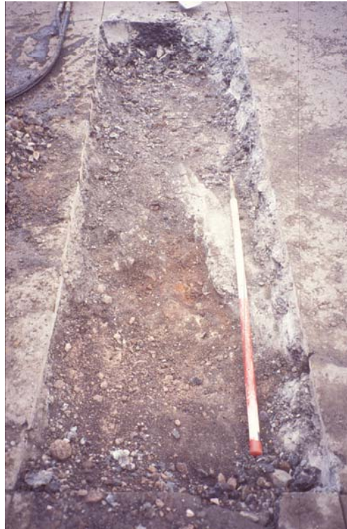
Plate 1: Brick-built culvert in SIP102, facing north-east
