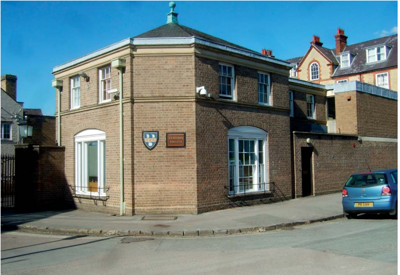
Plate 3 St Hilda's College Porters' Lodge (facing north west)
