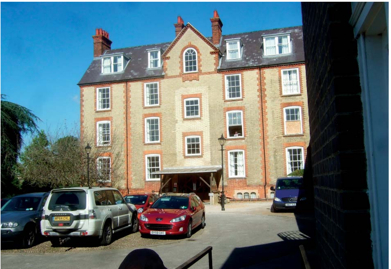
Plate 4 The early 20th century south wing of St Hilda's north building (facing north)
