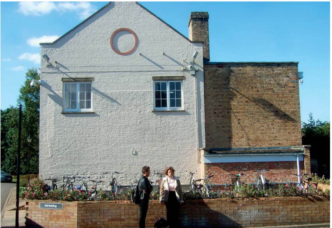
Plate 2 The east elevation of Milham Ford Building (facing west)
