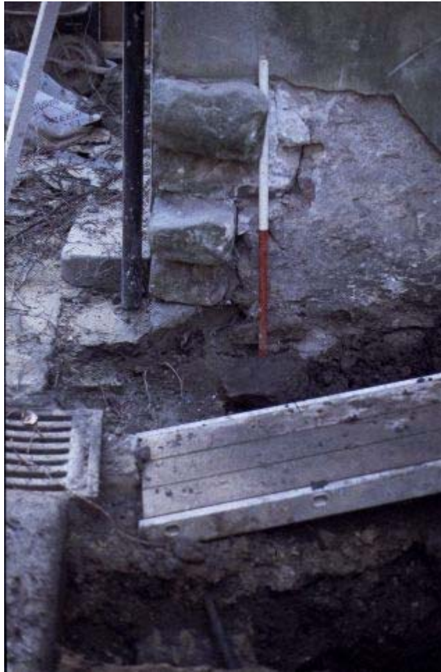
Plate 3: Wall scar on main building and demolished wall in trench
