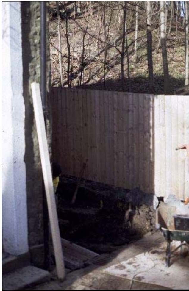
Plate 1: General View of excavated area
