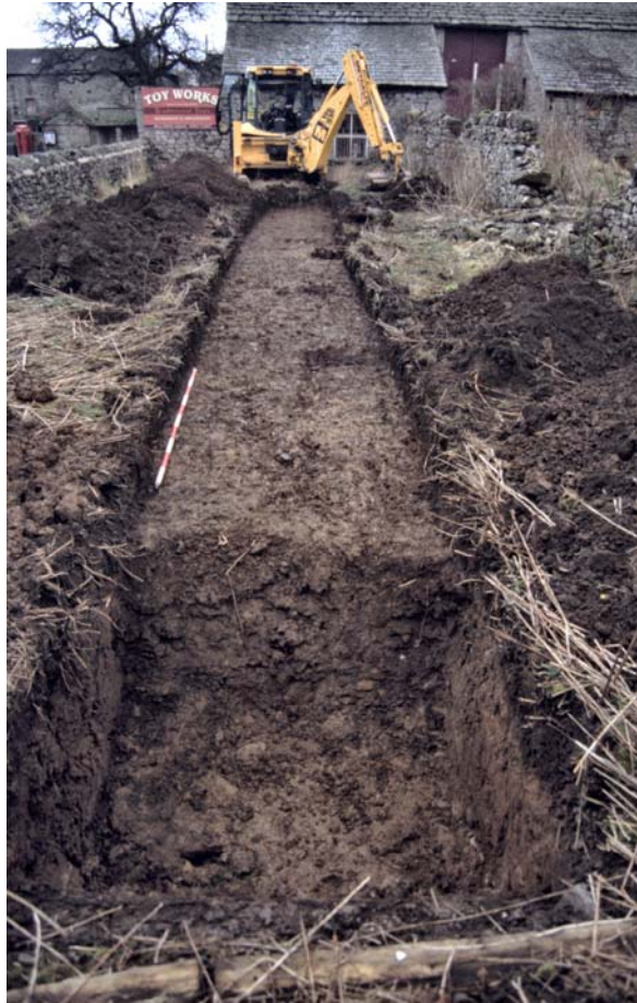
Plate 7: pre-excavation view of Trench 1, viewed from the north
