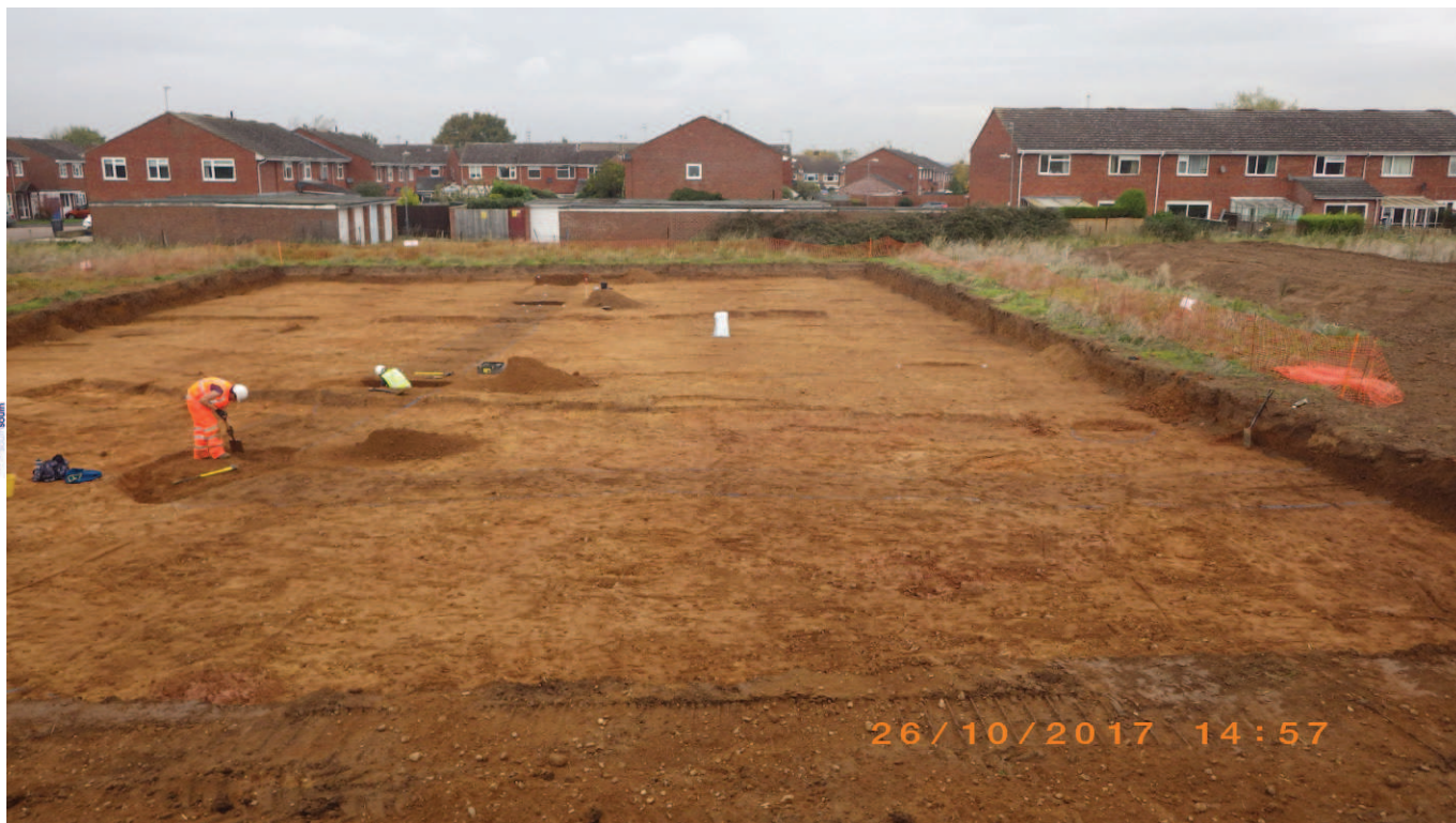
Plate 1: The site during excavation, looking north
