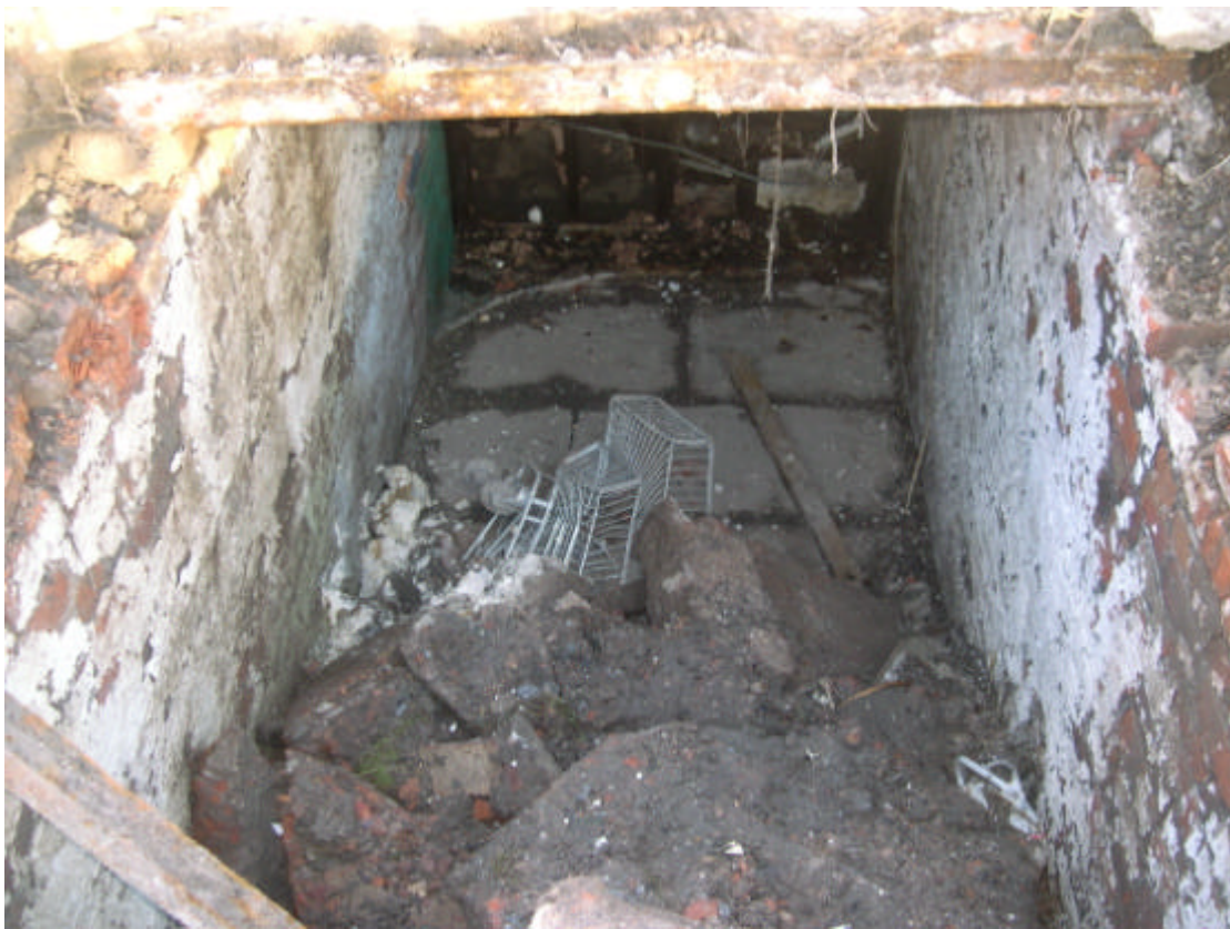
Plate 12: Cellar exposed within Trench 4, Area G3
