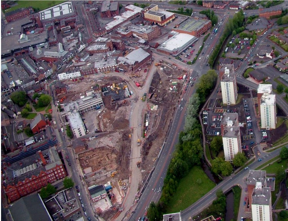
Plate 1: Aerial view of the development area
