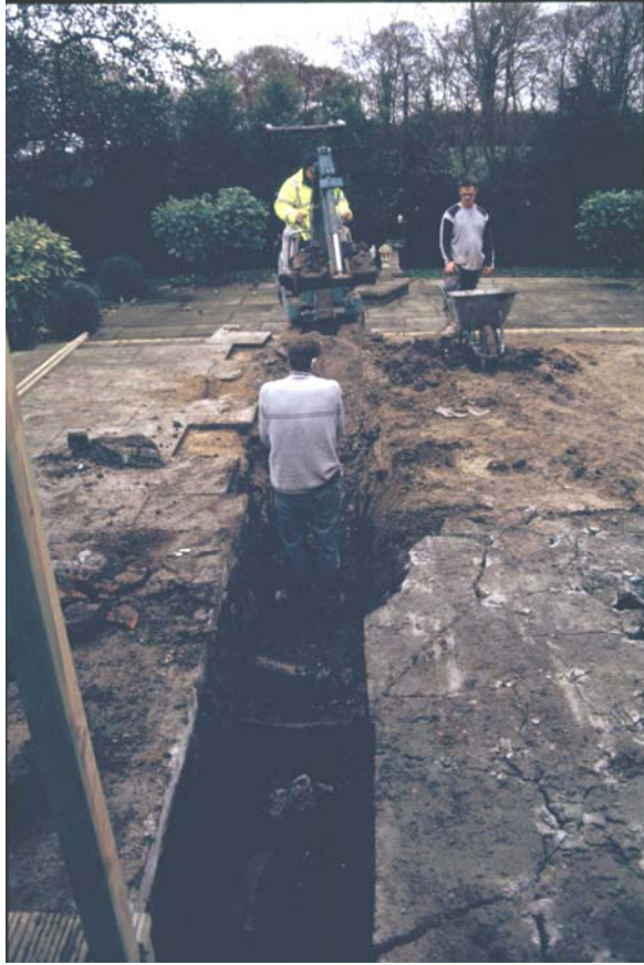
Plate 1: Excavation of the Foundation Trench
