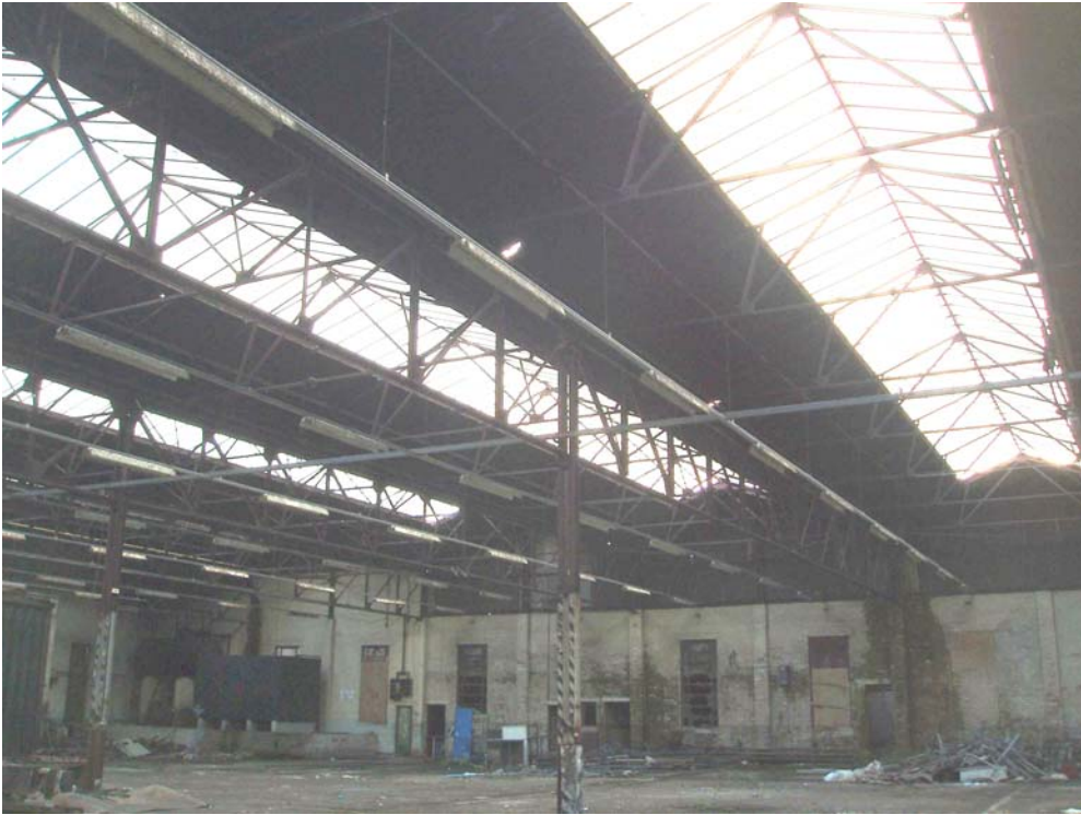
Plate 20: Roof of the depot
