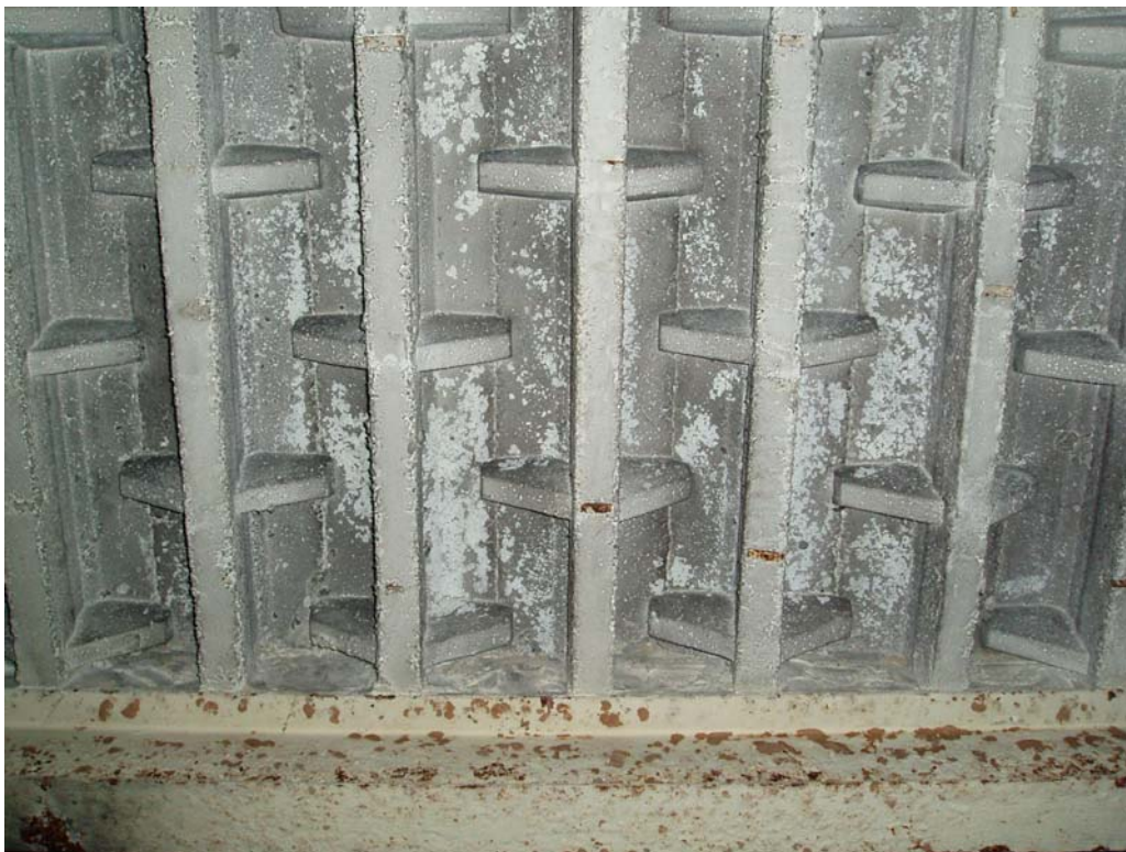
Plate 23: Typical pre-cast concrete ceiling in rooms along west end of the depot
