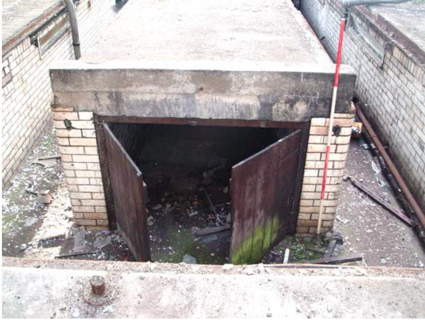
Plate 14: Storage bay in an inspection pit
