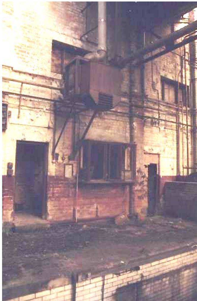
Plate 15: Oriel-style window in the east elevation of the depot
