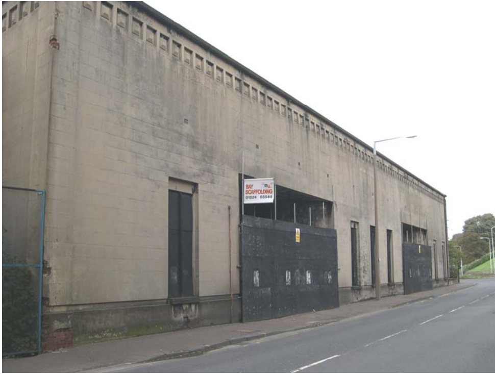
Plate 9: Rear (south) elevation
