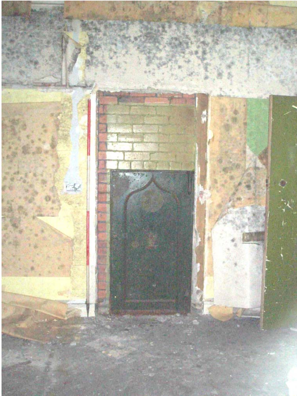
Plate 13: Iron door, probably for a safe, built into a blocked doorway in the west wall of the bar area
