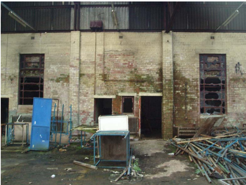
Plate 21: Inserted doorways and window in the west elevation
