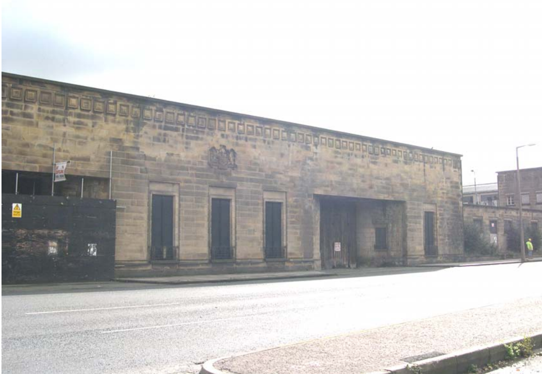
Plate 5: West end of the front (north) elevation
