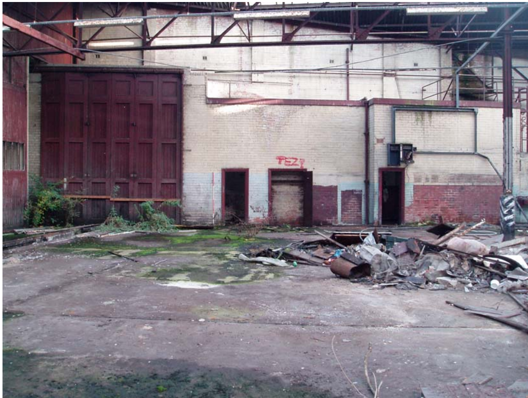
Plate 19: Row of small rooms attached to the south elevation of the depot
