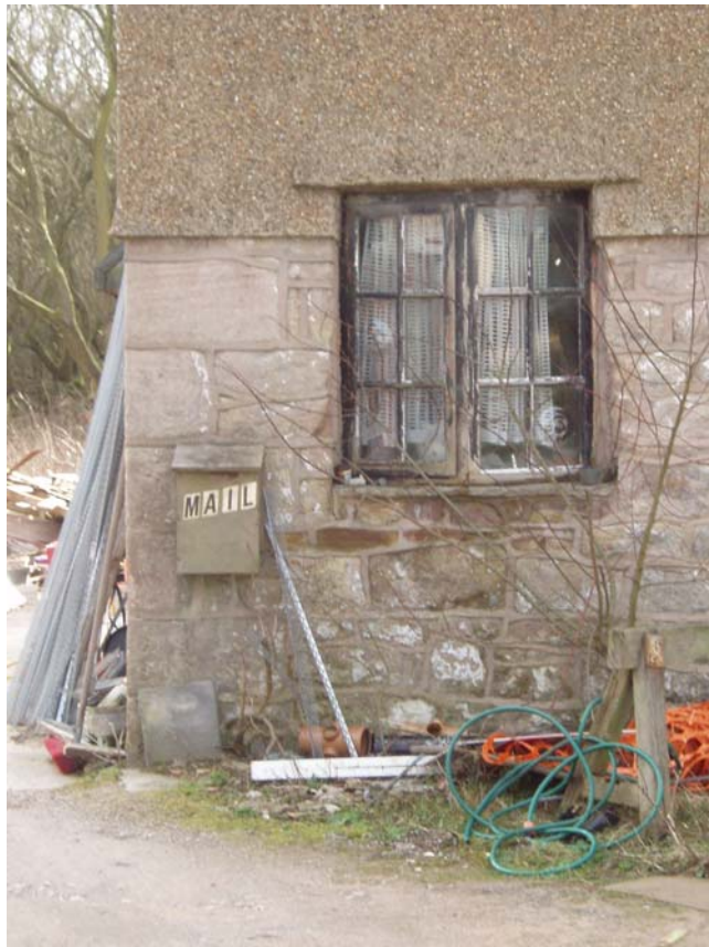
Plate 6: Window in north-west gable
