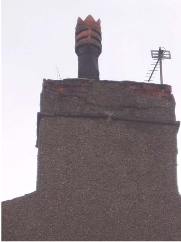
Plate 7: Chimney on north-west gable
