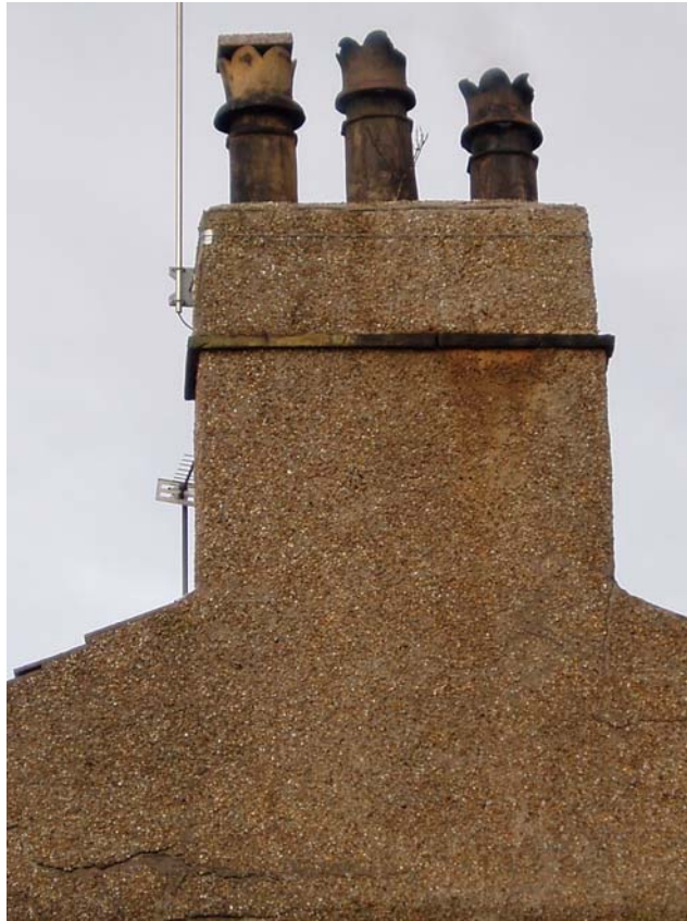
Plate 13: Chimney on south-east gable
