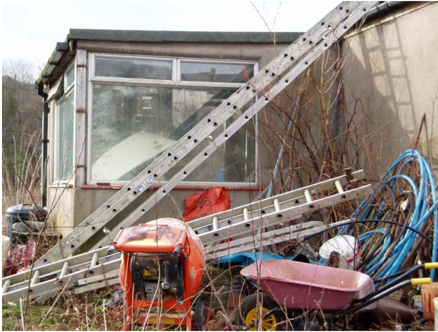
Plate 15: Extension on south-east elevation (south-west side)
