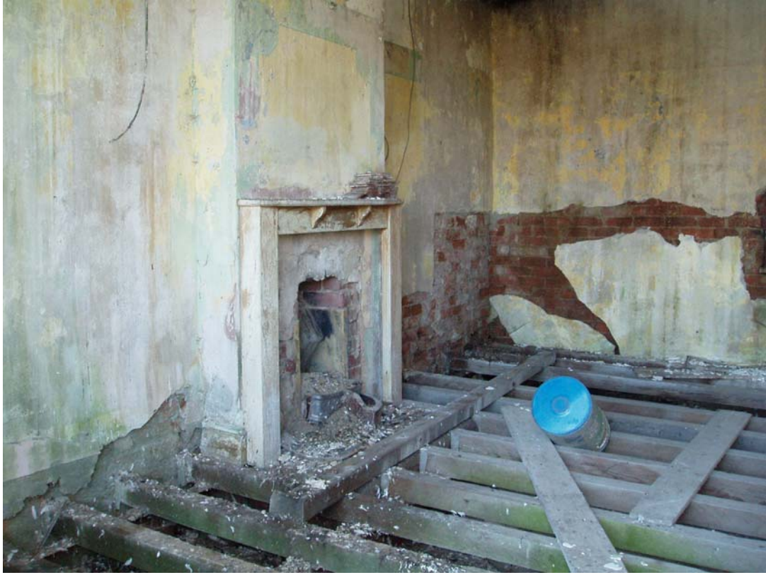
Plate 21: Fireplace in Room 2
