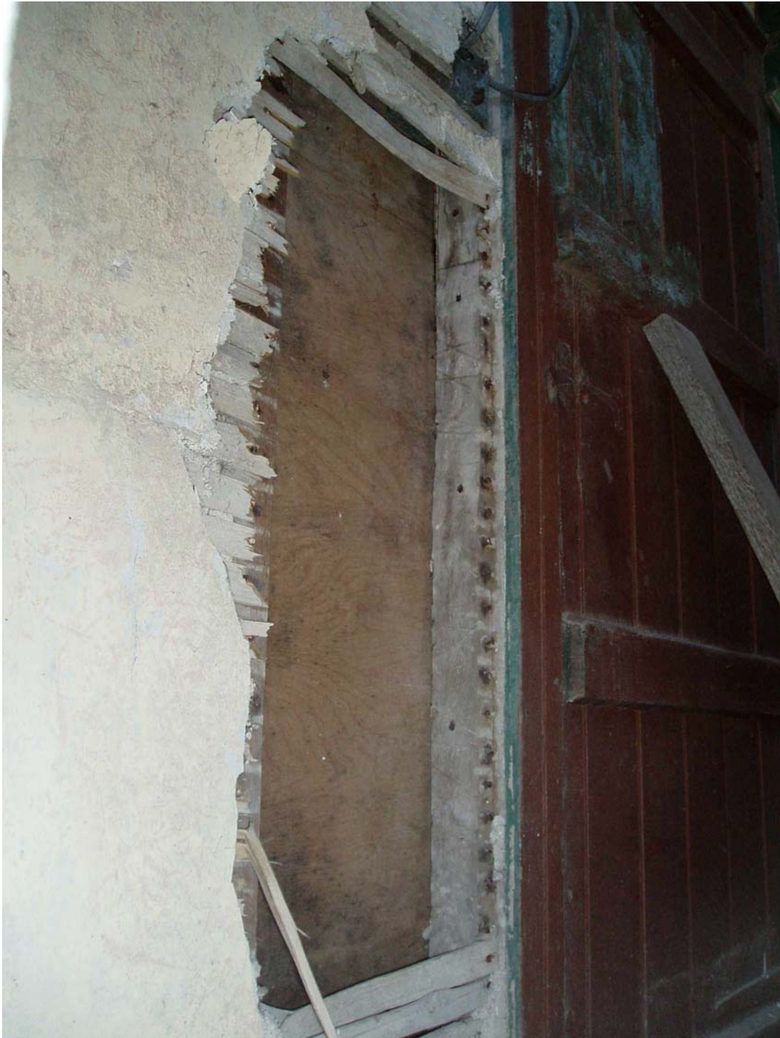
Plate 23: Baltic timber marks in the stud partition wall of Room 1A
