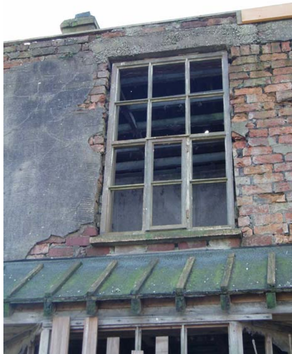
Plate 14: Inserted easternmost first floor window in front (north) elevation
