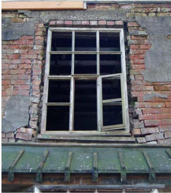
Plate 15: Inserted westernmost first floor window in front (north) elevation
