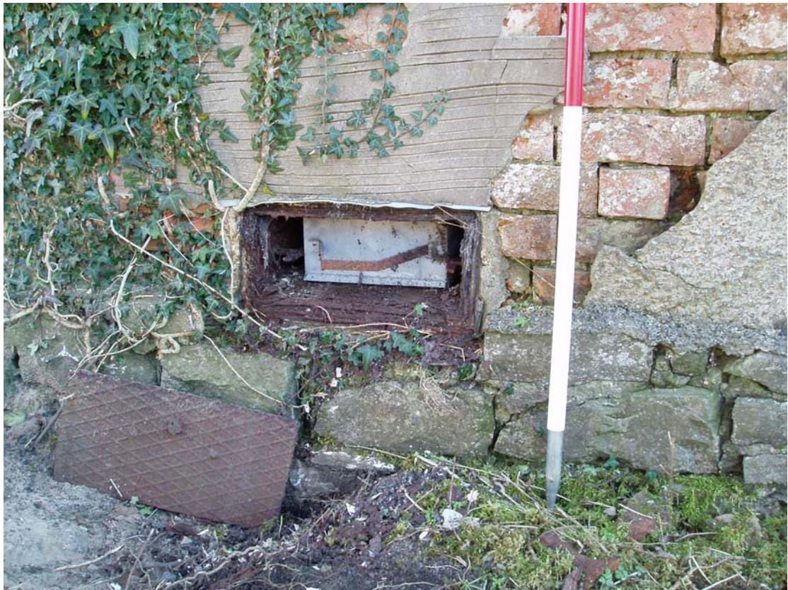
Plate 22: Ash chute and pan in east elevation of main building
