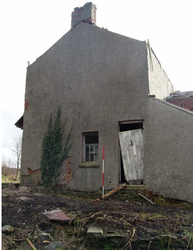
Plate 17: West external elevation
