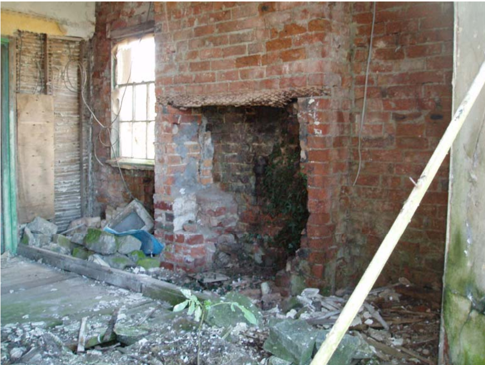
Plate 20: Fireplace in Room 1
