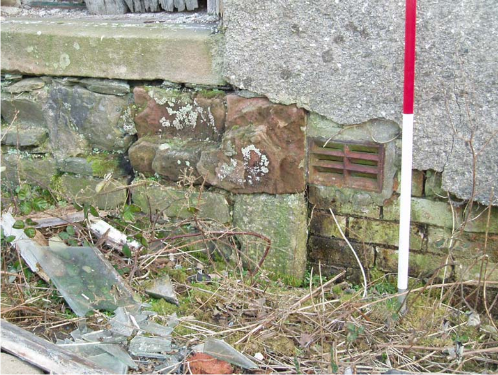
Plate 19: Detail of plinth at south-east corner of main building
