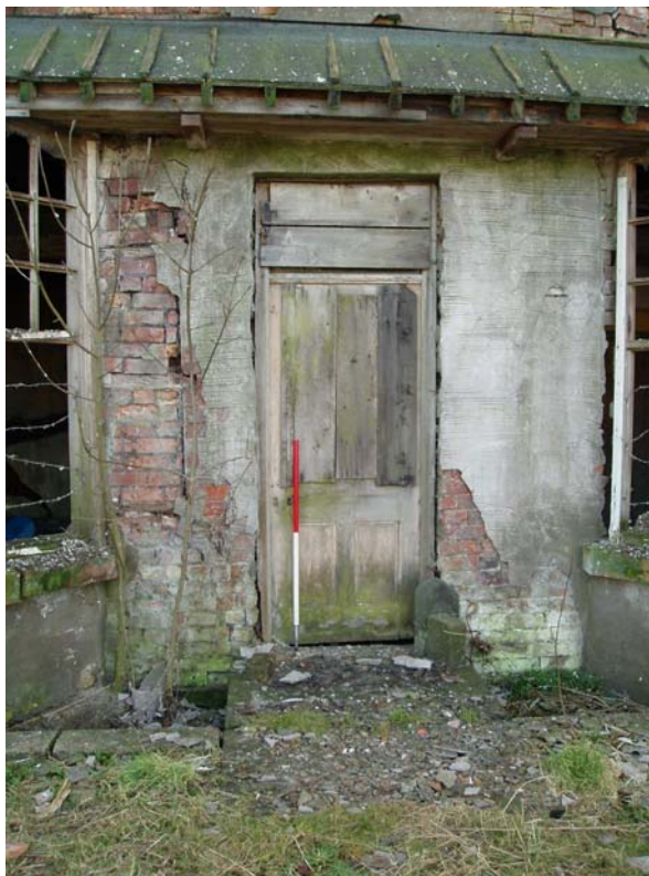
Plate 16: Altered or inserted front doorway in north elevation
