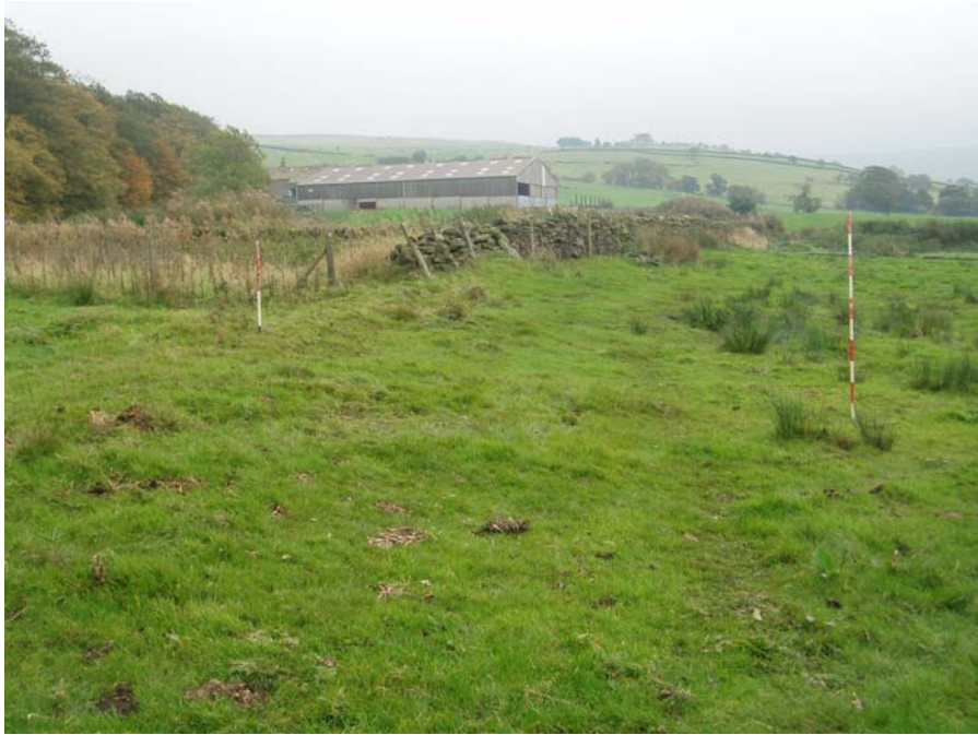
Plate 27: Site 119 , collapsed boundary wall, Laithe Farm
