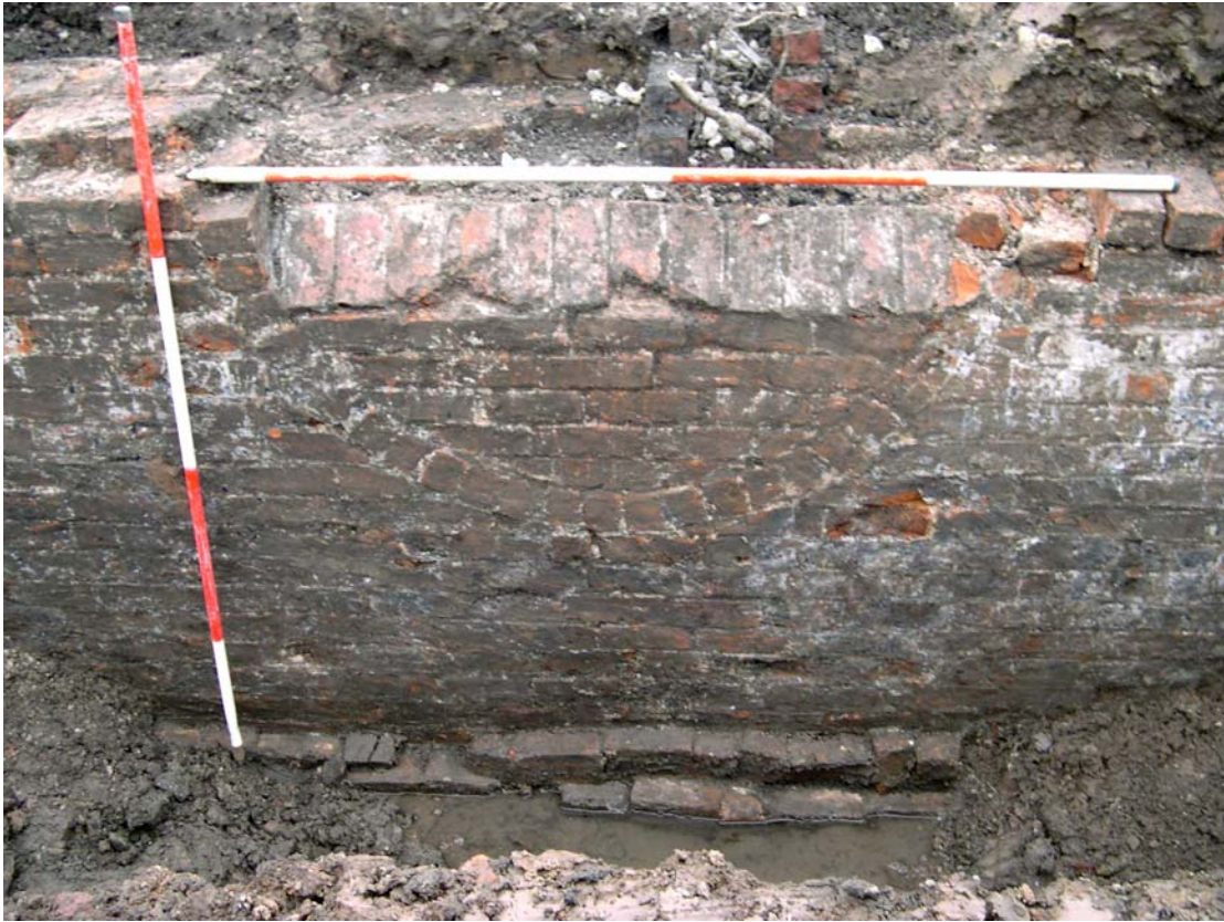
Plate 3: The central relieving arch within wall 205 , Trench 2, with sloping bricks denoting use as a cellar light
