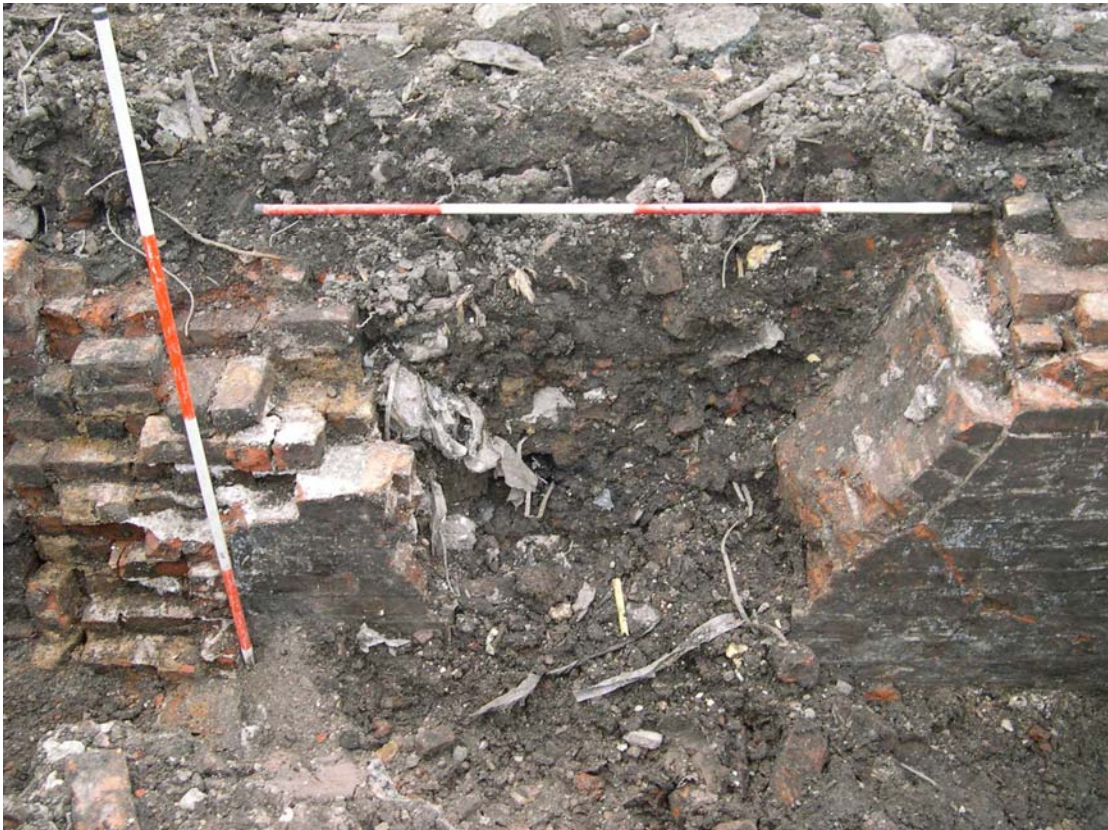
Plate 4: The north-western relieving arch within wall 205 , damaged subsequently by the insertion of manhole 208
