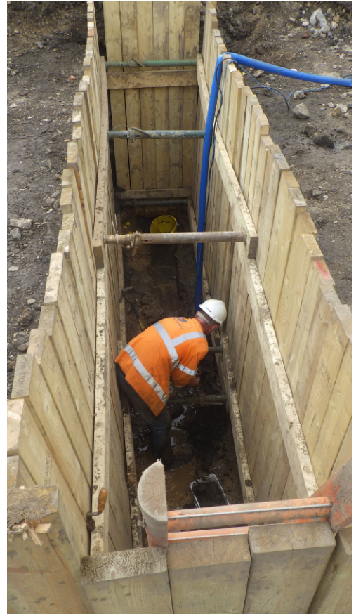
Plate 5: Excavating pits in Trench 2
